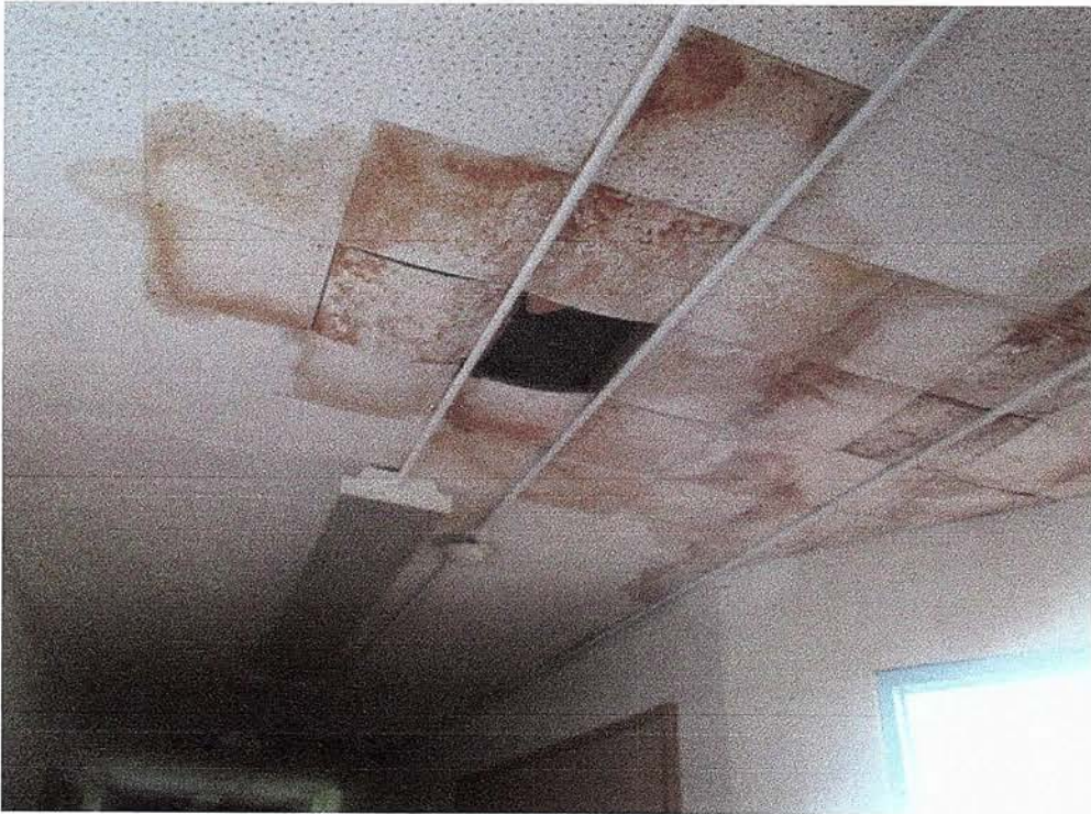
WATER DAMAGE THROUGH ROOF
