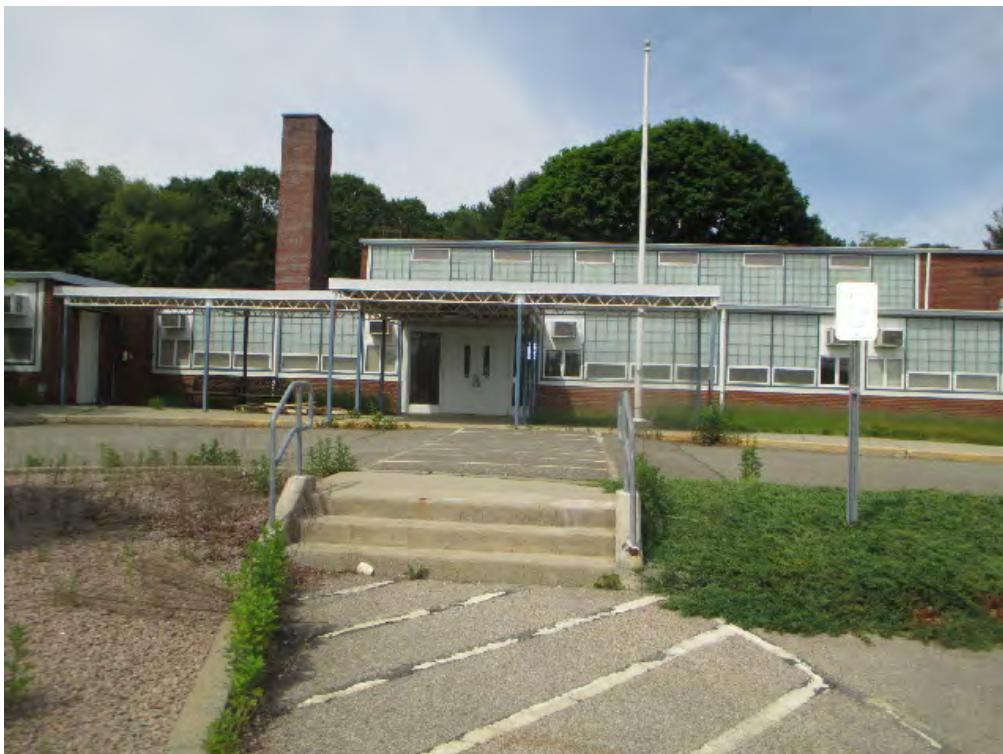
BUILDING NO. 1 - FRONT VIEW
