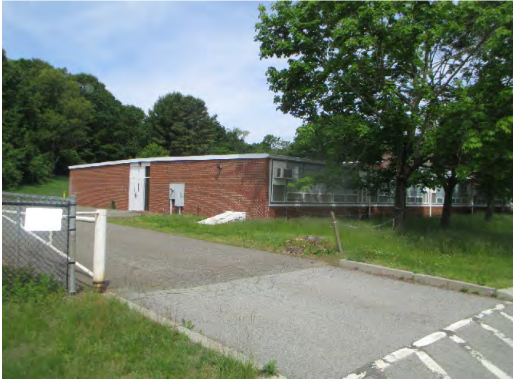
BUILDING NO. 1 - SIDE VIEW
