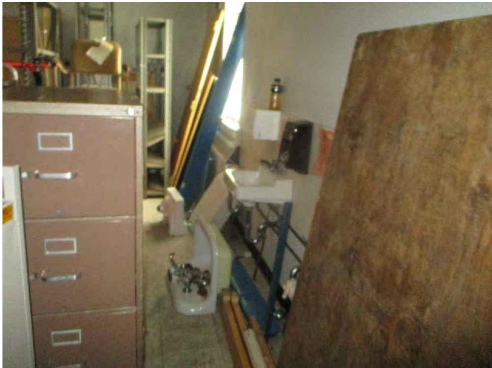
BUILDING NO. 3 - INTERIOR VIEW / BATHROOM
