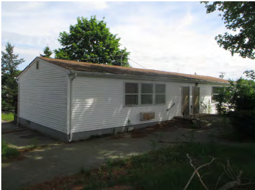
BUILDING NO. 2 - FRONT VIEW
