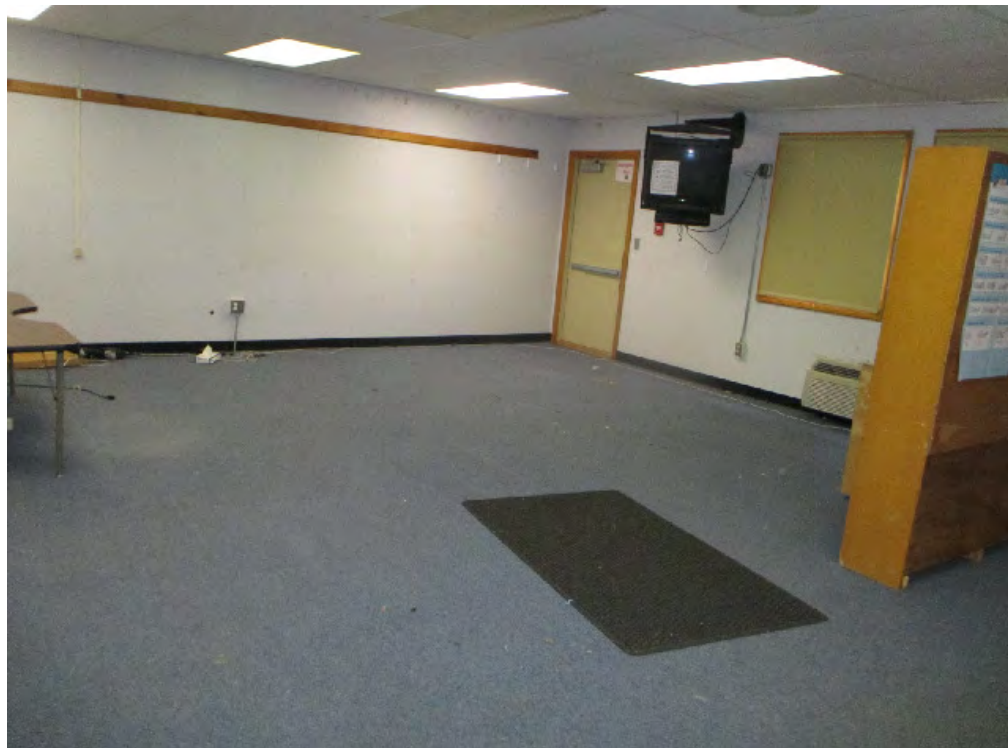
BUILDING NO. 2 - INTERIOR VIEW
