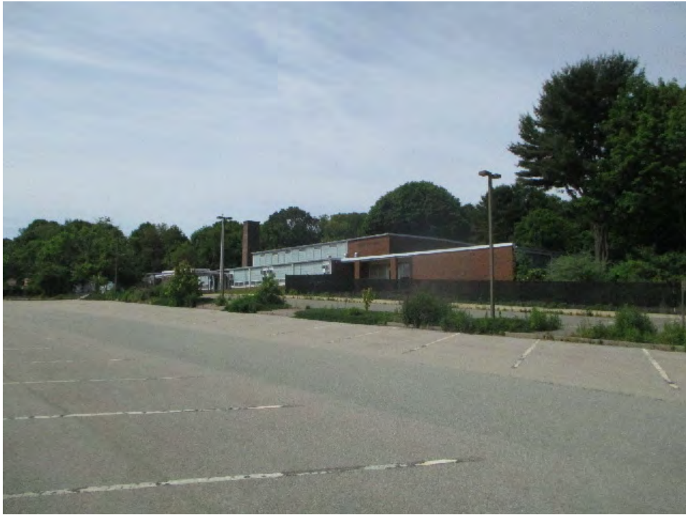
BUILDING NO. 1 - FRONT VIEW
