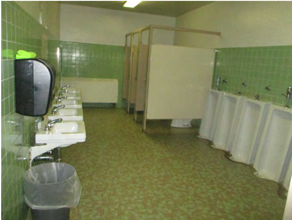
BUILDING NO. 1 - INTERIOR VIEW / BATHROOM
