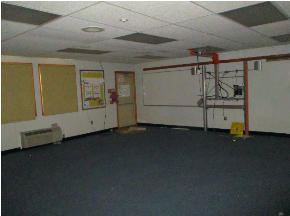
BUILDING NO. 2 - INTERIOR VIEW
