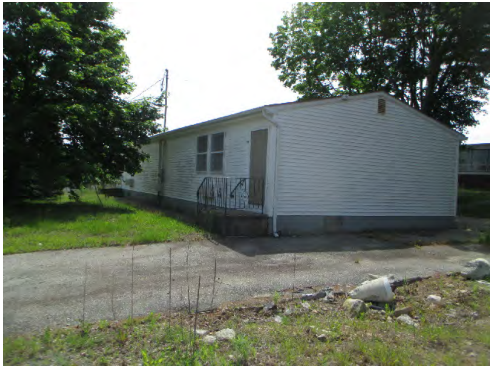
BUILDING NO. 2 - FRONT VIEW
