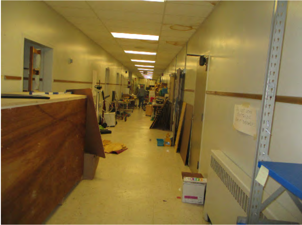
BUILDING NO. 1 - INTERIOR VIEW / HALLWAY
