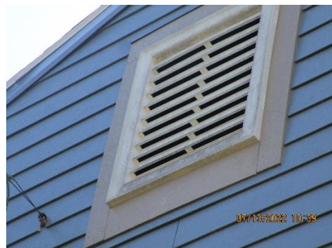
Images 18, 19: Attic ventilation is limited to gable vents at the gable end of each building "block", and shingle-over ridge vents.
