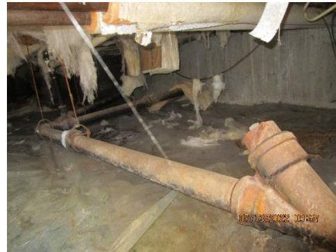
Images 12, 13: Crawlspaces with dislodged insulation, and unsealed poly vapor barrier
