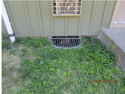
Images 5, 6: Basement window well and crawlspace vent level with existing grade and subject to water infiltration.
