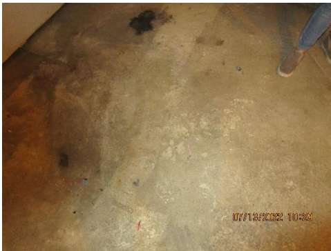
Images 16, 17: Surface spalling on concrete basement slab; staining and potential mold growth at base of concrete foundation wall.
