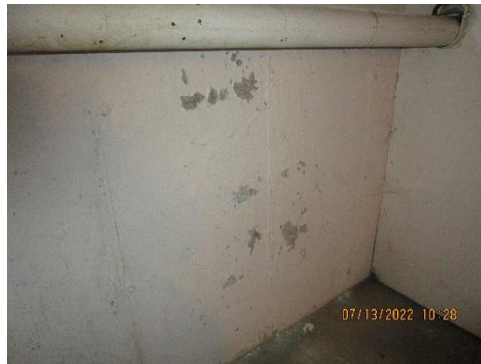
Images 14, 15: Typical basement space with framed partition to right of image; spalling coating indicating presence of moisture in concrete wall.
