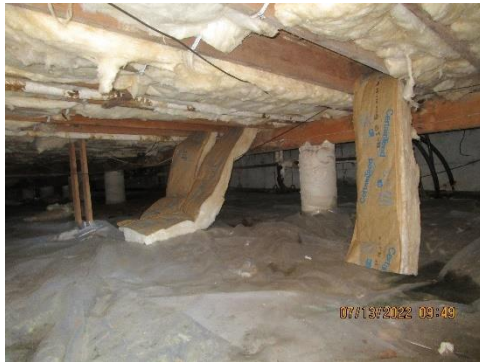
Images 12, 13: Crawlspaces with dislodged insulation, and unsealed poly vapor barrier
