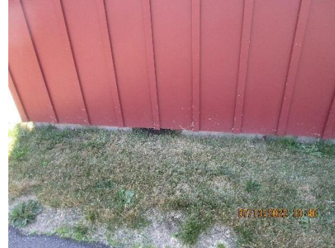
Images 5, 6: Basement window well and crawlspace vent level with existing grade and subject to water infiltration.
