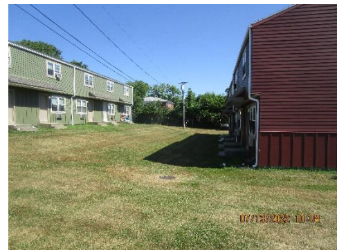
Images 7, 8: Grades slope to the northeast generally. Drainage swales exist between buildings but are marginal in some cases. Positive drainage away from foundations should ideally extend for 10' minimum away from each building.
