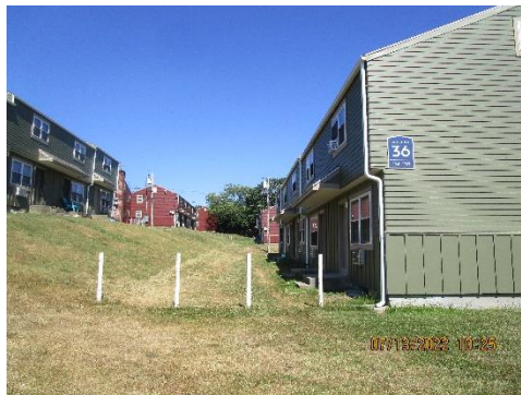
Images 7, 8: Grades slope to the northeast generally. Drainage swales exist between buildings but are marginal in some cases. Positive drainage away from foundations should ideally extend for 10' minimum away from each building.
