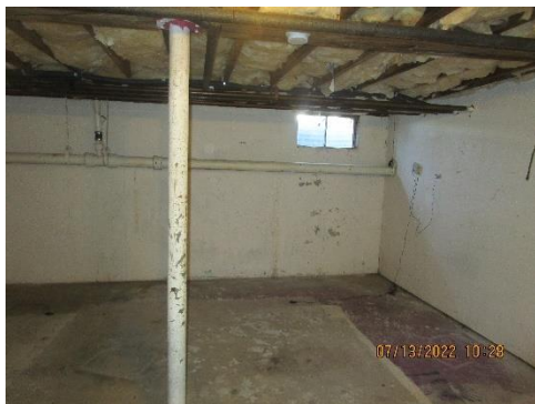
Images 14, 15: Typical basement space with framed partition to right of image; spalling coating indicating presence of moisture in concrete wall.
