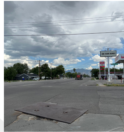
Missing Curb and Gutter
