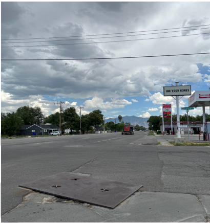
Missing Curb and Gutter
