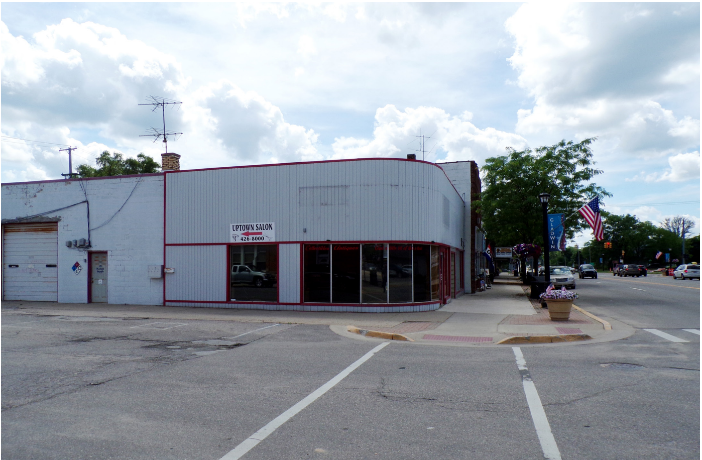
Vacant storefronts detract from the downtown's commercial environment.
