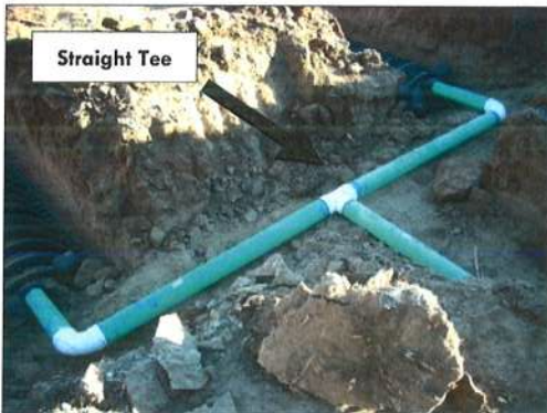
Straight tees (left) and four-way tees are not recommended because they will not evenly divide effluent entering the leach field.
