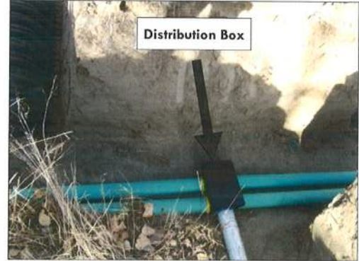
Preferred components for even distribution of effluent: Flow Divider Tee (left) and Distribution Box (right)
