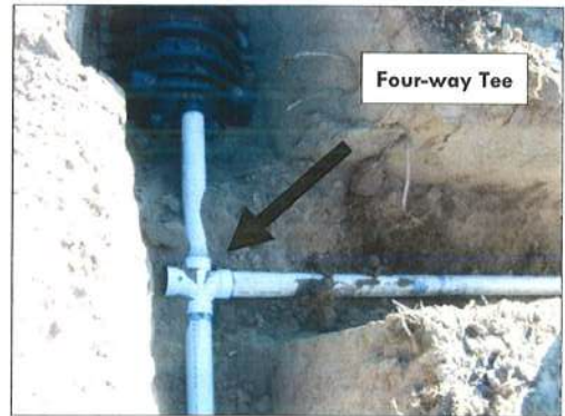
Straight tees (left) and four-way tees are not recommended because they will not evenly divide effluent entering the leach field.
