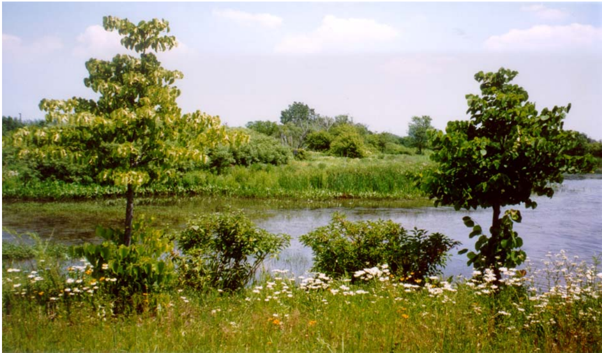
Photo 1 – Wet bottom basin with broad emergent shelf and wet-mesic prairie slopes with clusters of woody vegetation. Note the irregular shape of the basin. (early summer)
