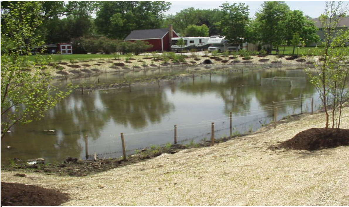
Photo 13 – Recently installed low-profile prairie and ornamental hybrid combination wetland bottom basin
