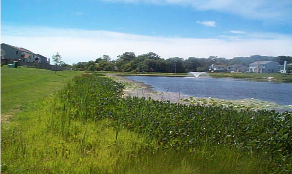
Photo 3 – Wet bottom basin with water quality aeration system, a broad emergent zone, and a deepwater emergent zone. Note that a portion of the shallow basin slope is vegetated with traditional turfgrass (summer) [Photo courtesy of EnCAP, Inc.]
