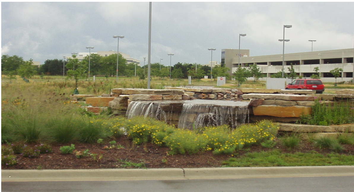
Photo 10 – Water quality enhancement cascade with ornamental landscape as part of stormwater management system
