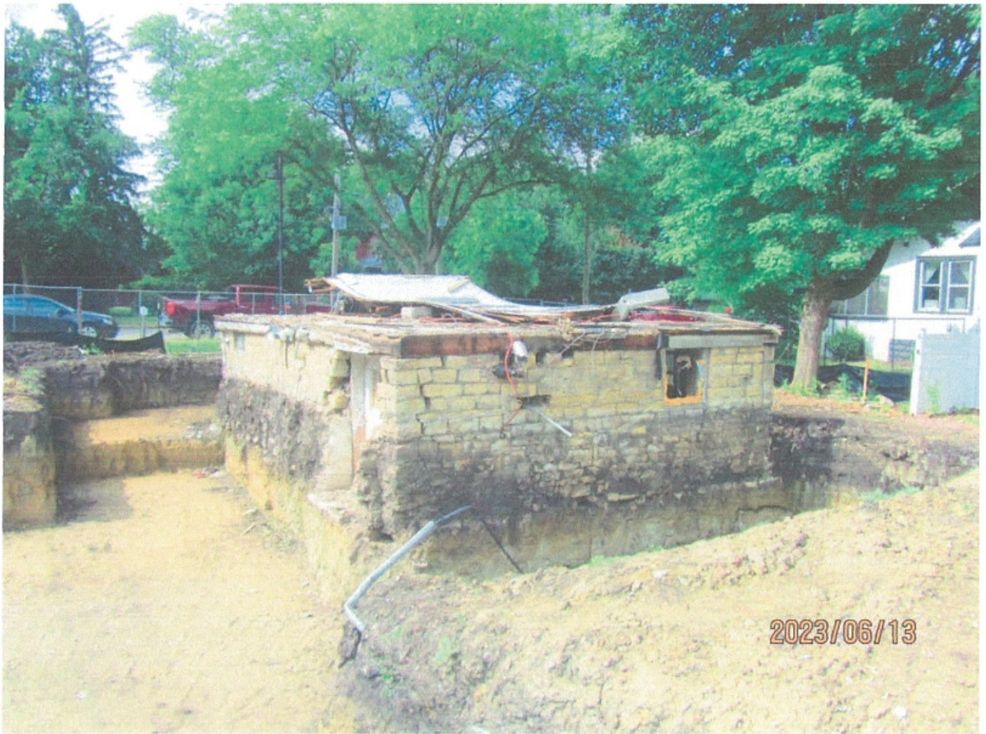
Large Cracks, Voids, and Displacement in Foundation Wall
