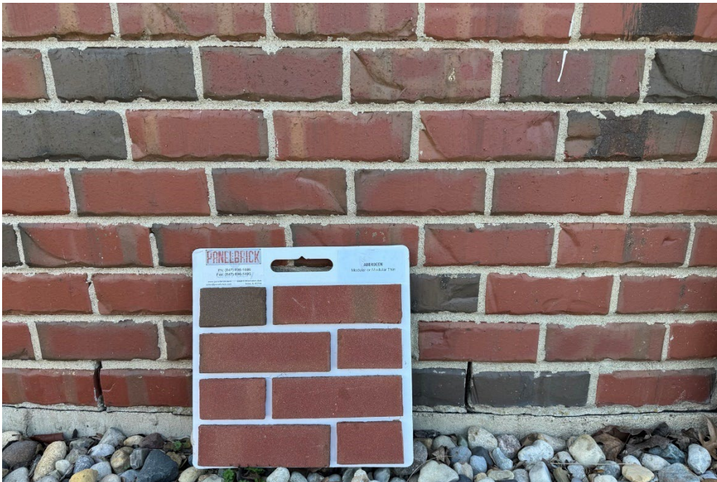
Figure 8: Existing brick façade at 10217 W. Lincoln Highway (same brick material among the other office buildings in Brookside Commons) compared to proposed Panelbrick brand thin brick veneer product in “Aberdeen” style (proposed to replace existing EIFS material on entrance tower).
