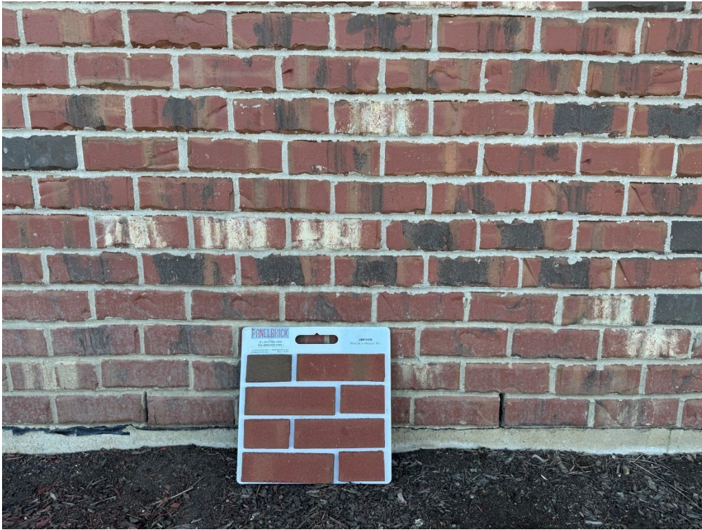
Figure 7: Existing brick façade at 10211 W. Lincoln Highway compared to proposed Panelbrick brand thin brick veneer product in “Aberdeen” style (proposed to replace existing EIFS material on entrance tower).
