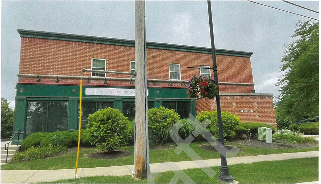
View of side of building (east):
