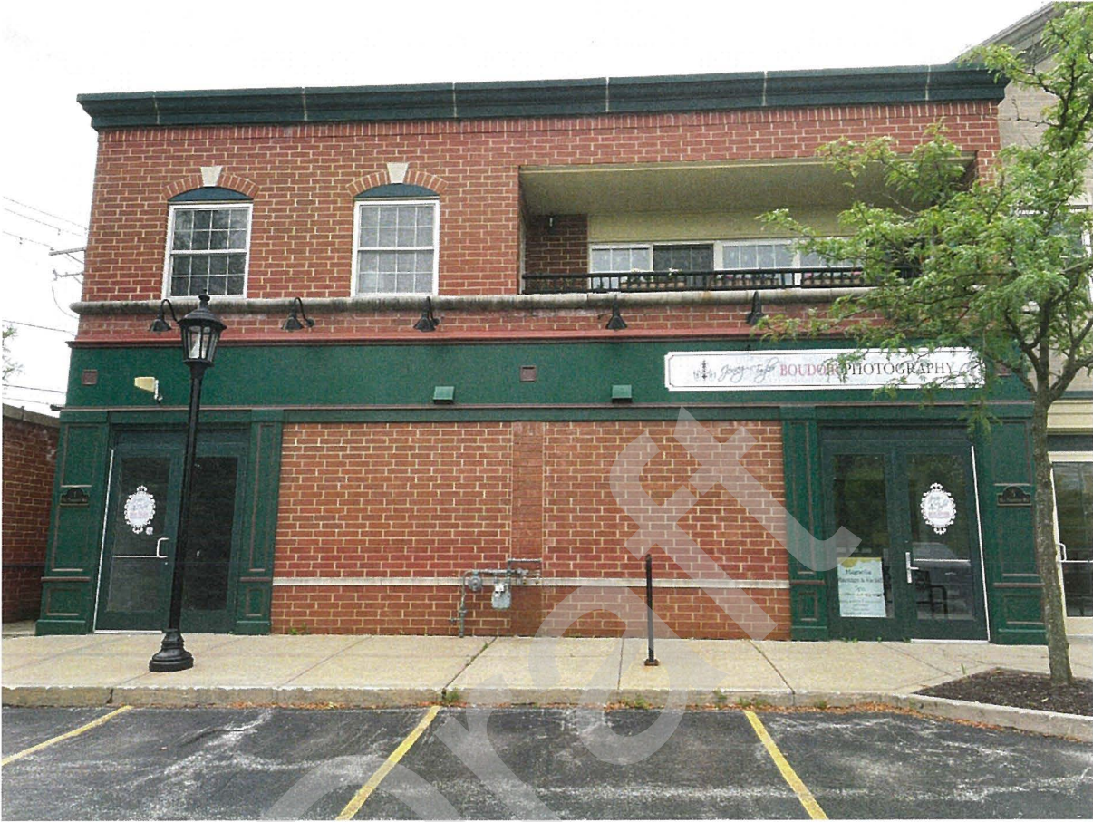
View of back of building (north):
