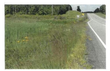
conditions suggest ditch problems: road appearance, ditch erosion or soil instability, and water flow.
