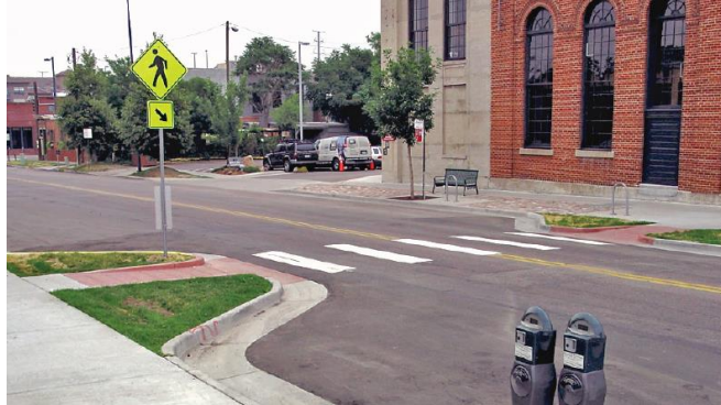
Curb Extension (“Bump-out”)
