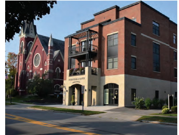
A mix of uses is important to a vital Main Street.
