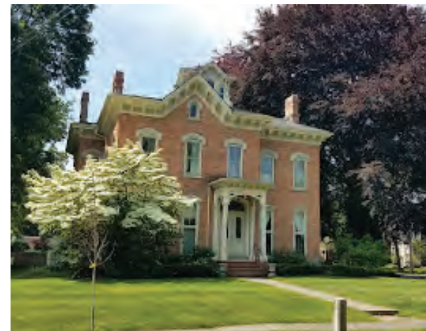
Diverse housing choices such as this multi-unit building can fit into historic neighborhoods.
