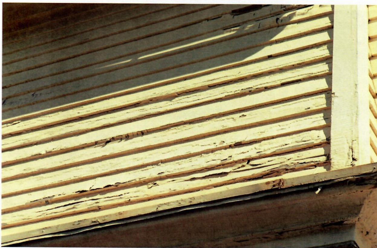
WOOD SIDING & TRIM NEEDS PAINTING EXCEPT AT TOWER - SOUTH SIDE IN WORST CONDITION
