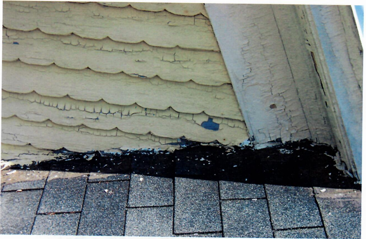
WOOD SIDING SHOULD BE CUT BACK & METAL STEP FLASHING PROVIDED WITH COUNTER FLASHING
