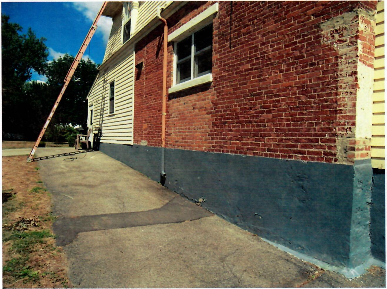
LOWER BLOCK & MASONRY SHOULD BE PAINTED & PATCHED
