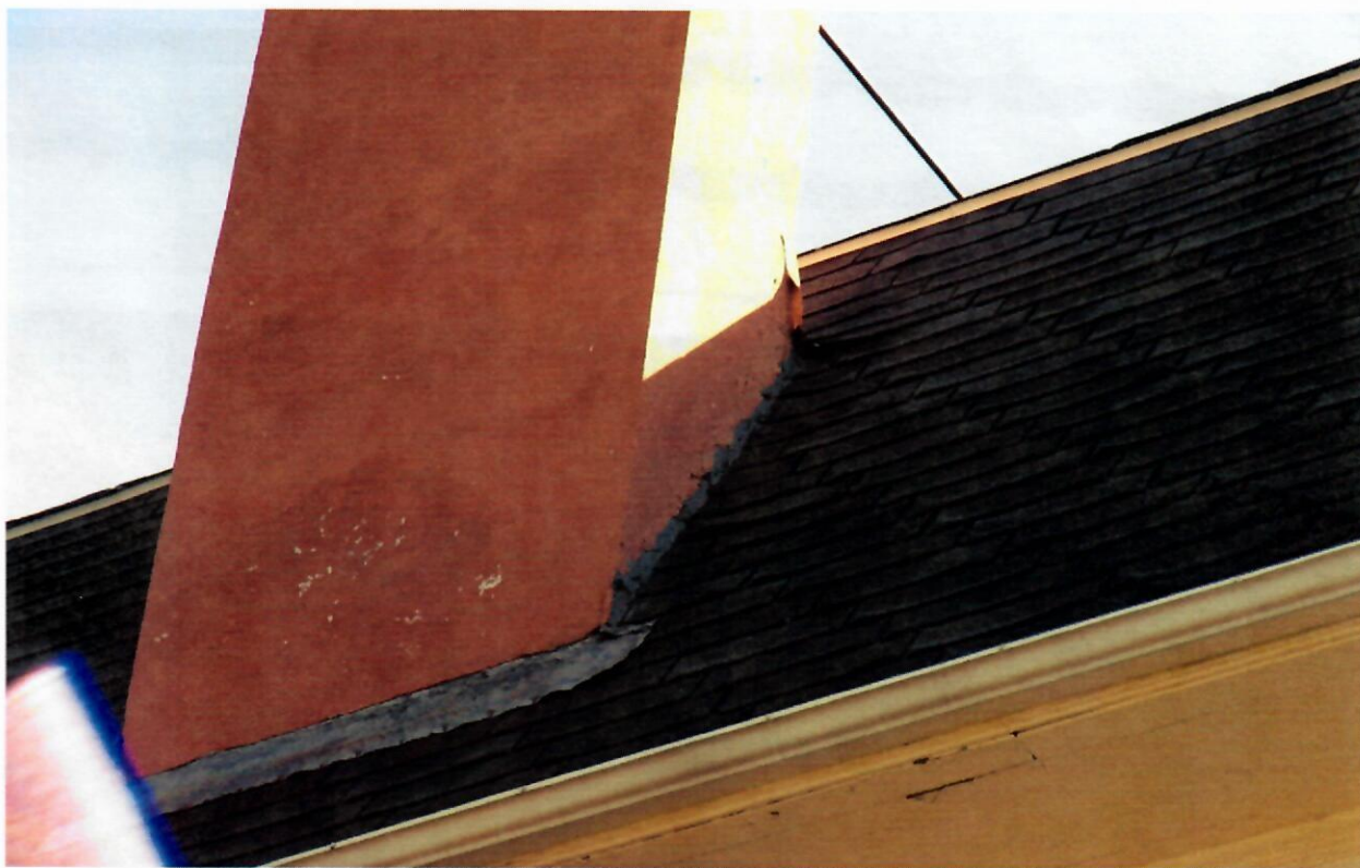
CHIMNEY NEEDS SADDLE & NEW FLASHING
