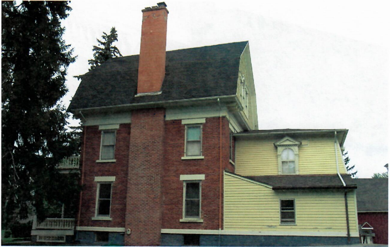
UPPER PORTION NEEDS PAINT REMOVED & REPAIR/REPOINTING
