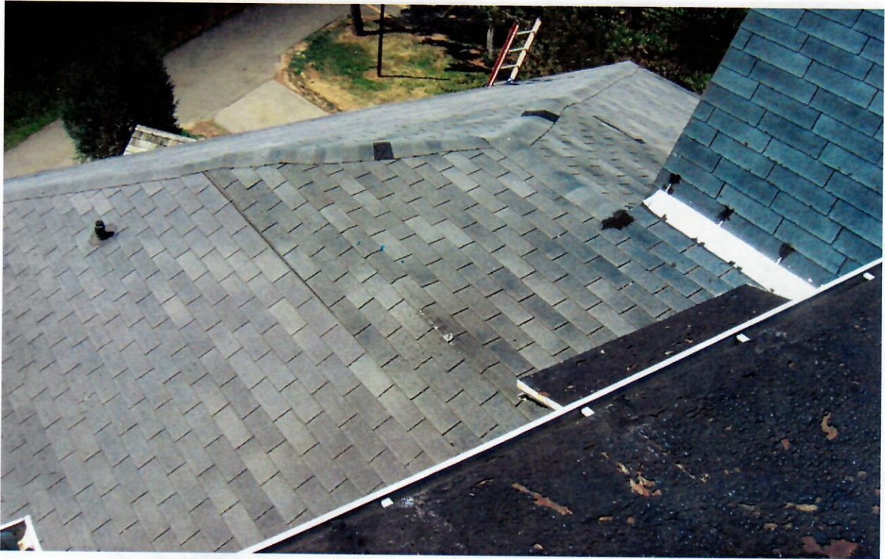
MISSING SHINGLES & CONFIGURATION OF ROOFS LEADS TO PREMATURE AGING
