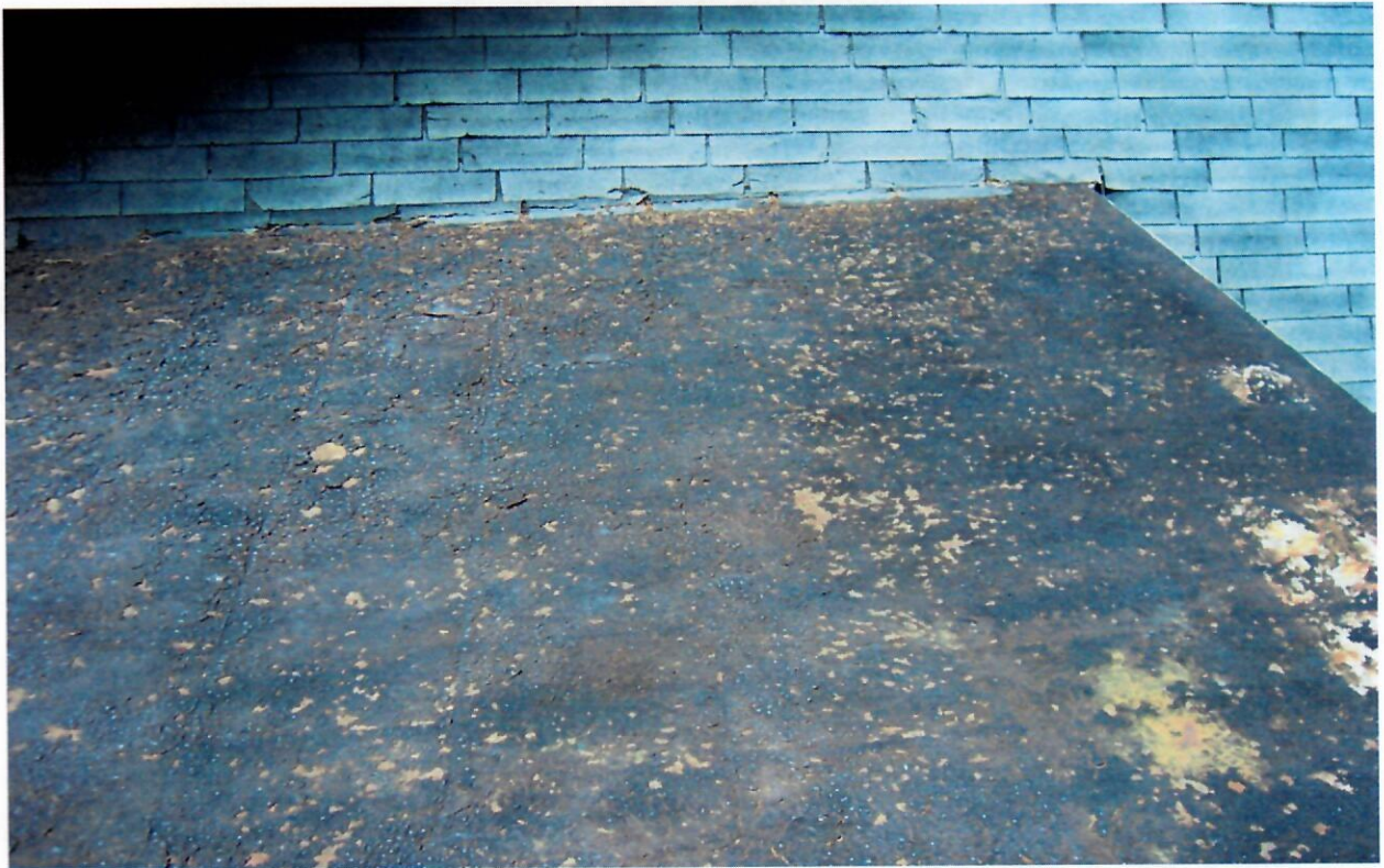
LOW SLOPE ROOF NEEDS REPLACEMENT
