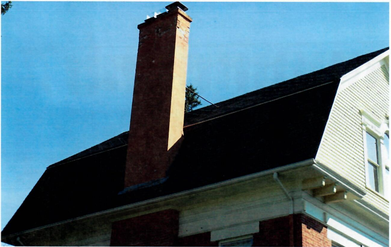
UPPER PORTION NEEDS PAINT REMOVED & REPAIR/REPOINTING
