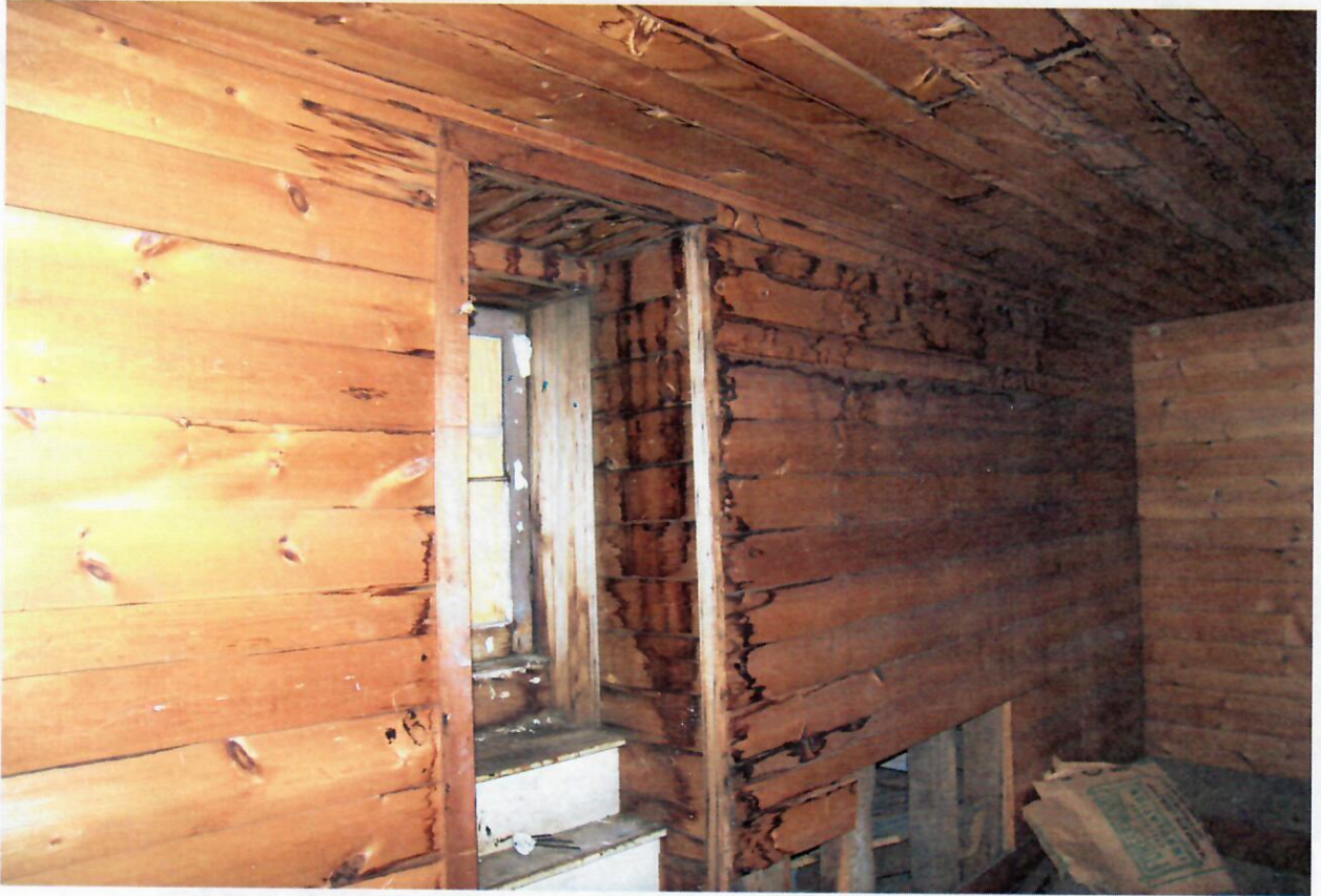
ATTIC WATER DAMAGE ABOVE / OUTDATED REST ROOMS BELOW
