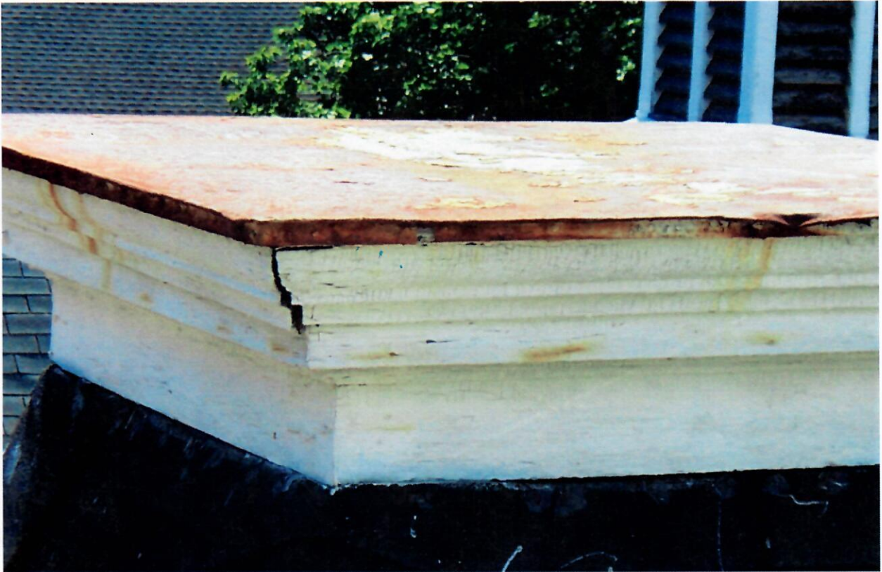
METAL ROOF CAP NEEDS REPLACEMENT
