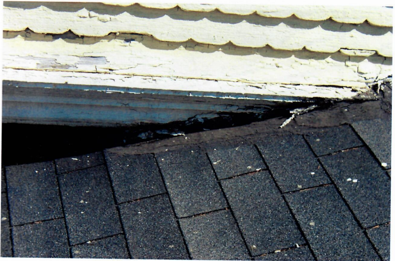
WOOD SIDING SHOULD BE CUT BACK & METAL STEP FLASHING PROVIDED WITH COUNTER FLASHING
