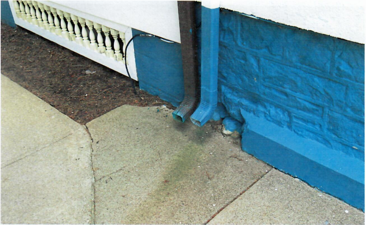
DOWNSPOUTS DRAINING AT GRADE DETERIORATING MASONRY AND WALK / DRAIN FROM BASEMENT
