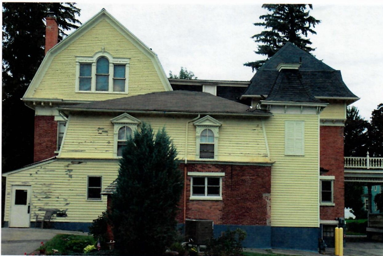
WOOD SIDING & TRIM NEEDS PAINTING EXCEPT AT TOWER - SOUTH SIDE IN WORST CONDITION
