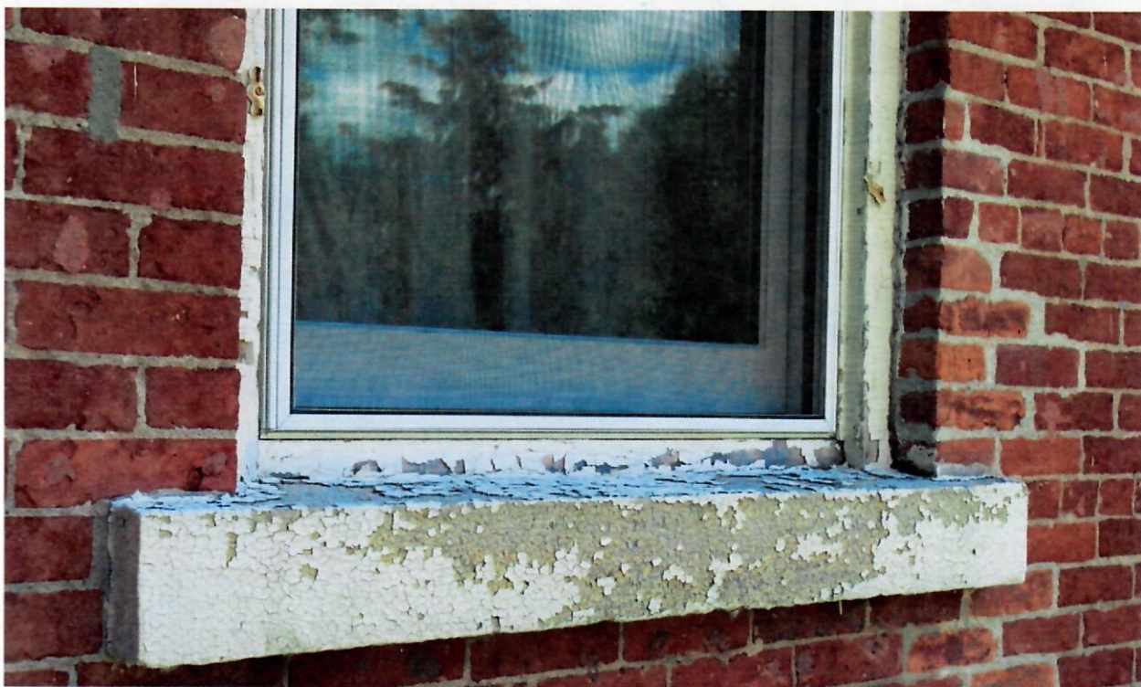
MASONRY SILLS NEED ELASTOMERIC PAINTING
