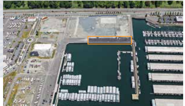
Infrastructure upgrades are necessary to ensure the Port of Everett Marina continues to be an operating asset that meets current and future market demands.
