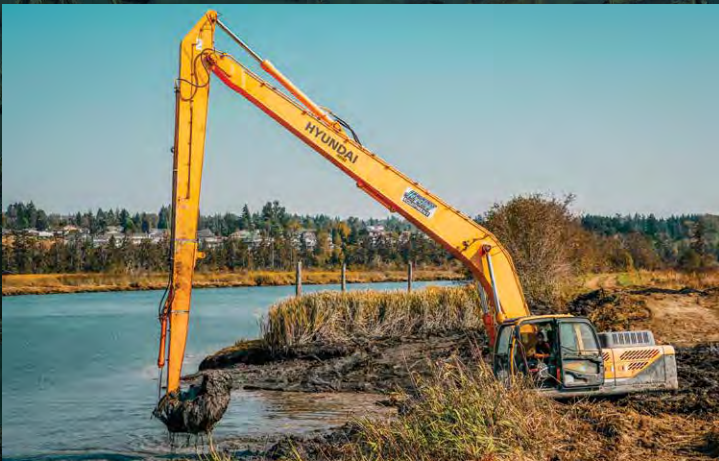
The four dike breaches were completed during low tide, one at a time, with waters flowing into the site with each successive breach. In response to the newly reconnected estuary habitat, salmon, bull trout, and other estuary-dependent species are expected to quickly return to the site.
