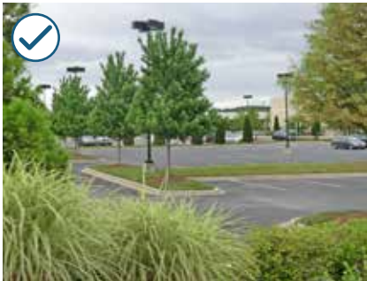
Divide a large parking area into interconnected, small modules with landscape buffers.
