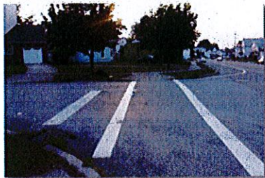
Wide radius curbs increase traffic speed and crossing distance
