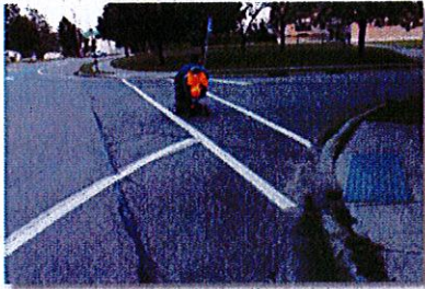
Wide radius curbs increase crossing distance
