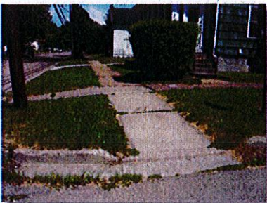
Curb cuts are abrupt and lack textured surface
