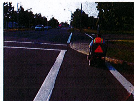
Crosswalk at Main requires pedestrians to move into traffic to reach the curb cut; no crosswalk signal
