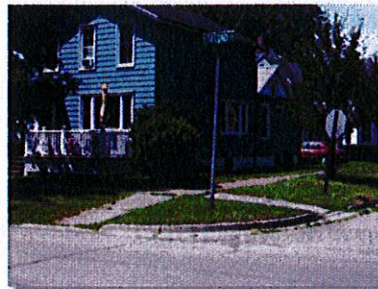
Curb cuts are abrupt and lack textured surface
