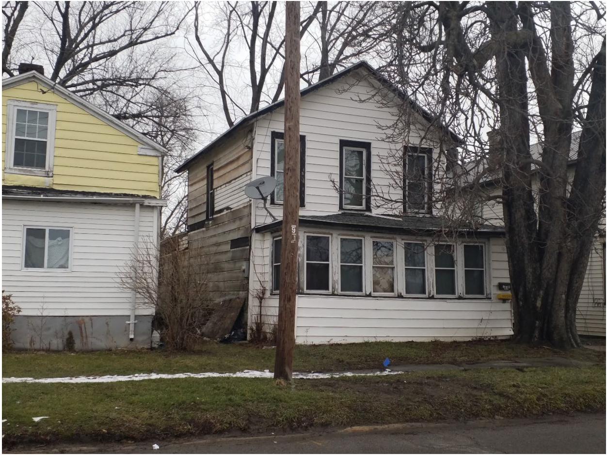
44 West Second: 2 story frame single family on crawl space
