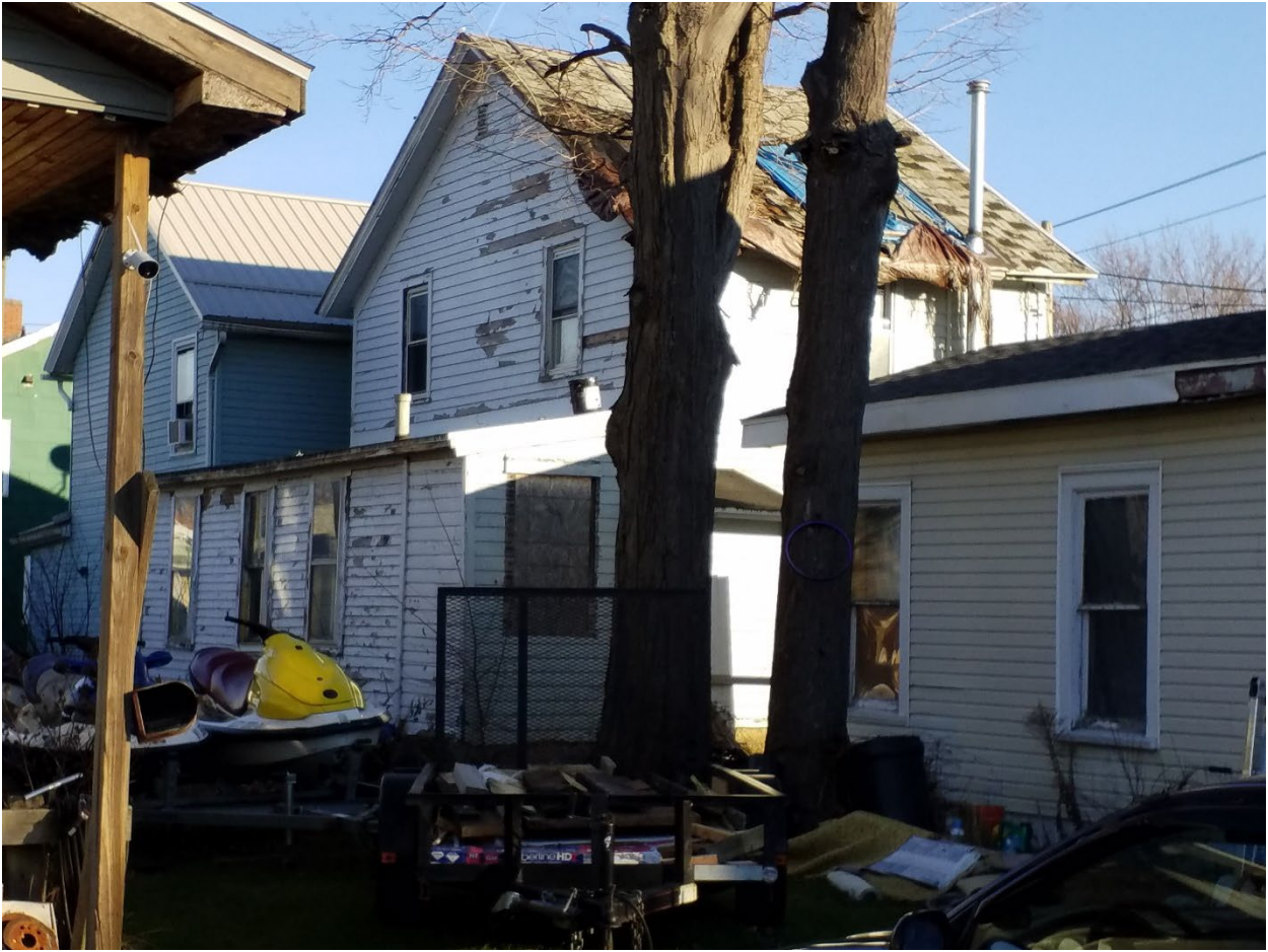
104 West Second Street: 2 story frame single family on partial foundation
