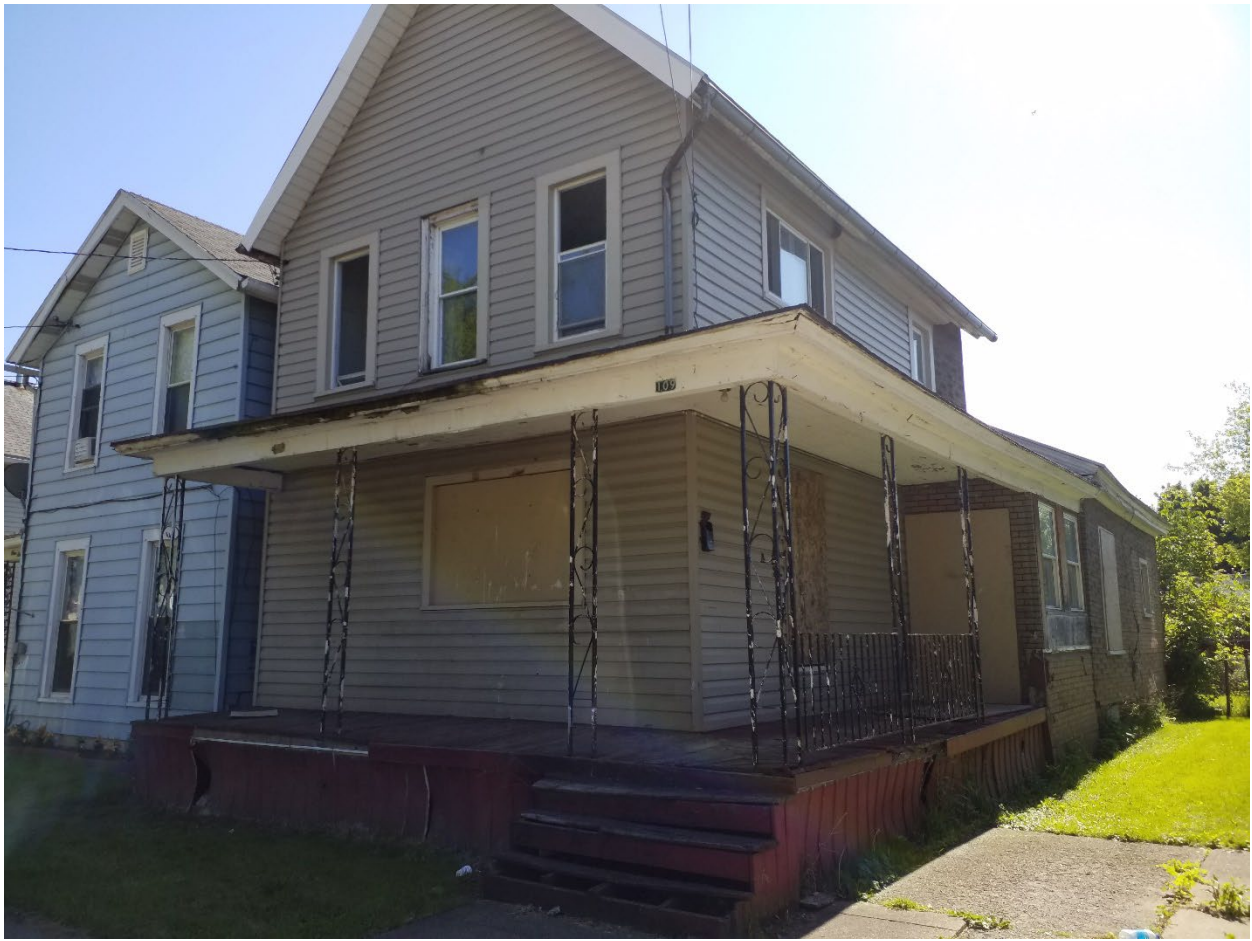
109 South Zebra Street: 2 story frame single family dwelling on basement
