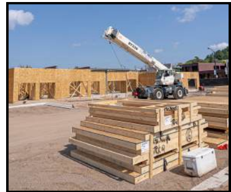
Construction in Iron Mountain
