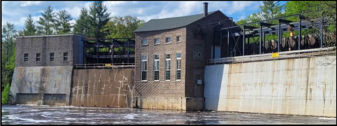
Sturgeon Falls Hydroelectric Dam Photo: CUPPAD
