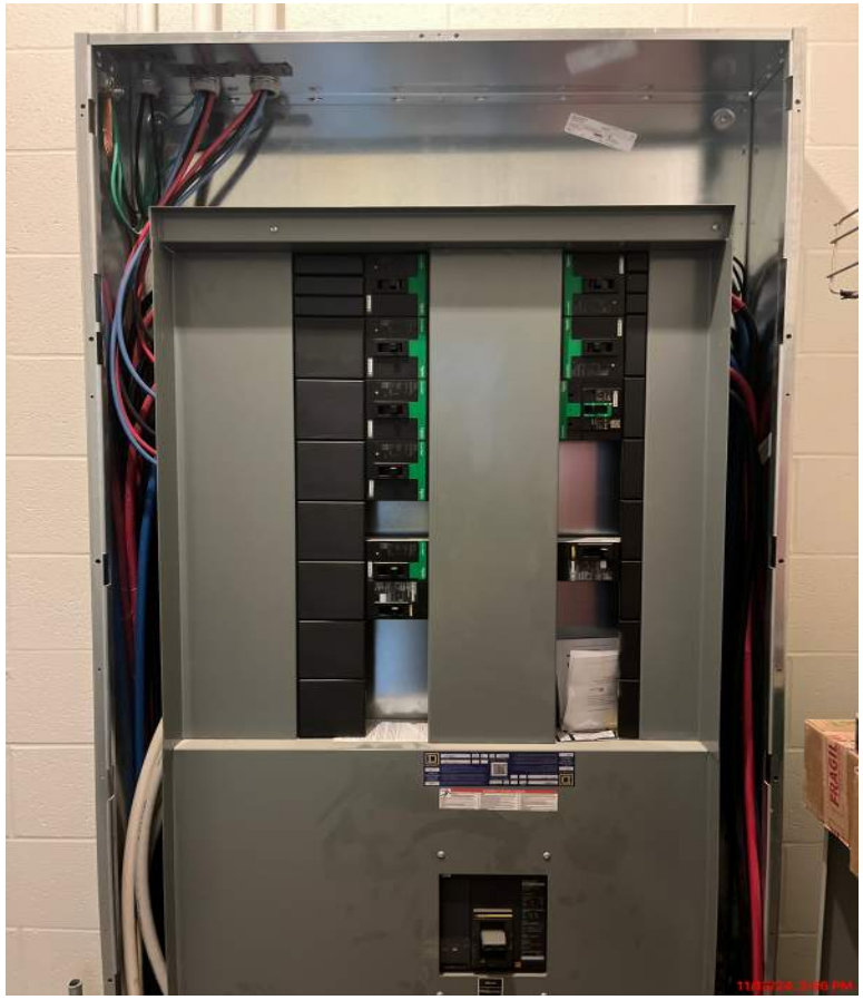
Main Distribution Panel - Installation In-Progress
