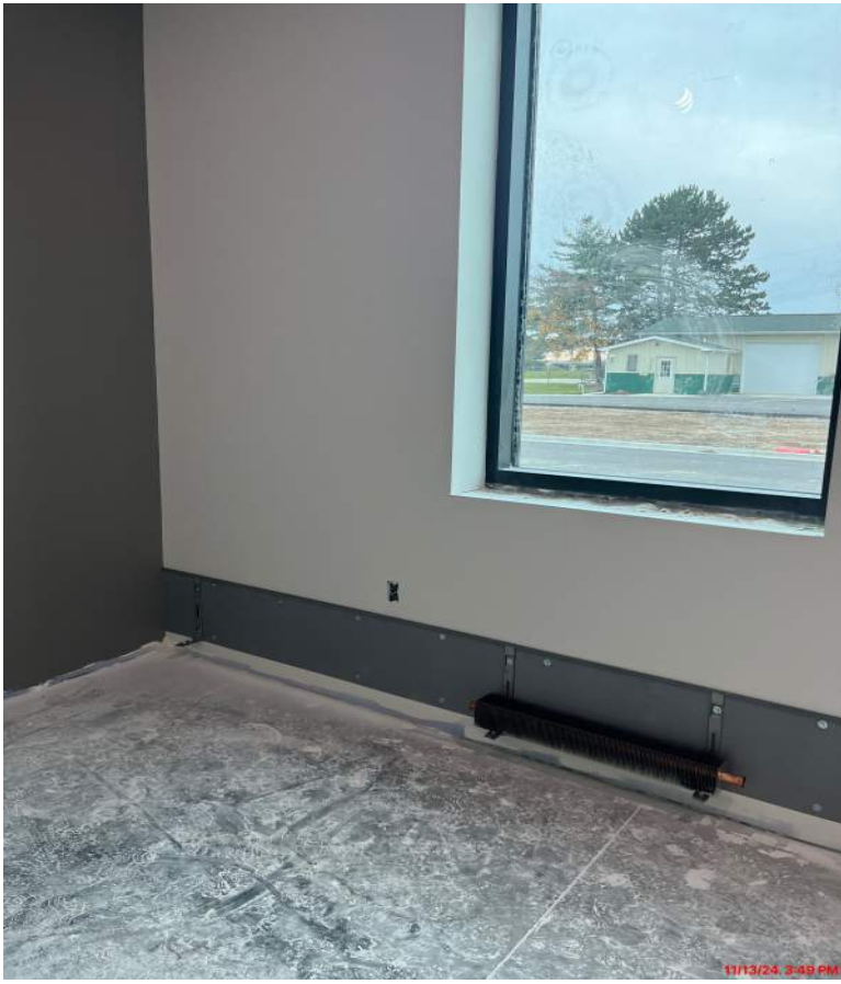
Final Painting and Finned-Tube Radiator Installation
