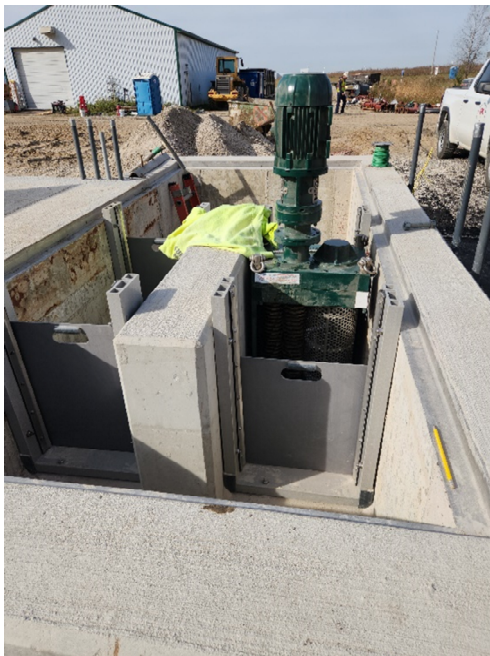
Photo 2: Channel grinders and stop plates placed in the influent channel on 10/22.
