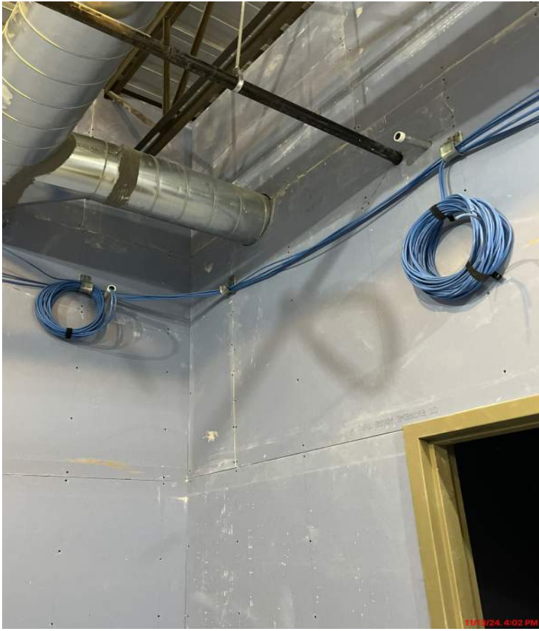
Installation of the Low-Voltage Data Cabling
