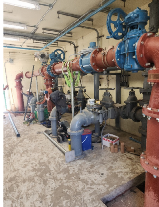
Photo 2: Pump Station Piping placed by 10/16.
