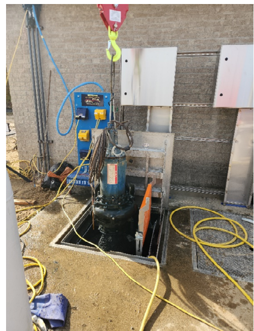
Photo 4: Wet well pumps 1 & 4 replaced and wet well level sensors placed 11/13.
