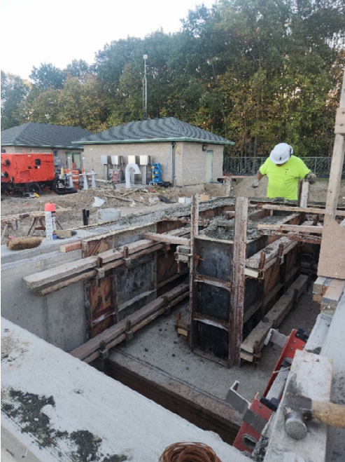
Photo 1: Influent Channel walls placed on 10/07.
