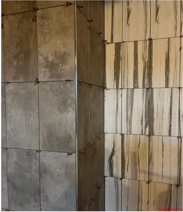
Women's Locker Room - Wall Tile Installation
