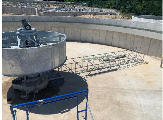
Photo 4: Final Clarifier No. 4 Mechanism
