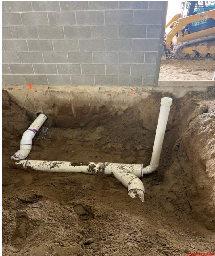
Sheriff Station - Interior Underground Plumbing
