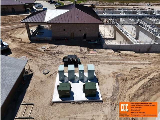
Photo 3: Blower Building Roof and Primary Switches
