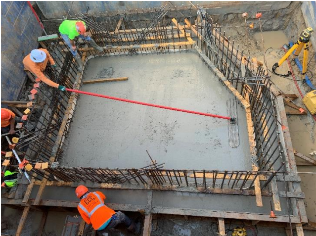
Photo 5: Junction Box No.3 Foundation Slab
