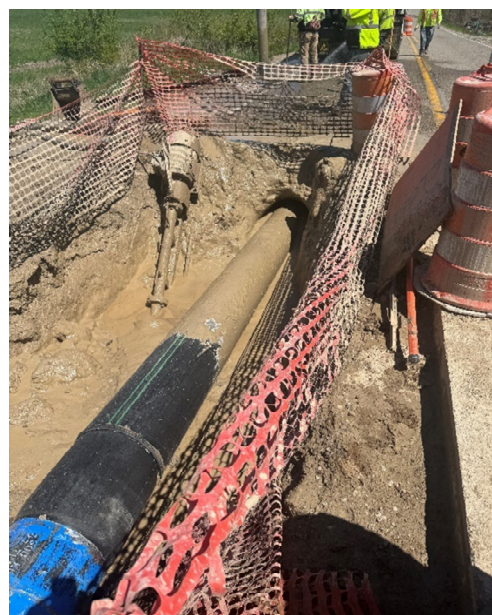
Photo 4: Pulling New Pipe Through Bore Hole.
