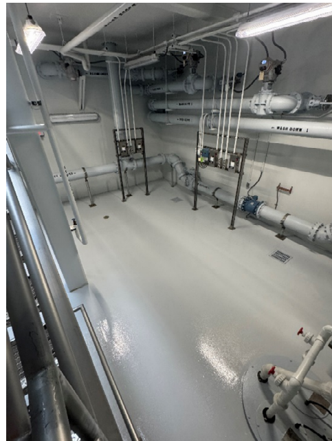
Photo 4: Floor coating placed in the EQ Basin basement and intermediate level by 4/29.
