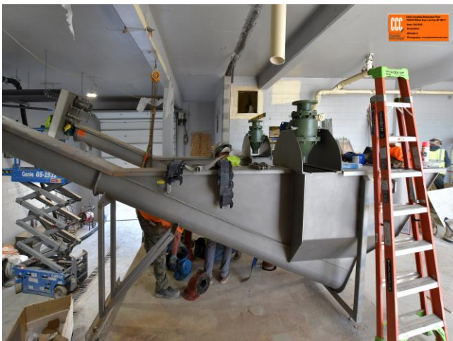
Photo 5: Grit Building Classifier Installation
