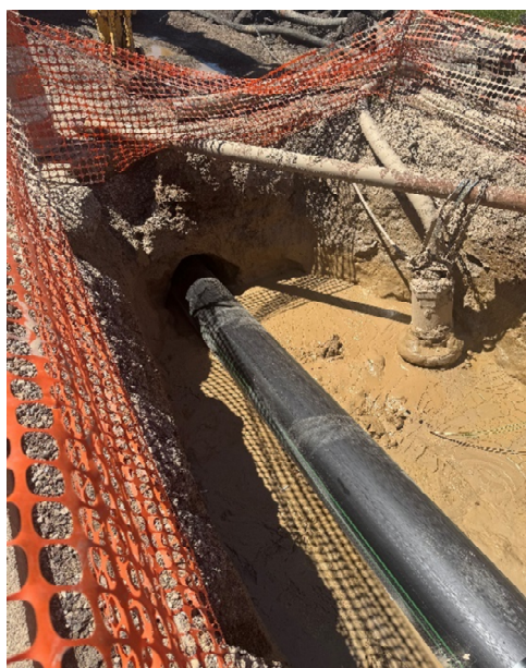
Photo 3: Pulling New Pipe Through Bore Hole.
