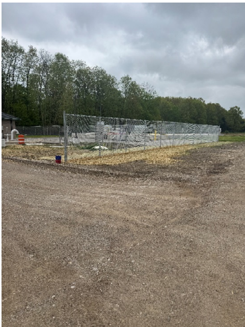
Photo 3: Site work including restoration and grading of aggregate base completed throughout the month of April.
