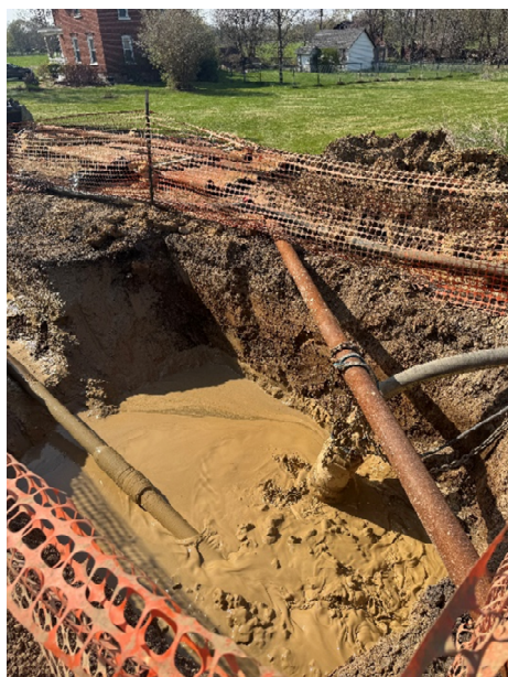
Photo 1: Directional Drilling Pipe Operation
