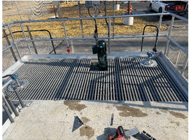
Photo 2: Influent channel FRP grating finalized by 4/17.
