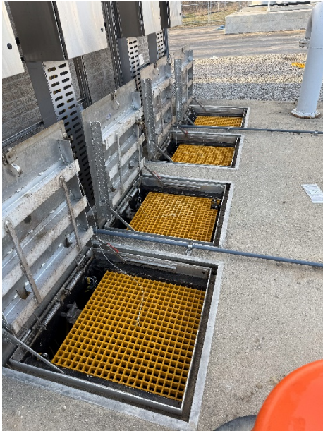
Photo 1: Wet well safety grates finalized by 4/17
