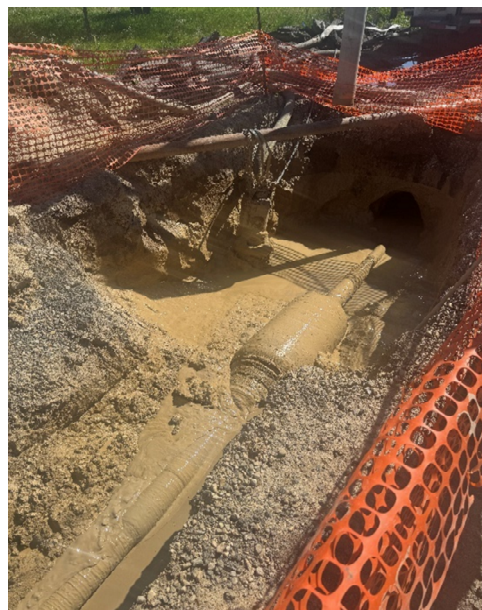
Photo 2: Directional Drilling Pipe Operation
