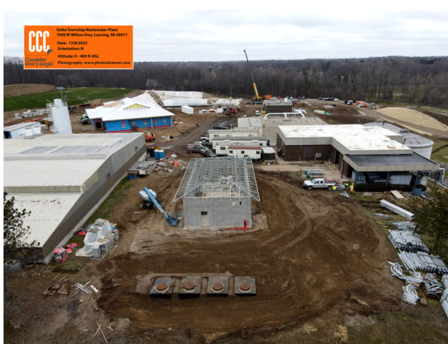
Photo 8: Electrical Building, truss install
