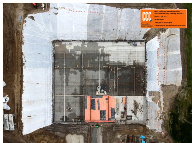
Photo 2: Aeration Tank Foundation, two pours completed
