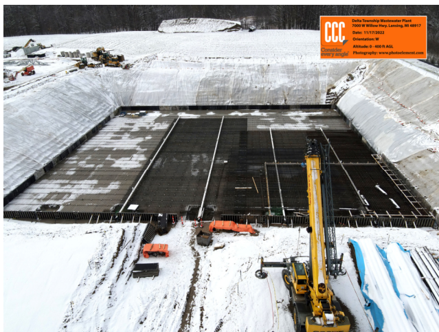
Photo 1: Aeration Tank Foundation, resteel and drain piping progress
