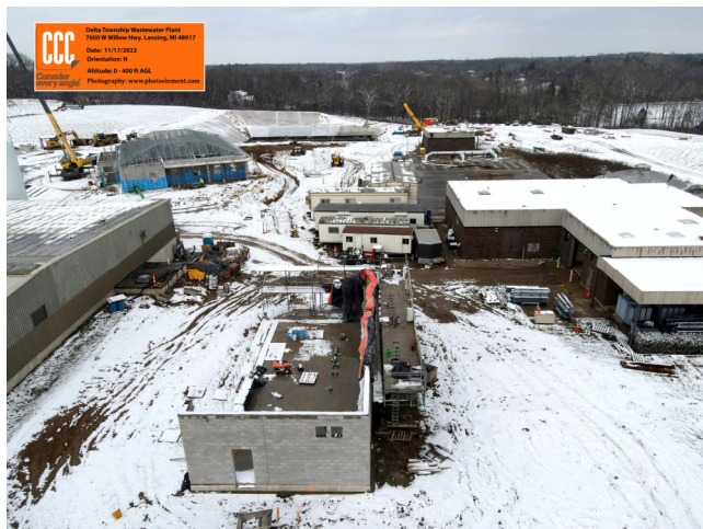
Photo 7: Electrical Building, CMU progress
