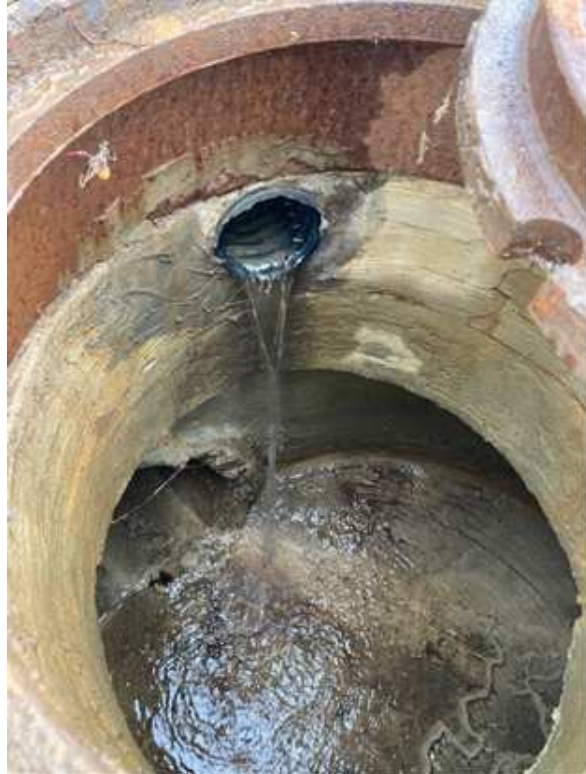
Figure 2 - Outlet pipe from swale to storm structure.
