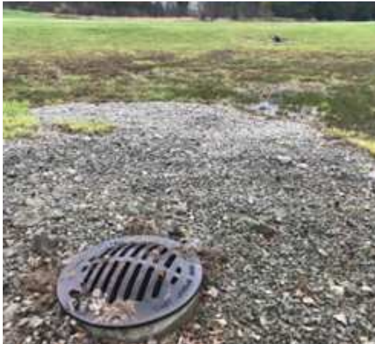
Figure 3 - Riser pipe outlet from the detention system.
