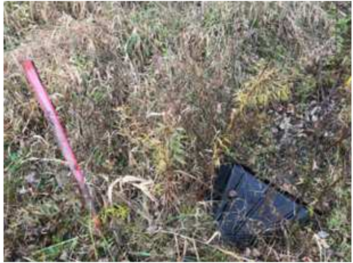
Figure 2 - Outlet pipe from dry detention pond and riser pipe.
