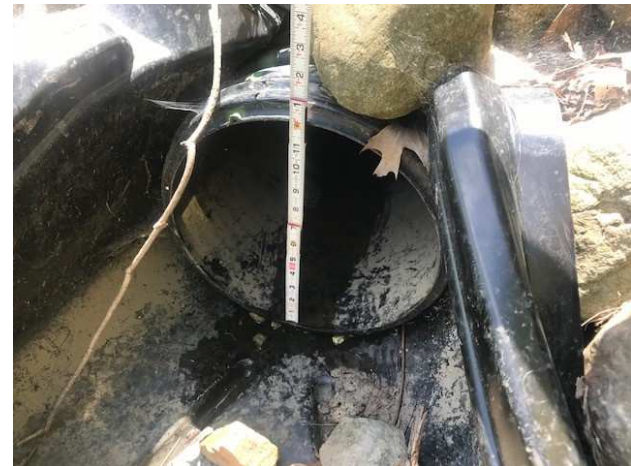
Figure 4 - HDPE pipe to Grand River.
