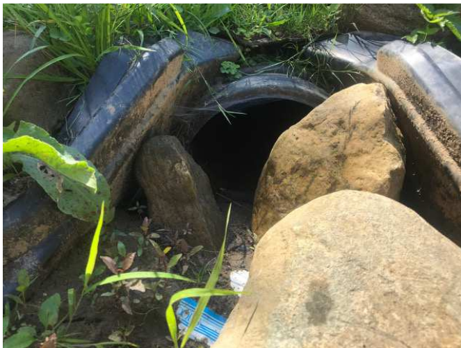
Figure 3 - Outlet swale to the Grand River.
