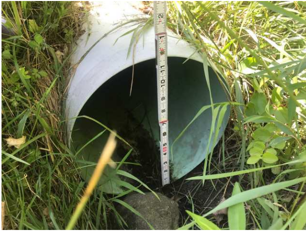
Figure 1 - Outlet pipe of swale.
