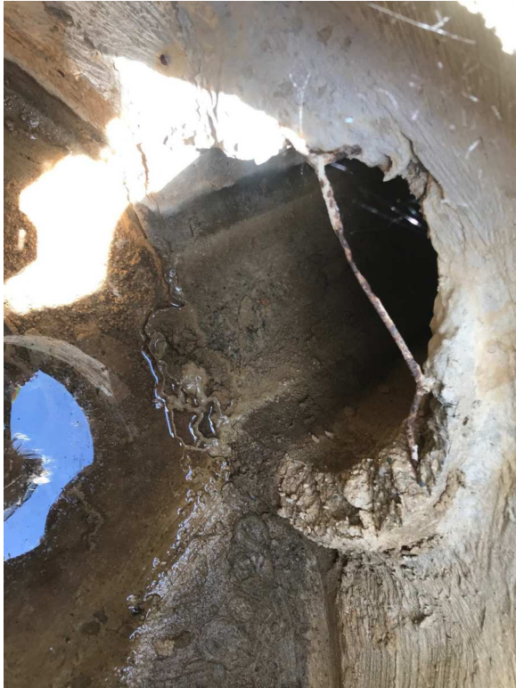
Figure 1 - Outlet pipe from swale to storm structure.
