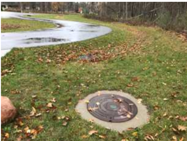
Figure 5 - Swale and BMP structure on site. Despite rainfall, no flow was observed through any of the infrastructure.
