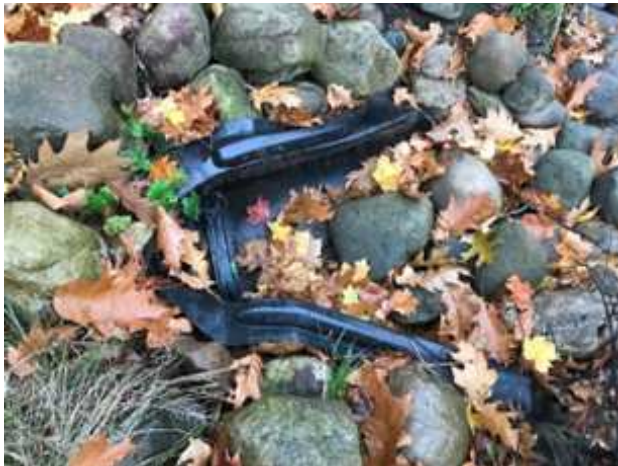
Figure 3 - Outlet pipe to Grand River with rip rap installed.
