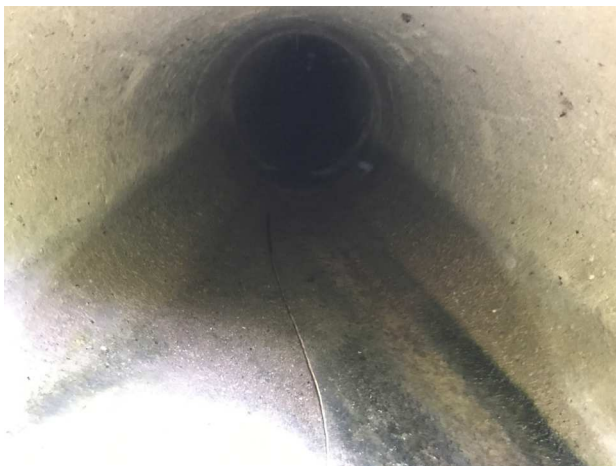
Figure 5 - Outlet pipe labeled 2B. Pipe is in good condition.
