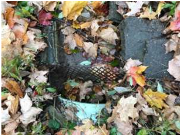
Figure 3 - Outlet pipe of vegetated swale.
