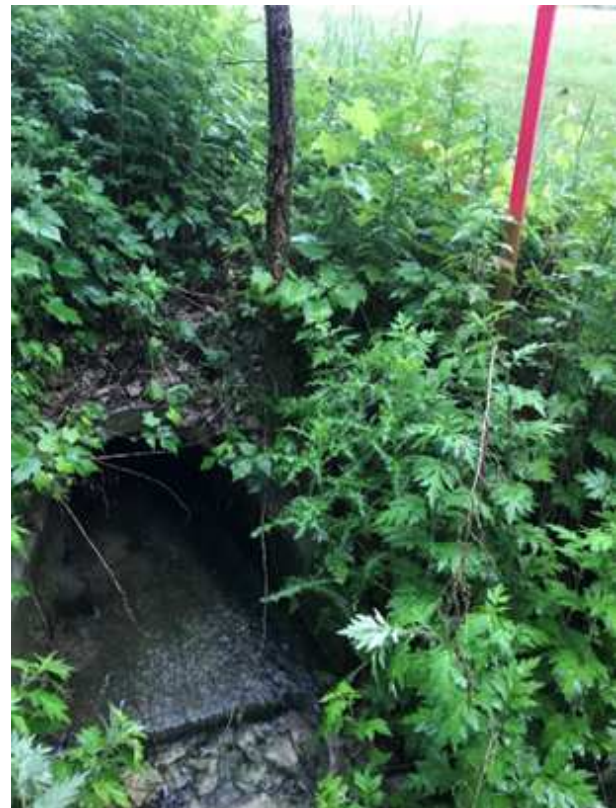
Figure 4 - Outlet pipe labeled 2B. Pipe is in good condition. Photo was taken during a rain event.
