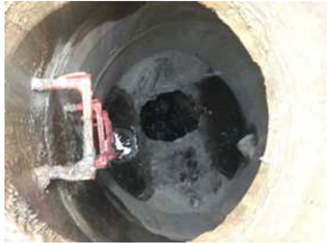
Figure 2 - PVC outlet pipe into storm structure.
