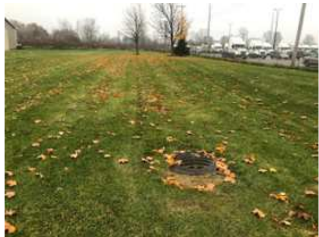
Figure 3 - View of basin. Beehive structure is the outlet of the basin. Note the slope of the basin at right.
