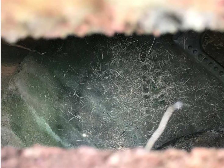
Figure 4 - Interior of beehive outlet. No flow, very dry during each inspection.
