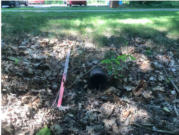
Figure 3 - Pipe under path, drainage for parking area, flows to swale.
