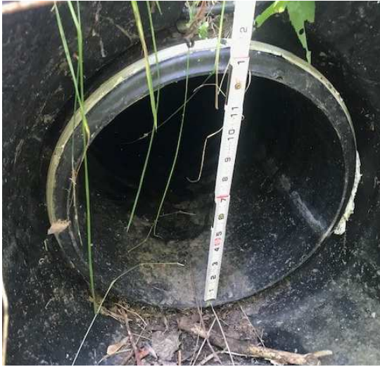
Figure 1 - Outlet pipe from dry detention pond and riser pipe.
