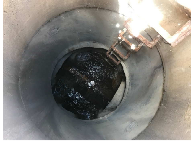
Figure 2 - Manhole south of pond where outlet pipe flows into storm system.
