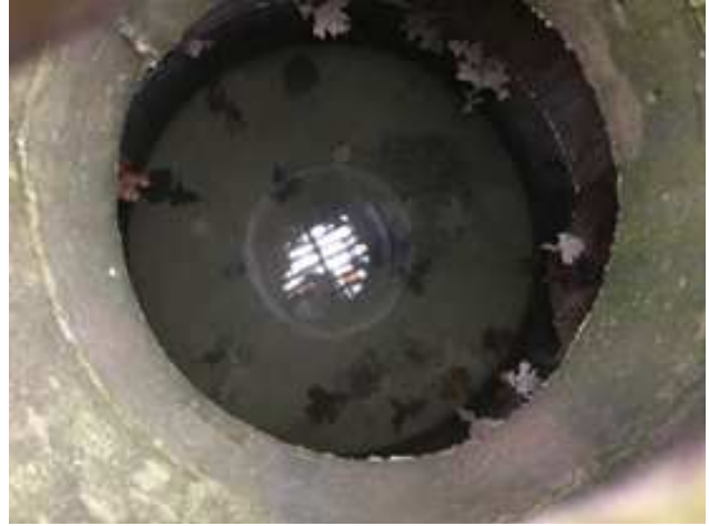
Figure 2 - Outlet structure for swale area. Underdrain flows to structure pictured.
