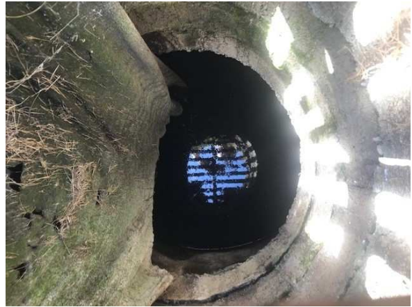
Figure 2 - Inside outlet beehive structure. Note the geotextile fabric at left.
