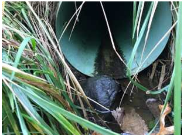
Figure 2 - Outlet pipe of swale.
