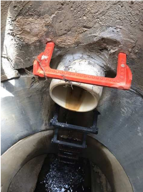
Figure 1 - PVC outlet pipe for underdrain of swale. Photo was taken during dry weather.
