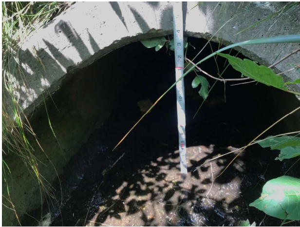
Figure 1 - Outlet pipe labeled 2A. Pipe is in good condition.
