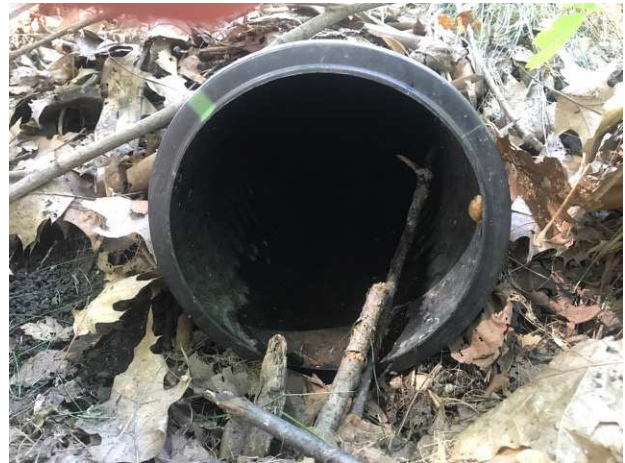
Figure 4 - Pipe under path, drainage for parking area, flows to swale.
