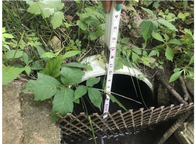
Figure 2 - Outlet pipe of vegetated swale.
