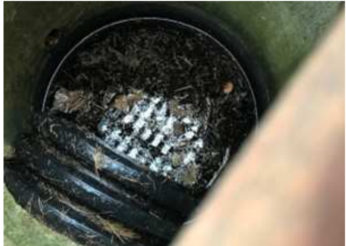
Figure 4 - Inside riser pipe outlet. No flow was leaving from the structure.
