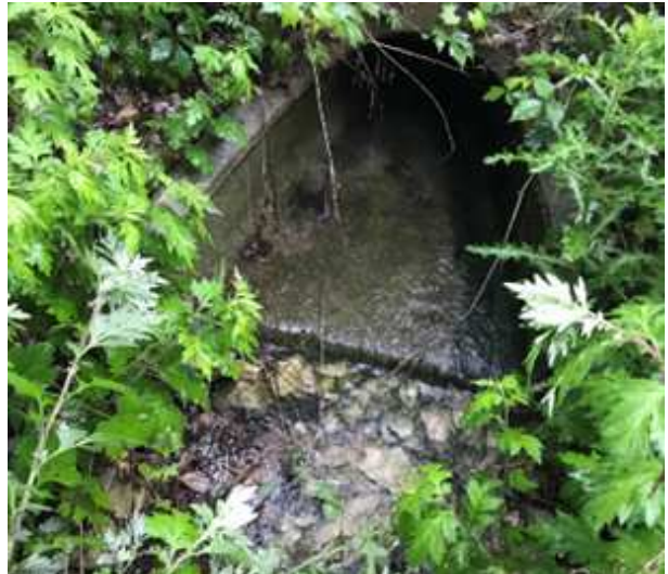
Figure 2 - Outlet pipe labeled 2B. Pipe is in good condition. Photo was taken during a rain event.
