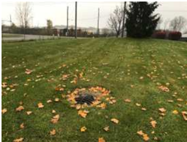
Figure 2 - View of basin. Beehive structure is the outlet of the basin.
