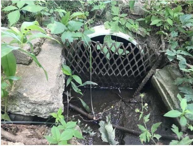
Figure 1 - Outlet pipe of vegetated swale.
