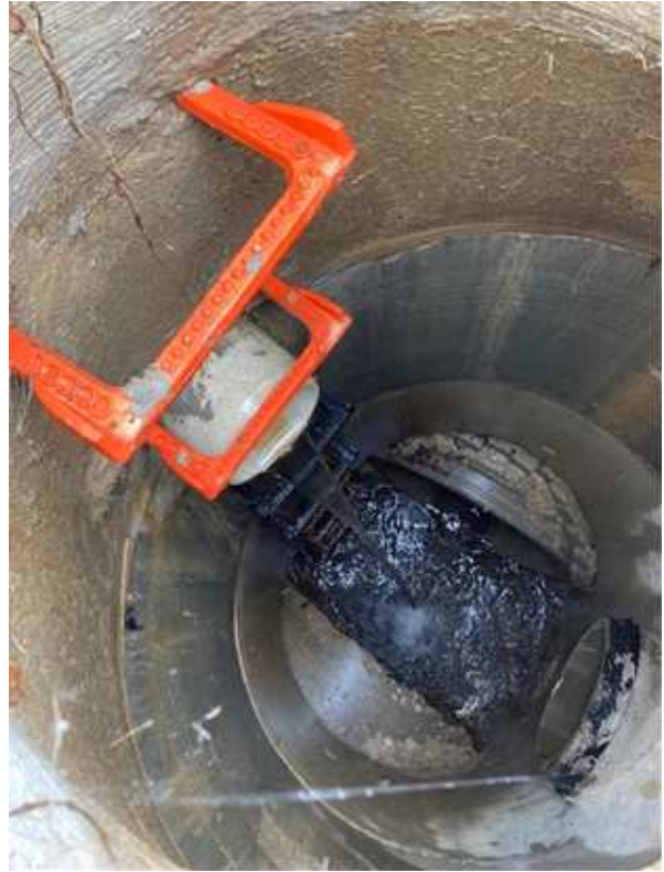
Figure 2 - PVC outlet pipe for underdrain of swale. Photo was taken during dry weather.
