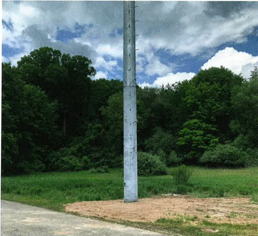
Figure 1. Recently Installed Pole at East Lansing WWRF
