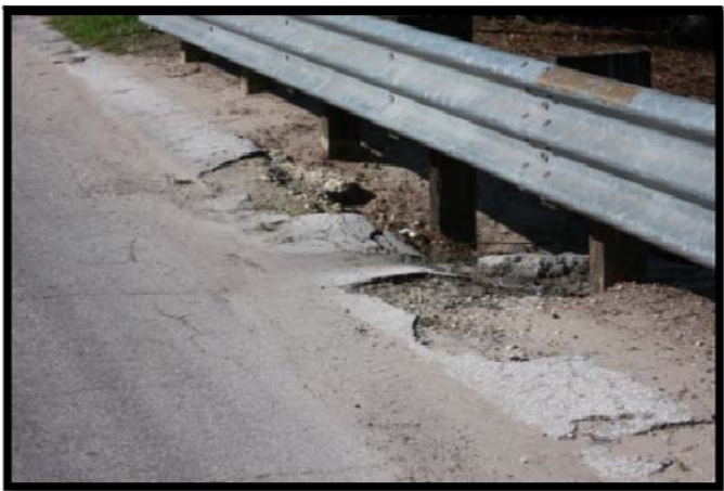
Wilson St. Pavement Failure at canals.
