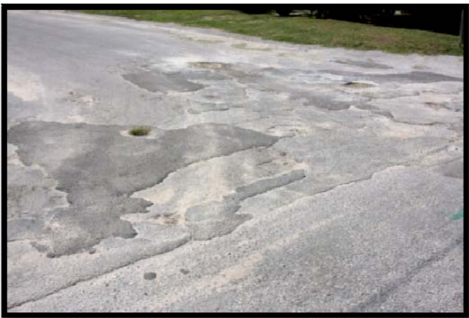
Wilson St. & Ferguson Ave. Pot Holes & Failing Patches
