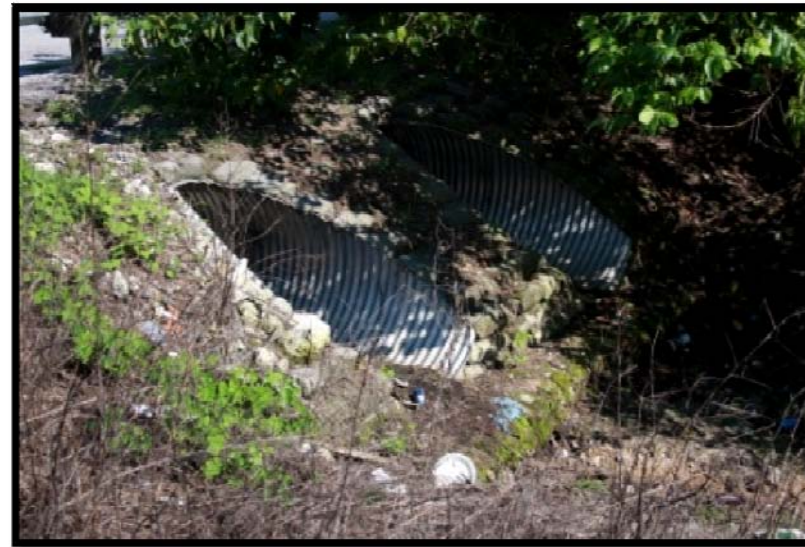
Culverts Openings are Large and Not Secured.
