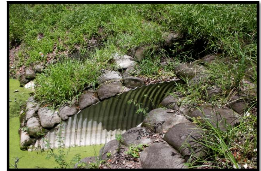
Failing Structure Around Culvert Watch for Possible Pavement Failure Above.
