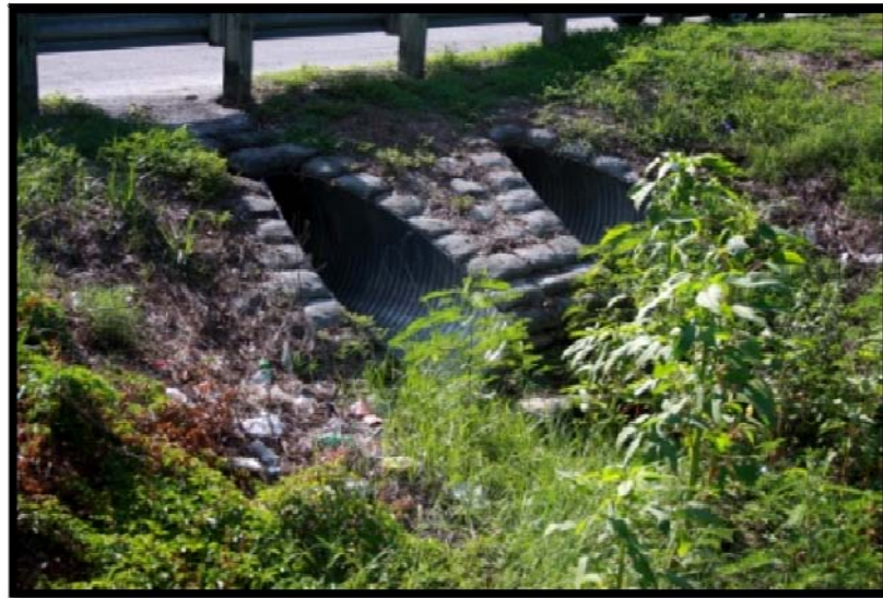
Excessive Vegetation Around Culverts Water Level Remain Low.
