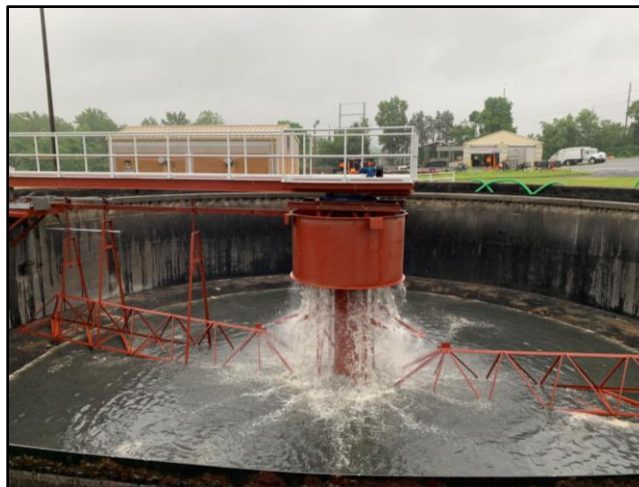
New WPCF Primary Clarifier Drive Assembly
