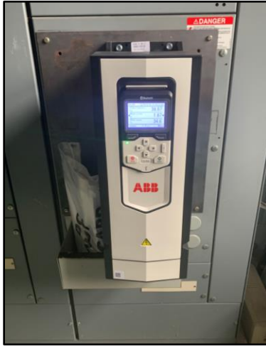
New VFD on a WTP Finish Pump
