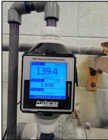
New chemical feed flowmeters at WTP
