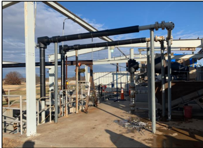
Dragon Jacket insulation system on exposed piping at WPCF Headworks
