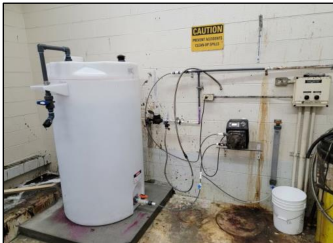
New double wall permanganate storage tank at the WTP
