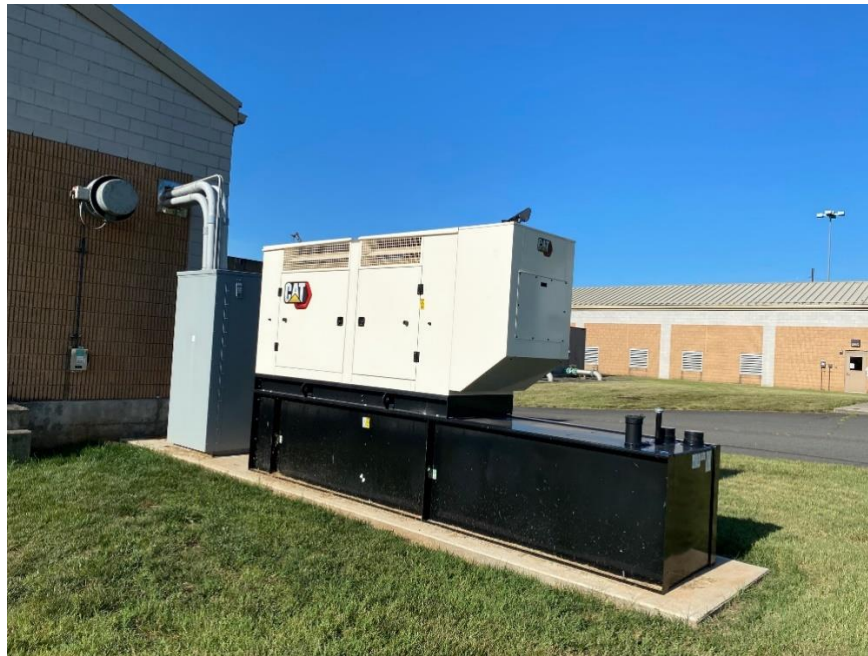
New emergency generator for AWT (UV Disinfection) process (January 2021)
