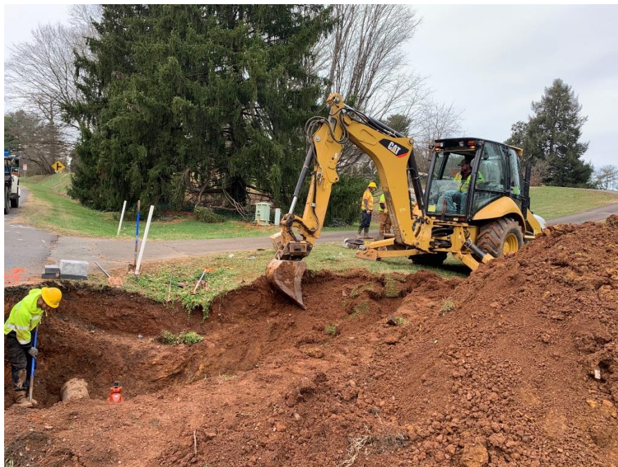
Construction of new 6 inch water distribution main serving the Stoneybrook and Oaklawn neighborhoods (April 2021)
