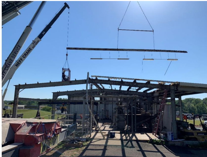
Removed WPCF headworks roof structure and walls for renovation (May 2021)
