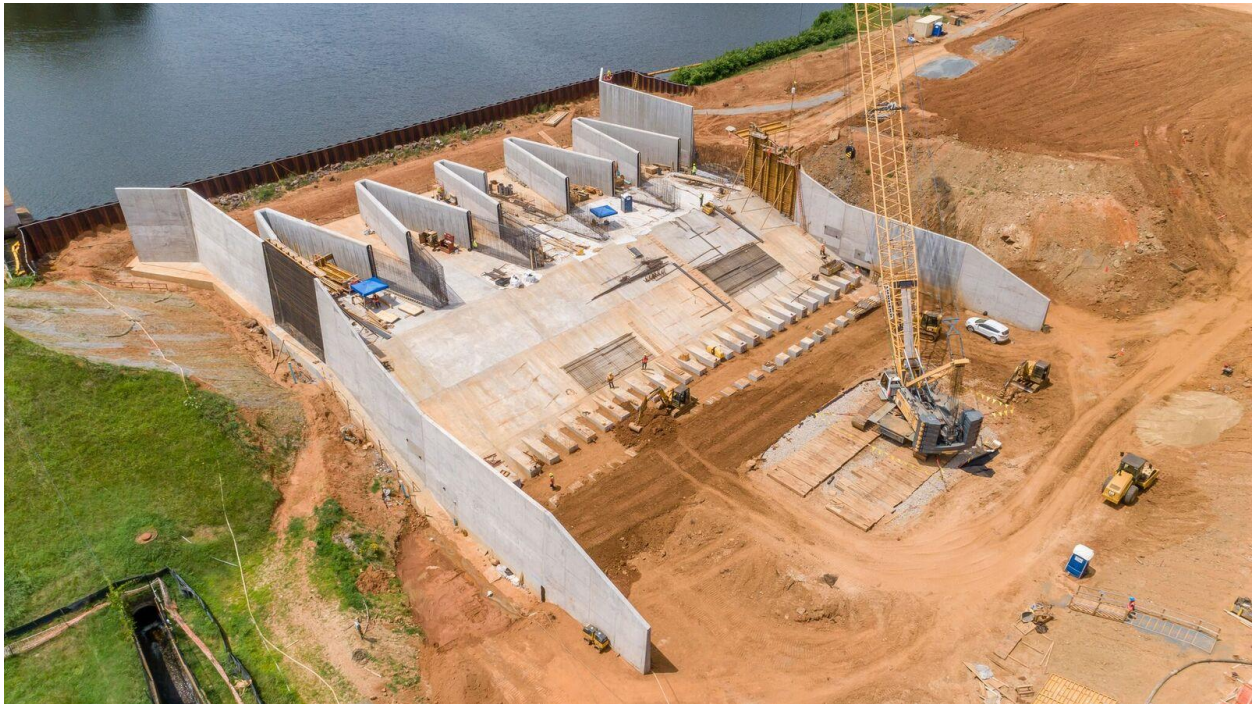
Lake Pelham (MR50) Labyrinth Weir Spillway during Construction, June 2018
