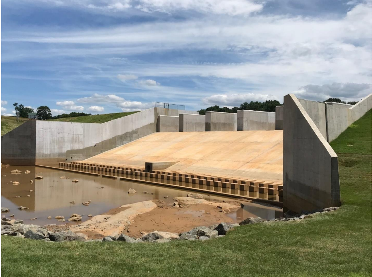
Mountain Run Lake (MR11) Labyrinth Weir Spillway at Final Completion, June 2019
