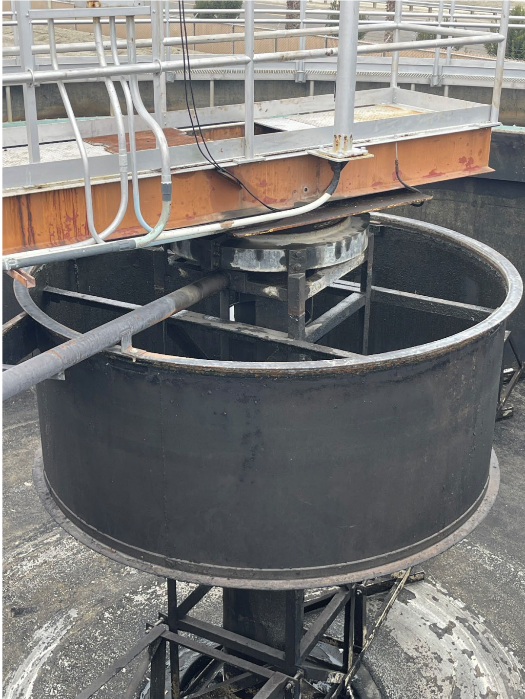
Influent well and support with center column and cage visible
