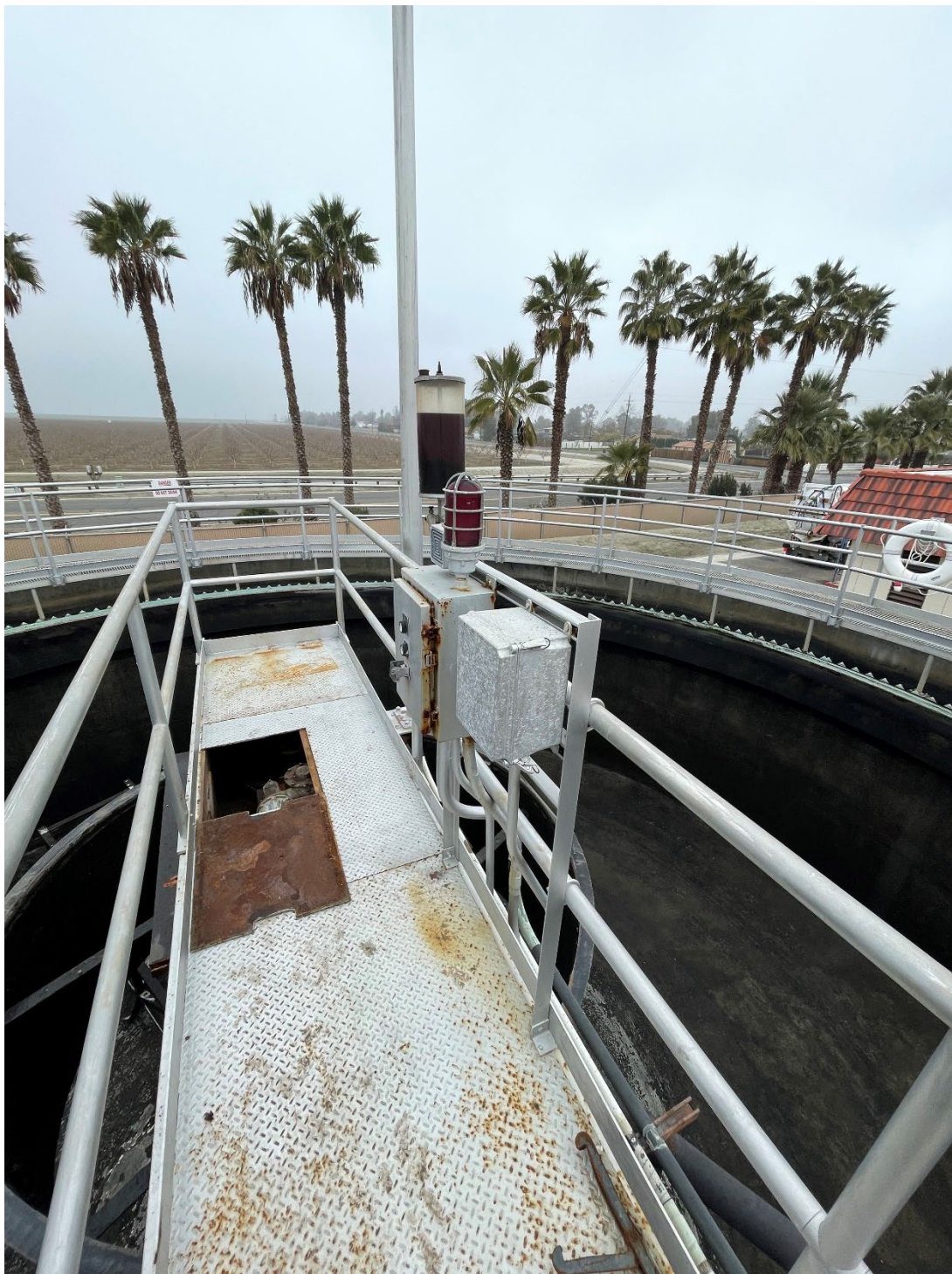
Local control of clarifier drive
