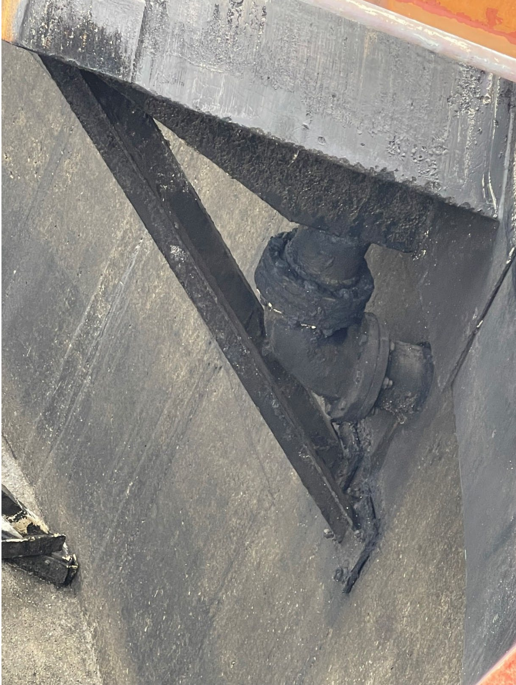
Scum box 6" ductile iron elbow and piping
