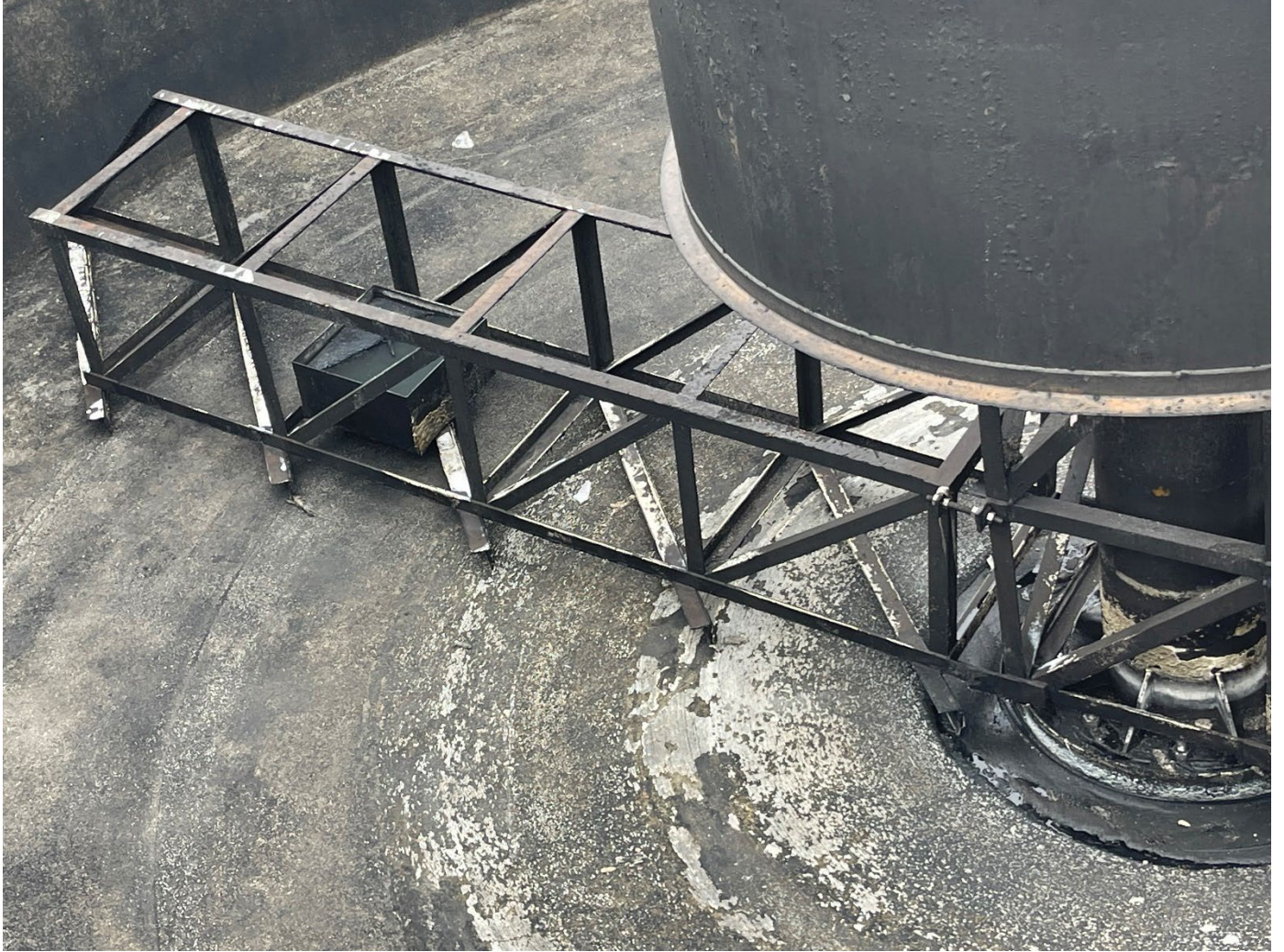
End of trussed rake arm
