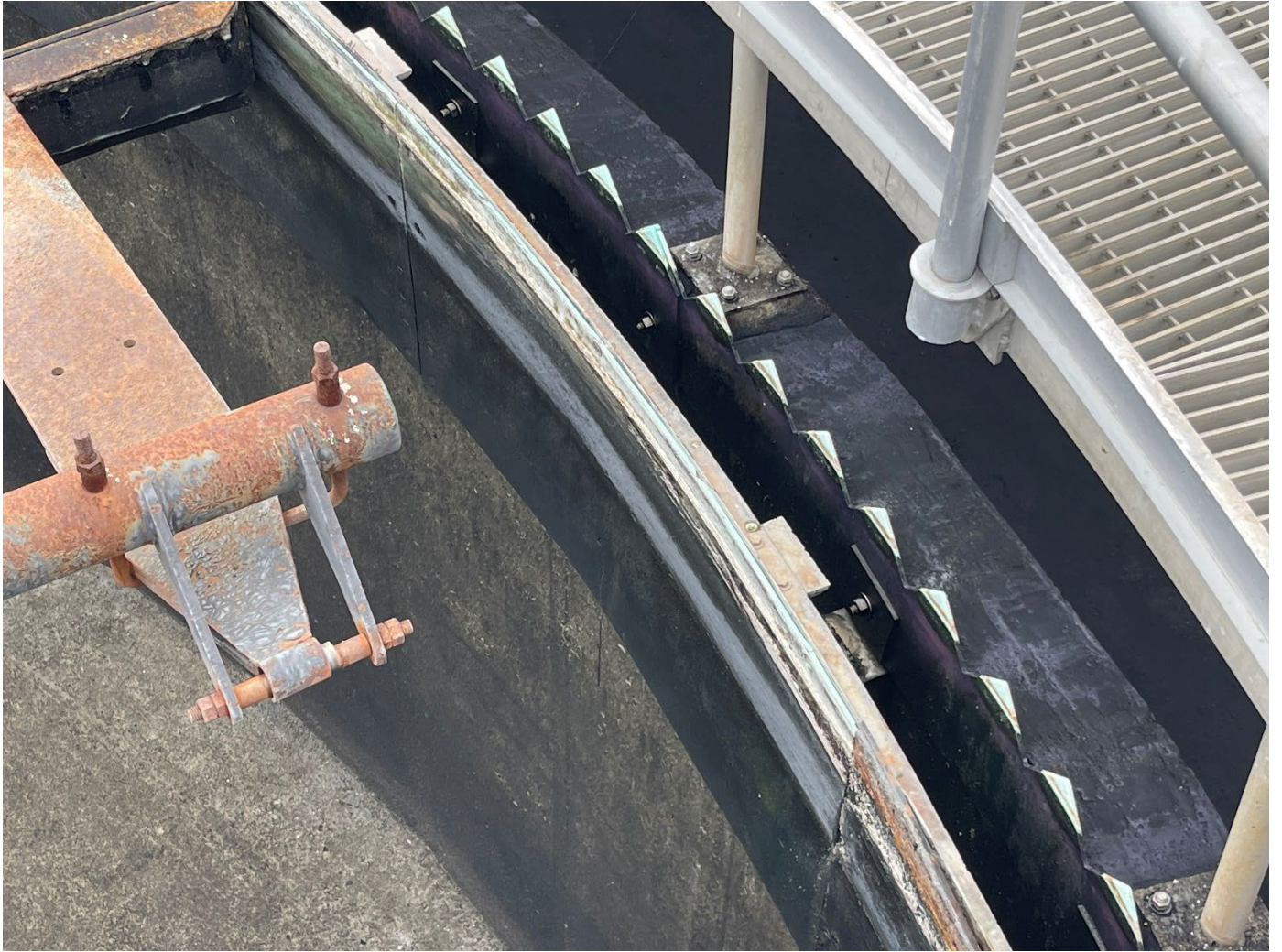
V-notch weirs with visible support and baffle
