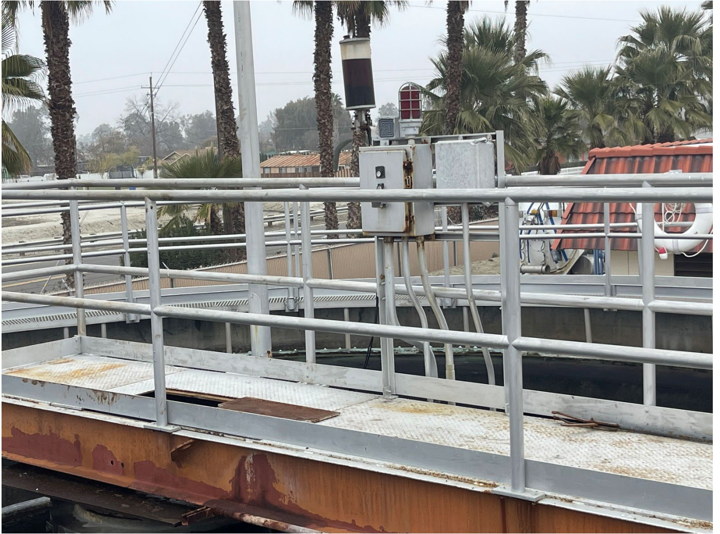
Catwalk and local control of clarifier drive
