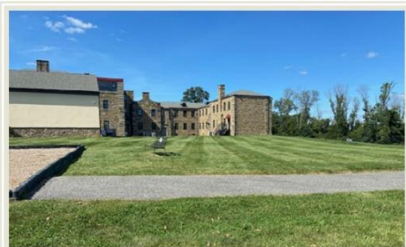
Future site of Concord Bocce Ball.
