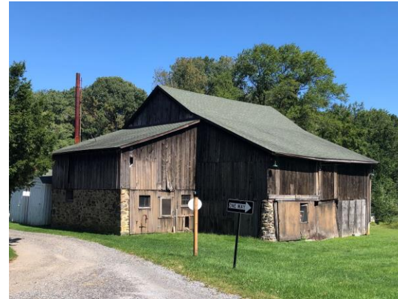
Wilson Palmer Barn at Bush Hill Farm
