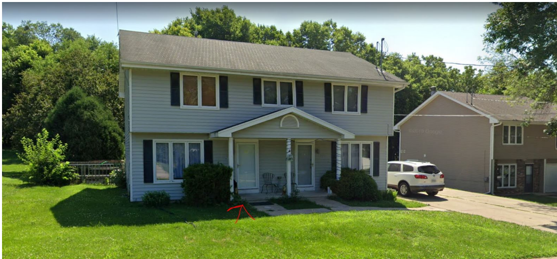
Figure 19: Example of property with a one-step designation for lowest floor elevation estimate
