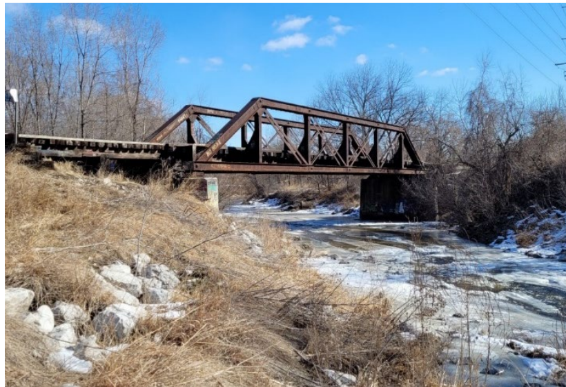
Figure 4: Photo of existing railroad bridge
