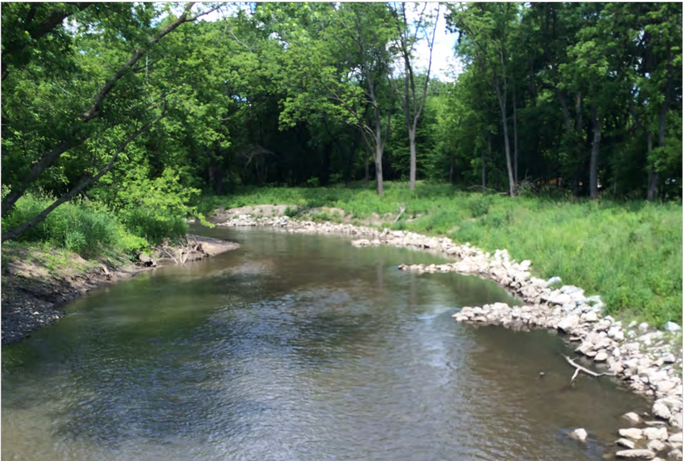
Stream restoration is a process that involves grading, stabilizing and re-vegetating the stream's flood way to help minimize channel erosion and preserve habitat.
