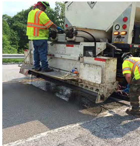
Application of HFST on State Roadway
