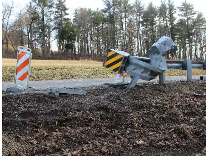
Guardrail damage on Route 28
