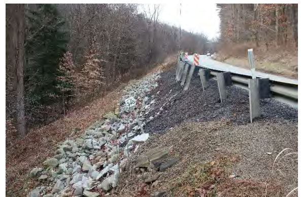
Guiderail erosion repair on Route 28
