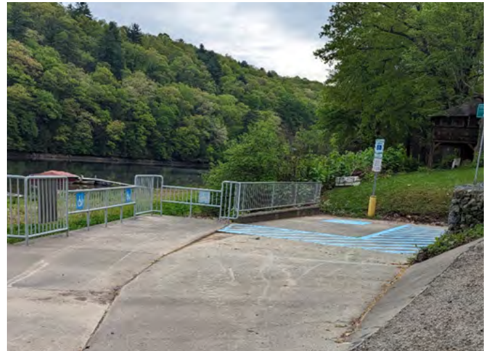
Some of the ADA infrastructure at the Toby Boat Launch
