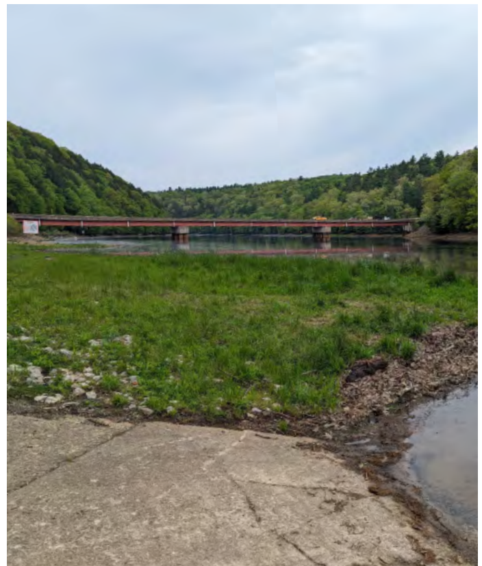
View of the Route 322 Bridge from the Toby Boat Launch in Clarion Borough
