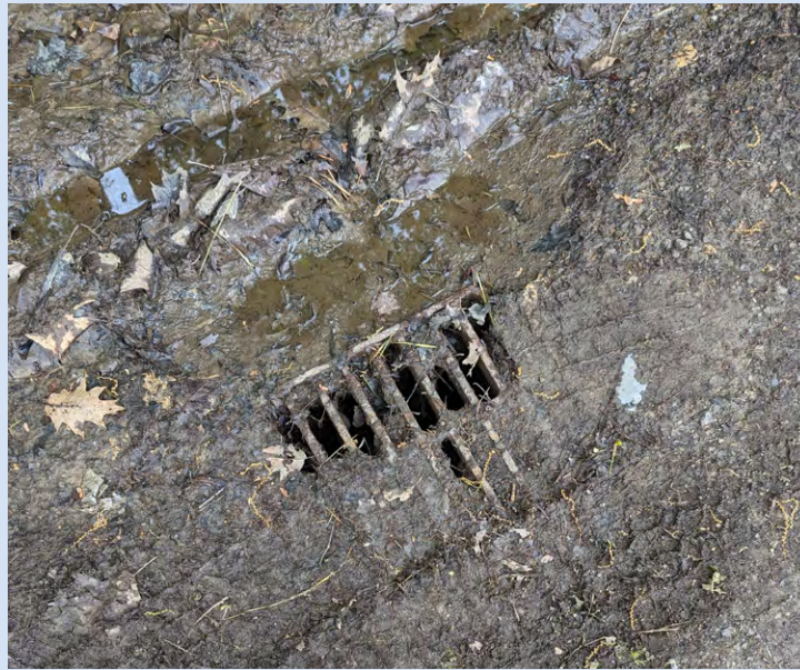
Vehicle maneuvering in tight spaces plus eroding steep slopes combine to exacerbate stormwater concerns
