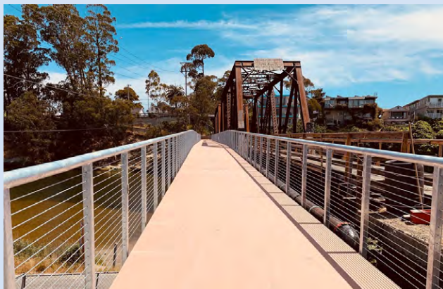
Courtesy of Creative Composites Group: A cantilever sidewalk with aluminum rail
