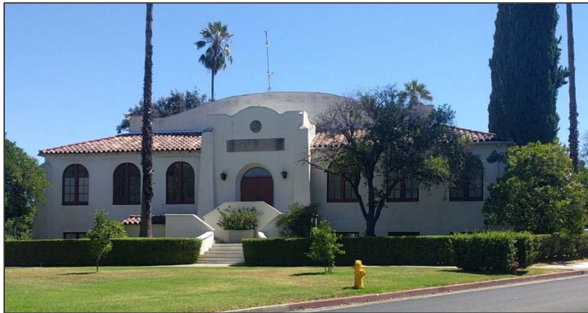
Example of the Mission Revival style, ARG 2020.
