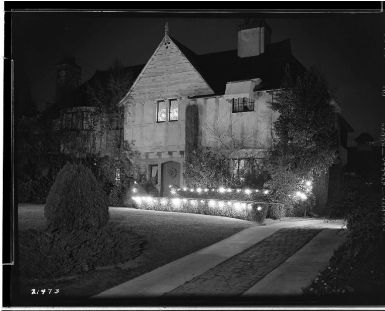
Tudor Revival house in San Marino, n.d. Southern California Edison Collection, The Huntington Library, San Marino, California.
