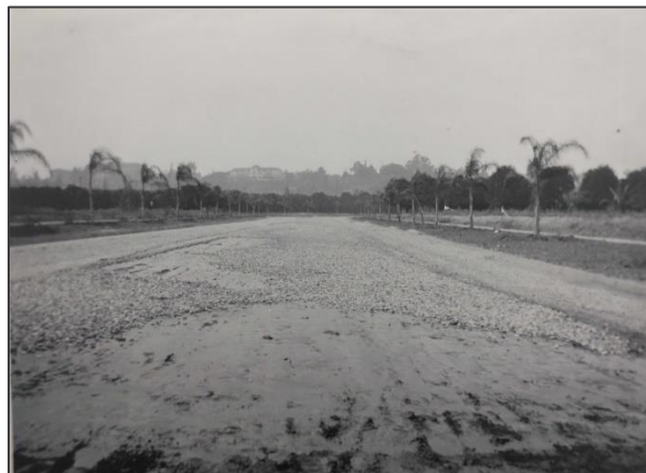
Newly graded road with immature palm trees in Tract 6012, ca. 1923 (Huntington Hotel in background). Huntington Land & Improvement Company Collection, The Huntington Library, San Marino, California.
