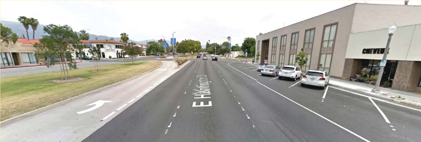
Existing Conditions at Winston Avenue and Del Mar Avenue at Huntington Drive
