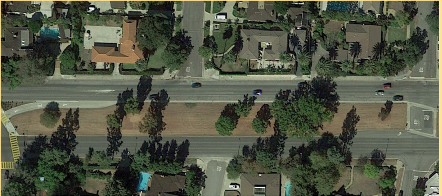
Huntington Drive between Cambridge Road and Bedford Road. A typical cross-section of Huntington Drive.
