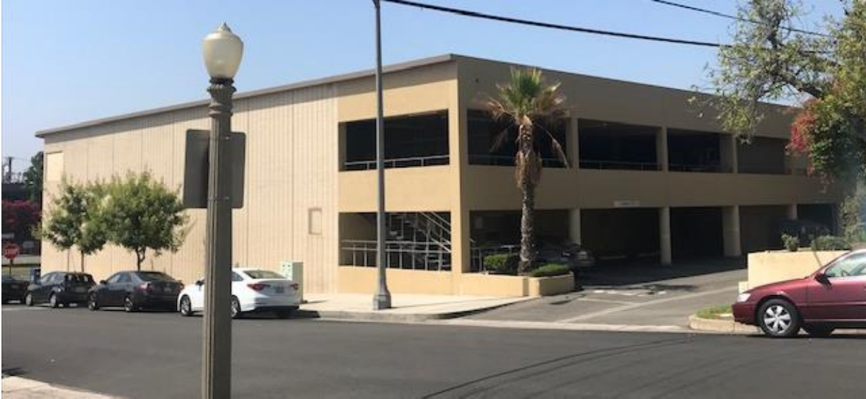
Figure 10: Parking for Wells Fargo Building, 2375 Huntington Dr
