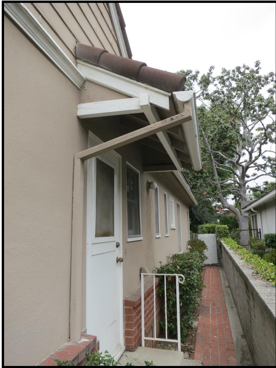
East Elevation North View
