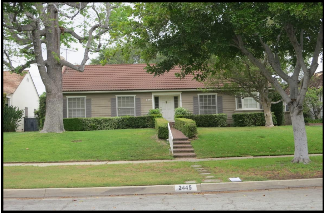
South Elevation North View
