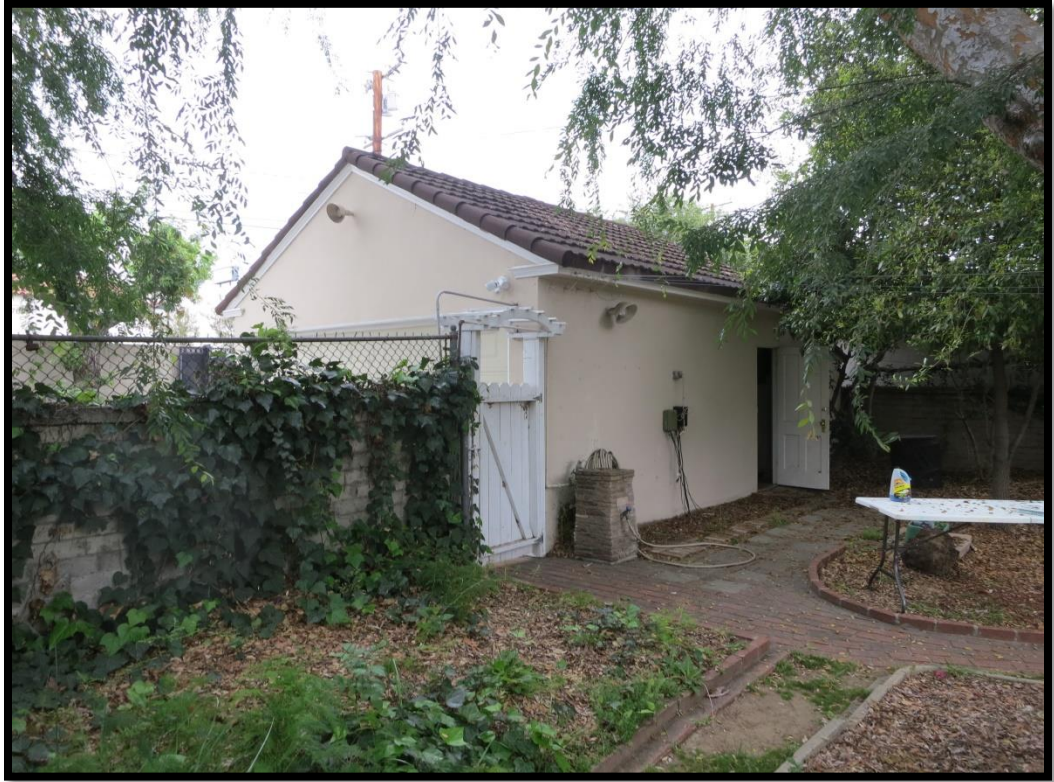
Garage Southwest Elevation North View
