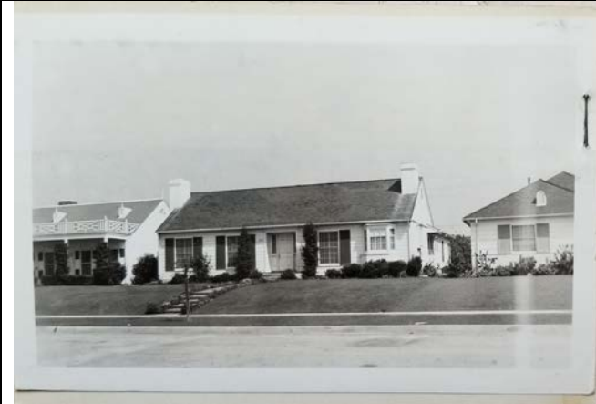
Figure 1. 1941 Photograph South Elevation
