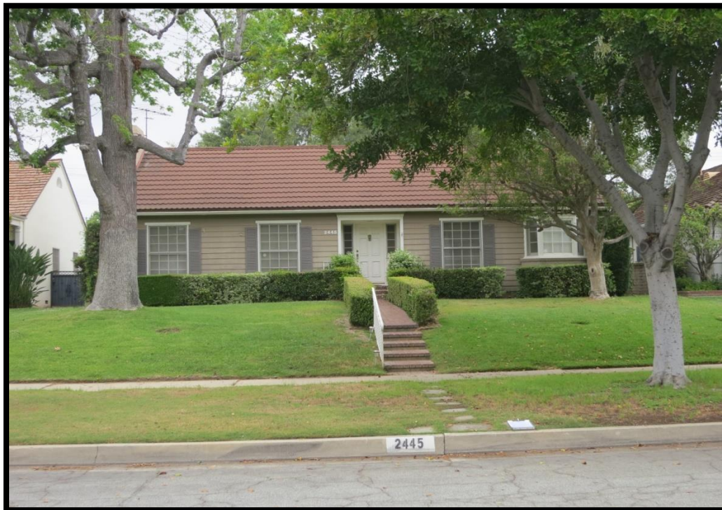
Figure 1. Subject Property Primary South-Facing Facade
