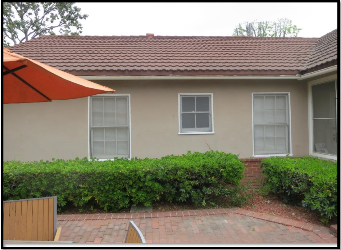
West Elevation North Wing
