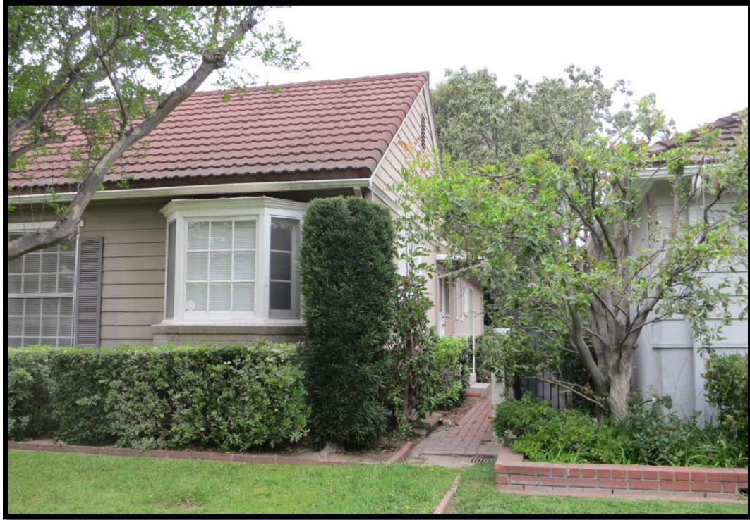
Southeast Elevation View North 1
