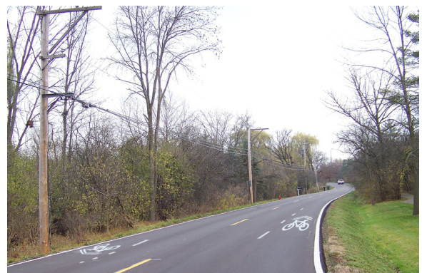
After: installation of a sharrow is a cost effective way to designate a road as a preferred bike route.
