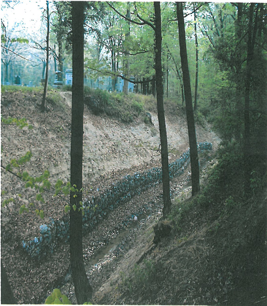
A restored Ravine: Some vegetation removed to improve light. The banks have been replanted with native forbes that will send roots deep into the bank to help stabilize once the weather warms (photo taken in early May). Bottom channel lined with Gabions and Check Dams installed to slow water flow.
