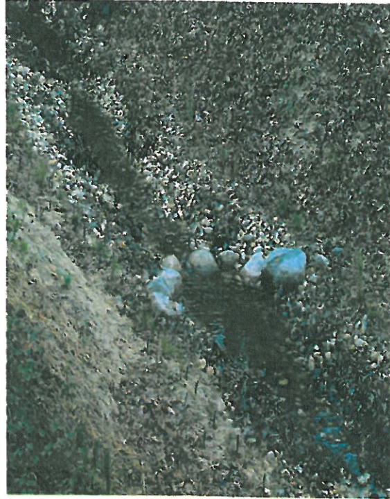
Water flow is slowed by Check Dam like the one pictured above. The rocks shown sit on top of a Gabion Basket buried in a ravine and covered with small stones
