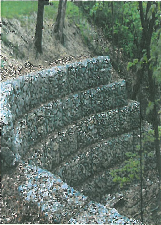
Gabion Baskets lining a steep slope for support
