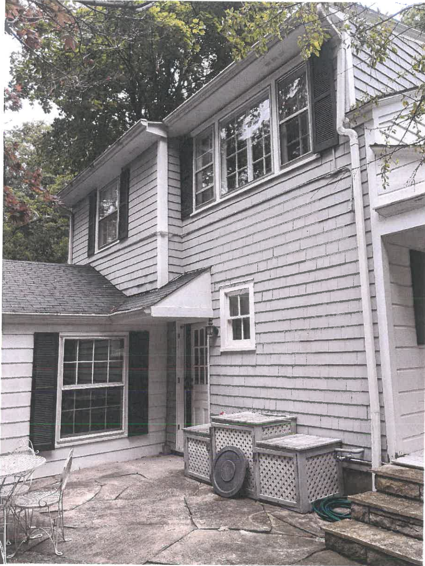
Main House (West Elevation)
