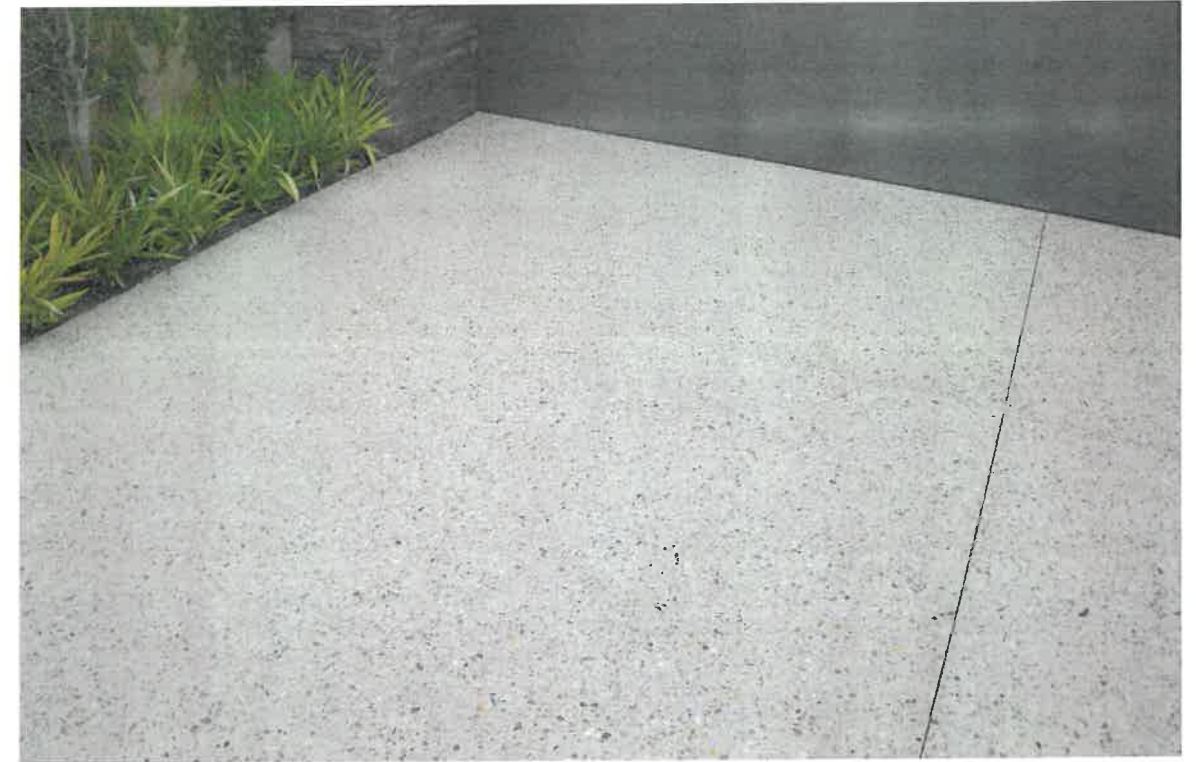
TOP RIGHT: EXPOSED AGGREGATE DRIVEWAY: BOTH EXISTING CONCRETE PAVER DRIVEWAYS TO BE REPLACED WITH EXPOSED AGGREGATE CONCRETE.
