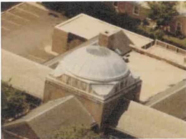
Figure 1. Original lead-coated copper roofing on the library in 1978, with a neutral gray patina.
