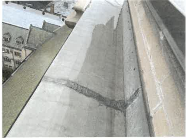
Figure 2. Tin-zinc-alloy coated copper gutter installed in Evanston in 2009. After thirteen years of weathering, it has a neutral gray patina.
