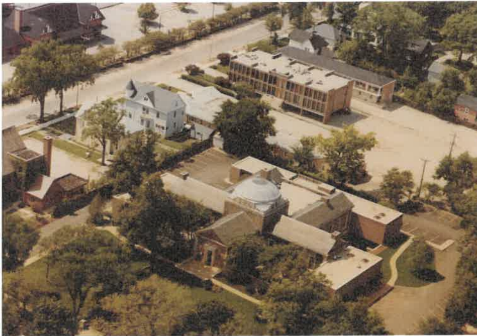
Figure 7. Aerial view, 1978, after completion of the additions to the library. Note the light gray color of the dome, the staining of the masonry below, and the gutter and downspouts atop the limestone watertable.
