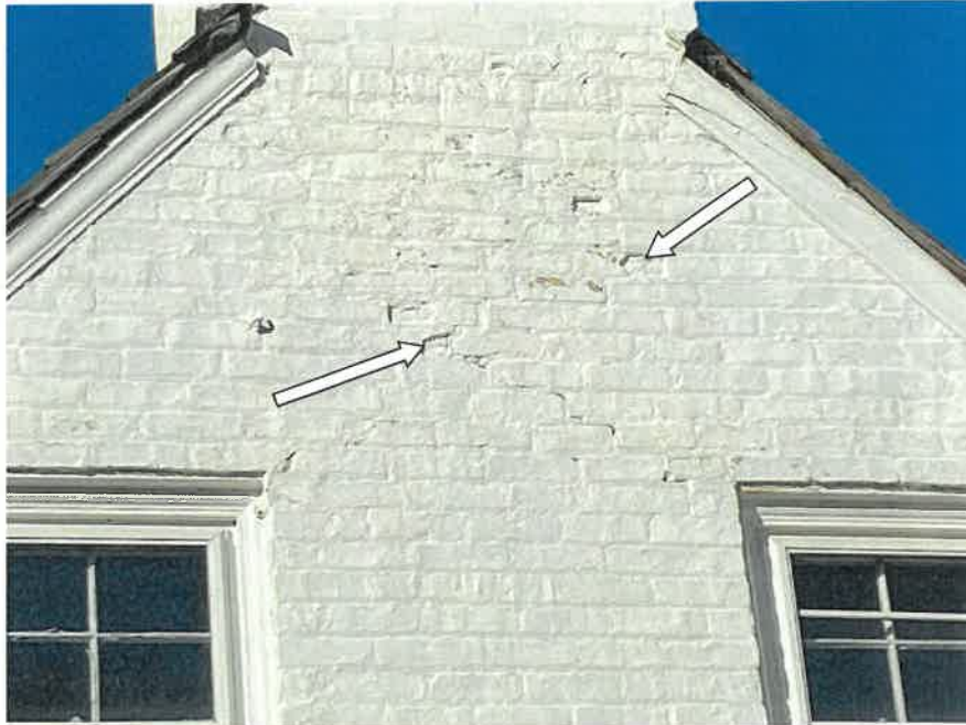
Photo One – Deteriorated masonry on the veneer of the detached garage.
