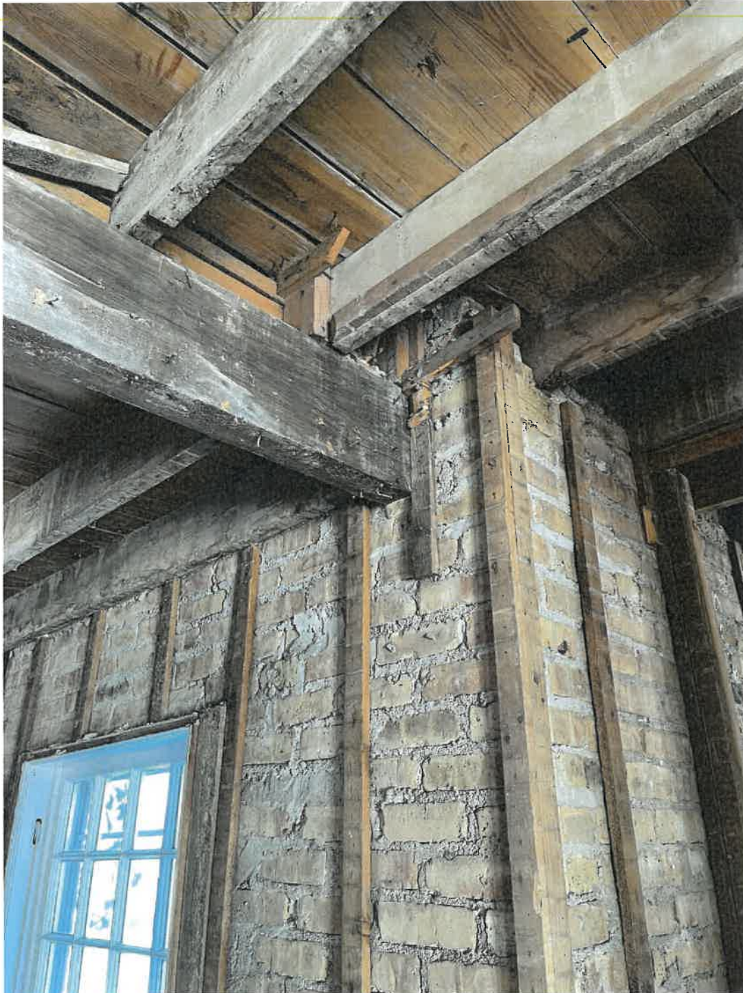
Photo 13A: North Wing (First Floor) – Wood framing at east wall. South end of timber beam pocketed into 3-wythe brick masonry bearing wall with evidence of water damage and possible mold.
