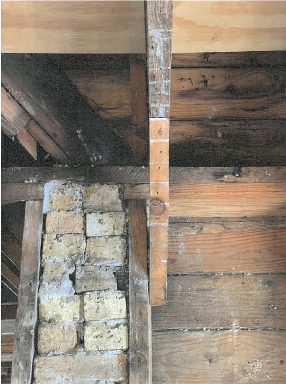
Photo 5: South Wing (Second Floor) – Intersection of Central (2-wythe brick masonry) Wing with South (wood framed) Wing at roof valley. Indeterminate bearing point for valley framing, evidence of charred valley rafter from prior fire, efflorescence at brick wall and evidence of moisture damage at wood framing members
