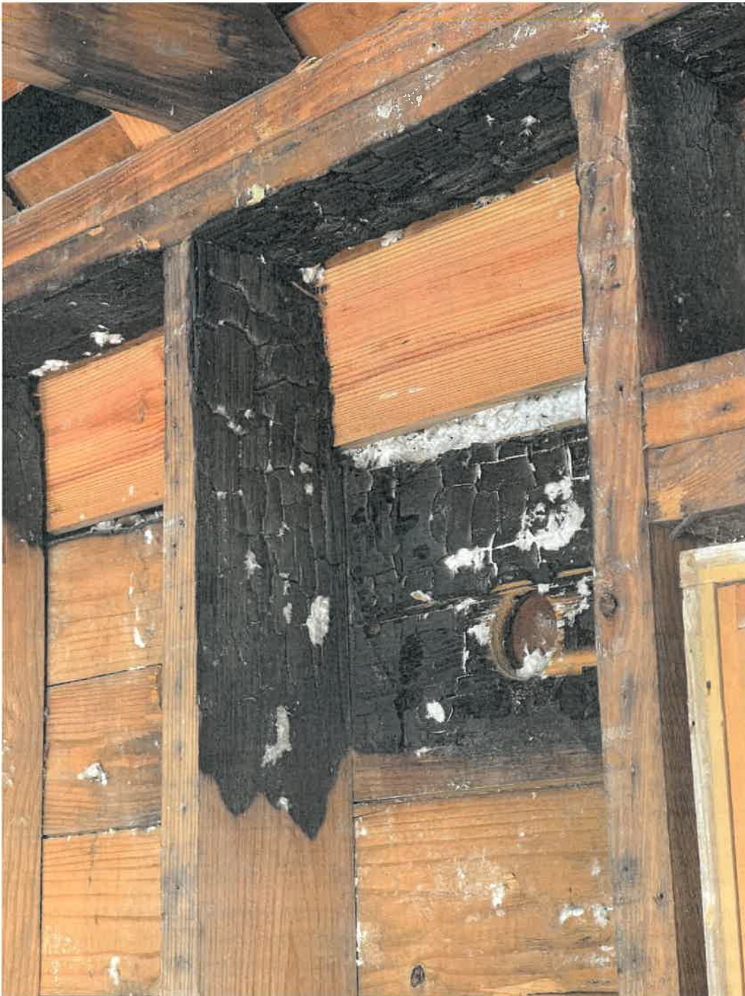
Photo 16: North Wing (Second Floor) –Wood framing at east wall. Charred remains indicate evidence of prior fire
