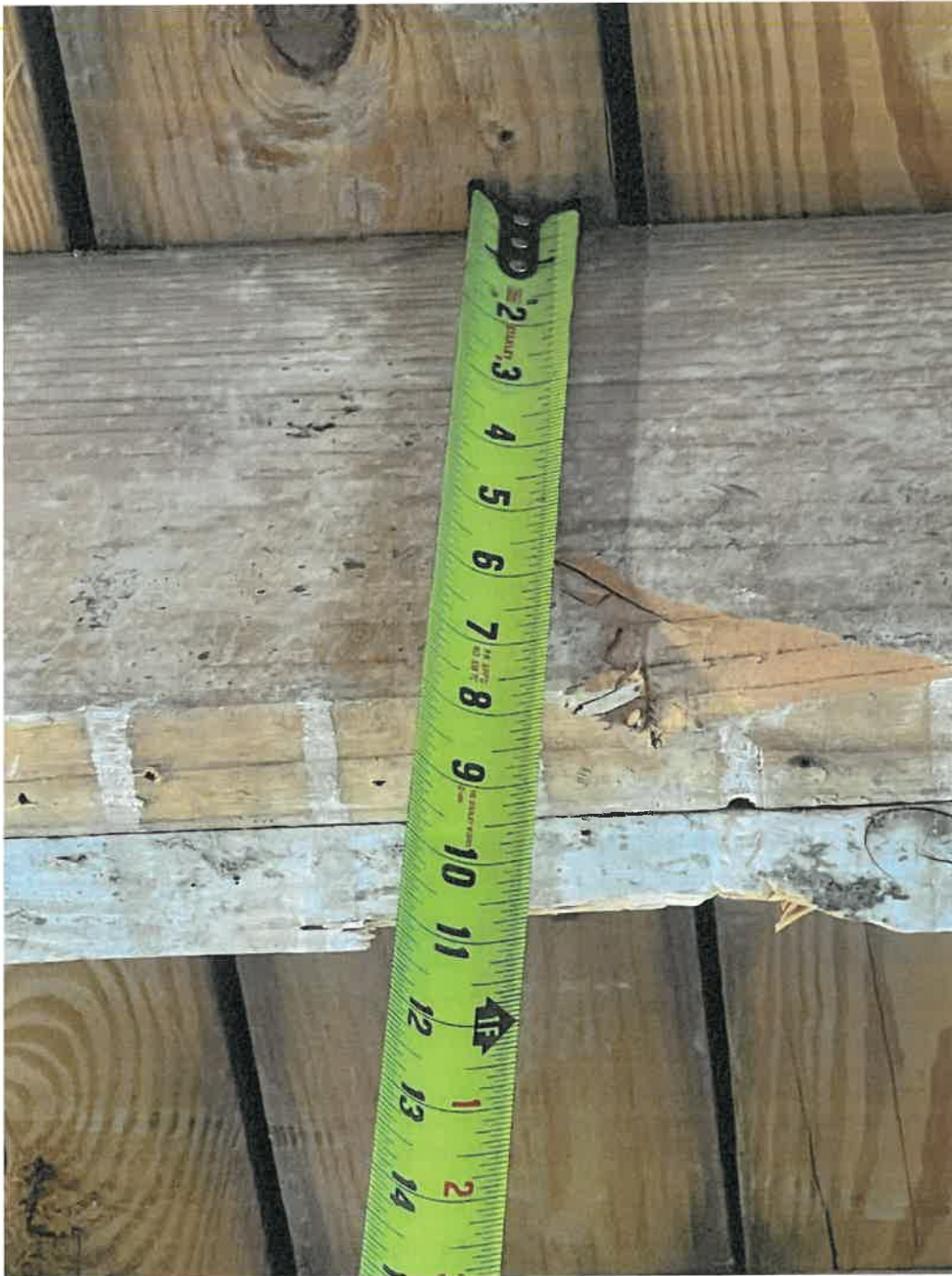
Photo 24A: North/East Wing (First Floor) – Second floor wood floor framing appears undersized (2x8 depth). Floor system is bouncy and significantly not level with 3" +/- dip in floor. Structural reinforcement of floor framing required.
