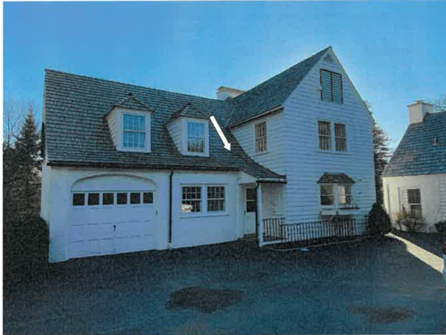
Photo Five – A sag in the roof plane above the garage is evidence of similar sagging in the second-floor joists within.
