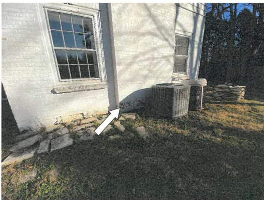
Photo Three – Deteriorated masonry at the base on a chimney on the main house.
