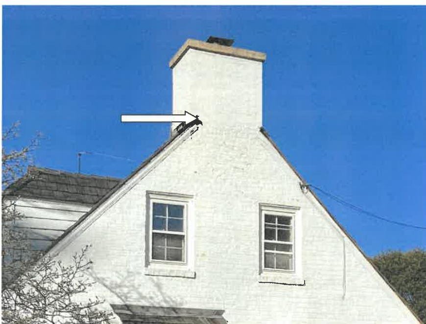
Photo Four – The upper portion of this chimney had been replaced. Additional deterioration appears to be present in the brick below the repaired section of masonry.
