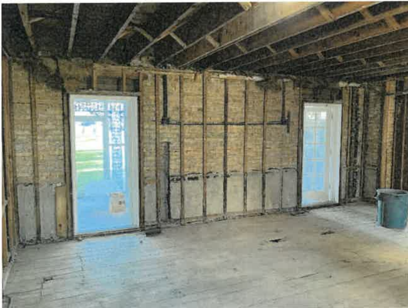
Photo 7: Central Wing (First Floor) – second floor wood joists fixed solid with masonry bearing on 3-wythe brick masonry wall.
