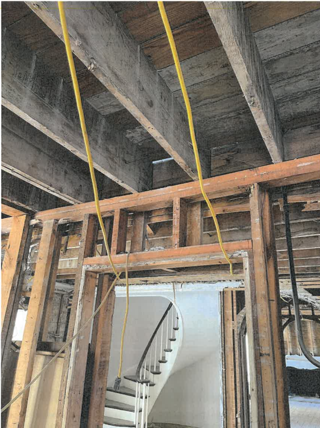
Photo 3: South Wing (First Floor) – Interior bearing wall with no structural header at door opening
