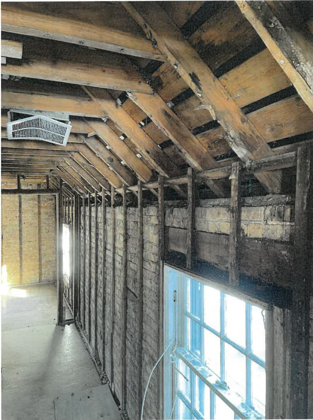
Photo 19: East Wing (Second Floor) – Roof framing undersized for spans. Evidence of moisture damage and possible mold at intersection of roof framing, wood plate and masonry.
