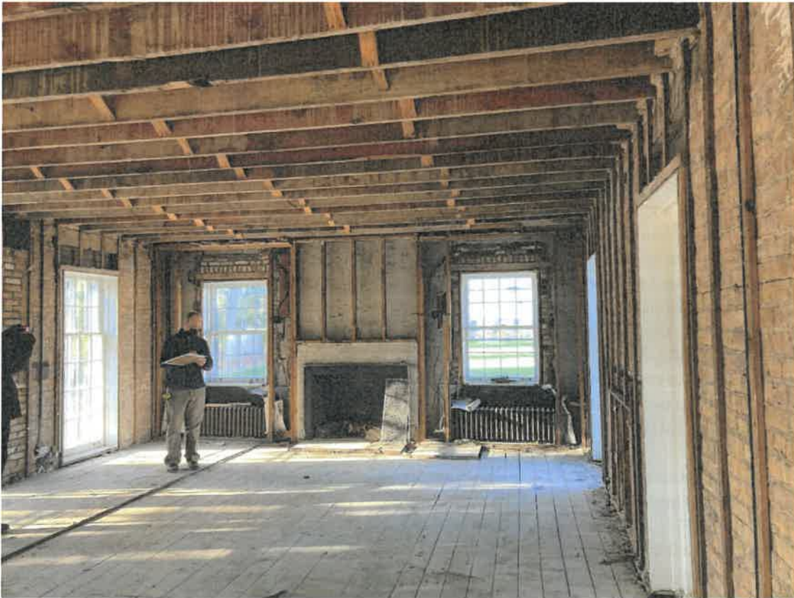
Photo 20: South Wing (First Floor) – Floor framing at both first and second floors bouncy with too much deflection. Structural reinforcement of floor and ceiling framing required. The environmental report indicated that there was an extremely high concentration of mold in the south wing crawlspace.
