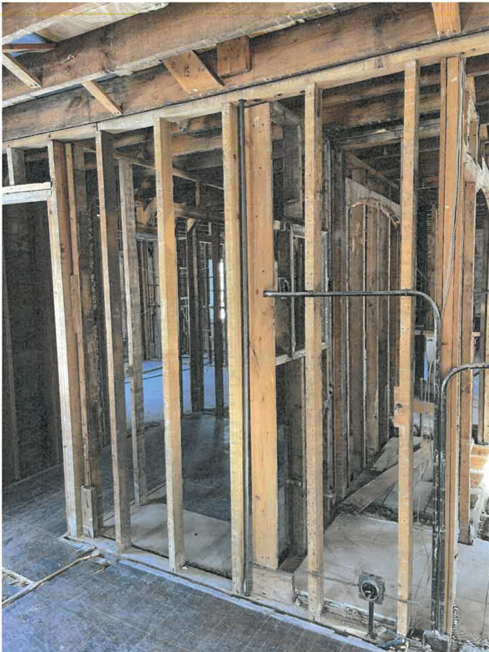
Photo 22: South Wing (Second Floor) – 1 of 2 tie rods through wall framing connected through to roof framing with carpenter built timber truss/beam at ceiling framing. Tie rods and truss/beam do not have any apparent structural purpose and probably distribute roof loads to undersized ceiling and floor framing members, contributing to structural failures and bouncy floors. Structural reinforcement of floor, ceiling and roof framing required.
