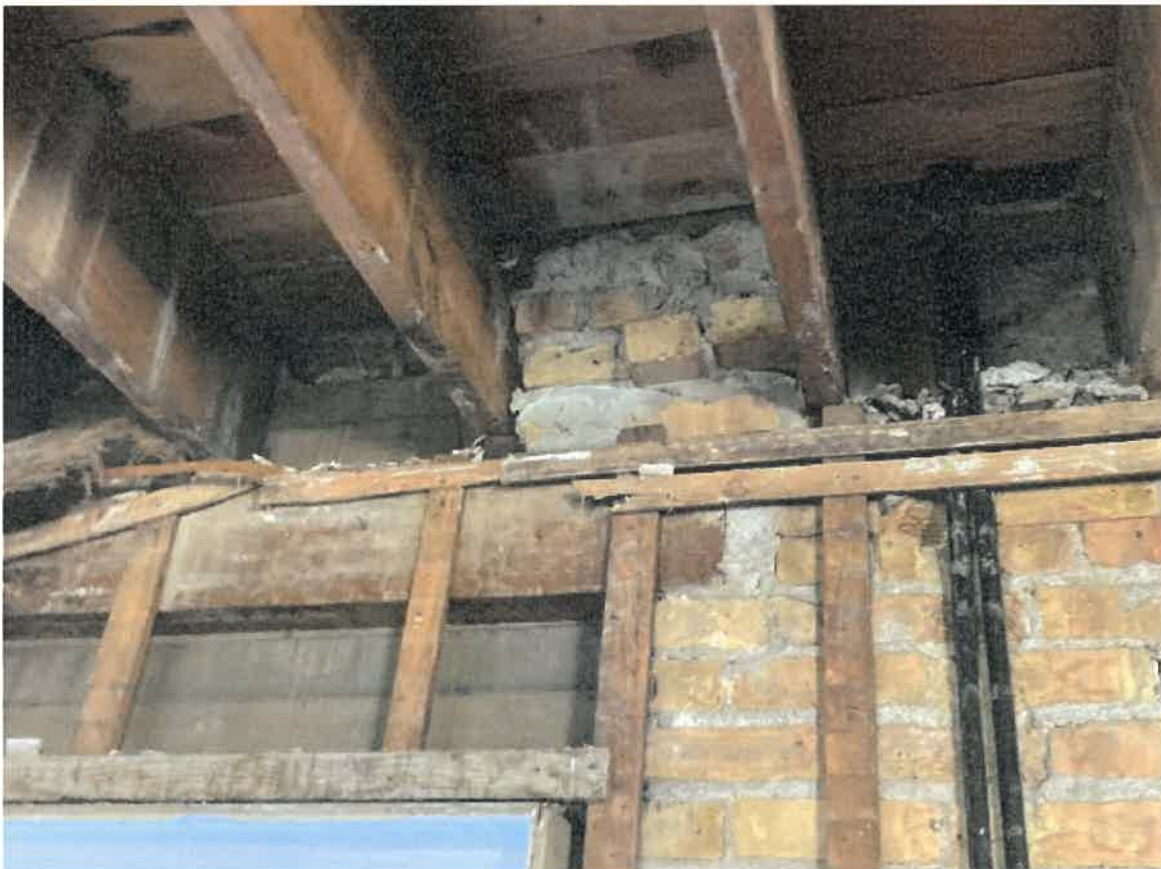
Photo 1: South Wing (First Floor) – Timber window header & second floor wood joists pocketed into 3-wythe brick masonry bearing wall.
