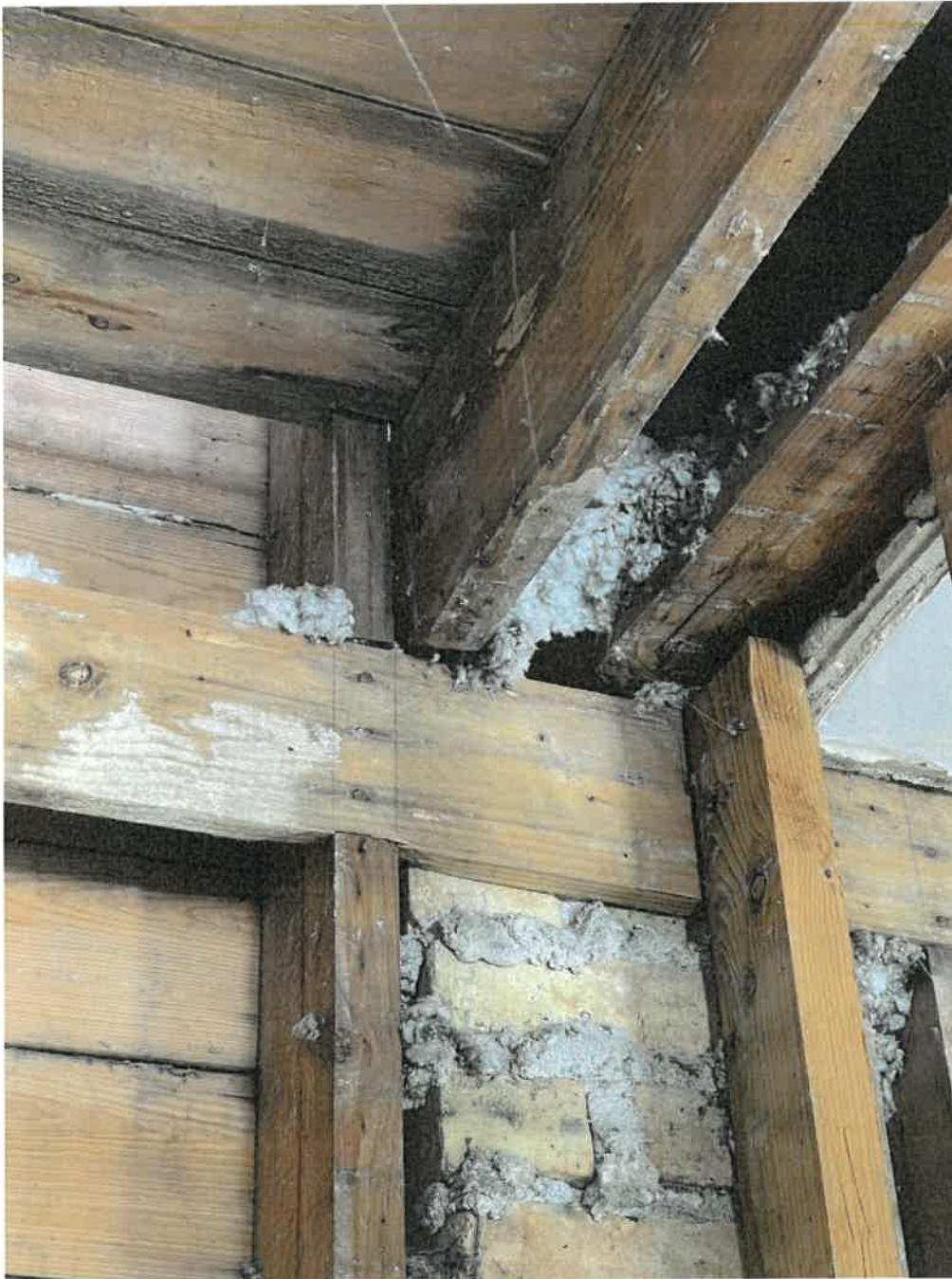
Photo 12: North Wing (First Floor) – Intersection balloon framing at east wall & brick masonry bearing wall, with floor joists pocketed into masonry. Staining of floor boards and framing members may indicate impregnated mold condition. Air gaps at intersection of wood framing and irregular masonry surfaces pose constructability problems for air sealing building envelope.
