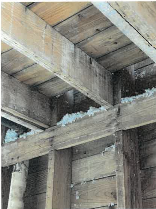
Photo 10A: North Wing (First Floor) – Balloon framing detail at west wall, no fire blocking between first and second floors. Staining of floor boards and framing members may indicate impregnated mold condition.
