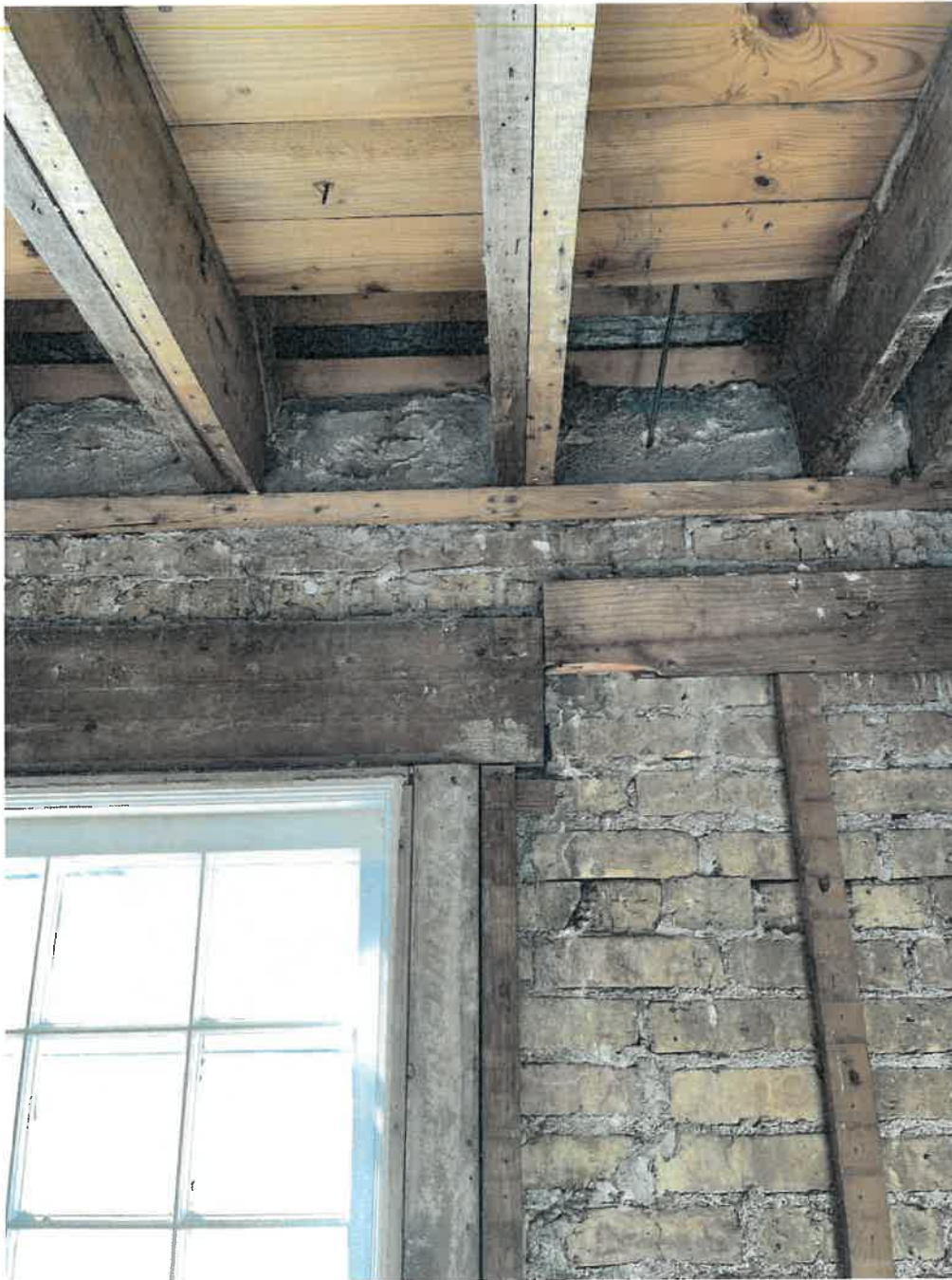
Photo 8: Central Wing (Second Floor) – Timber header showing evidence of moisture damage from masonry above. Masonry failure in various locations. Second floor ceiling joists are solidly set in masonry wall and show moisture damage and possible mold growth.
