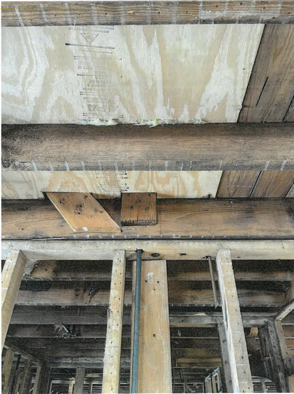
Photo 22A: South Wing (Second Floor) – Detail of 1 of 2 tie rods through wall framing connected through to roof framing with carpenter built timber truss/beam at ceiling framing with 1x4 vertical and diagonal members connecting to roof framing. Structural reinforcement of floor, ceiling and roof framing required.
