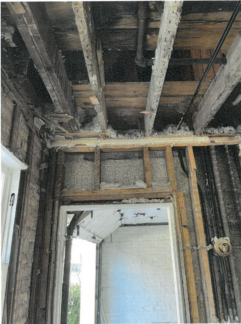
Photo 17: East Wing Garage (First Floor) – Wood floor/ceiling joists bouncy & not level. Wood framed bearing wall lacking header at door opening. Plumbing lines cut into floor framing members and second floor sheathing. Evidence of water damage and possible mold. Garage wall painted on both exterior and interior faces, not allowing masonry wall to breathe. Condition of masonry, under paint, unknown.
