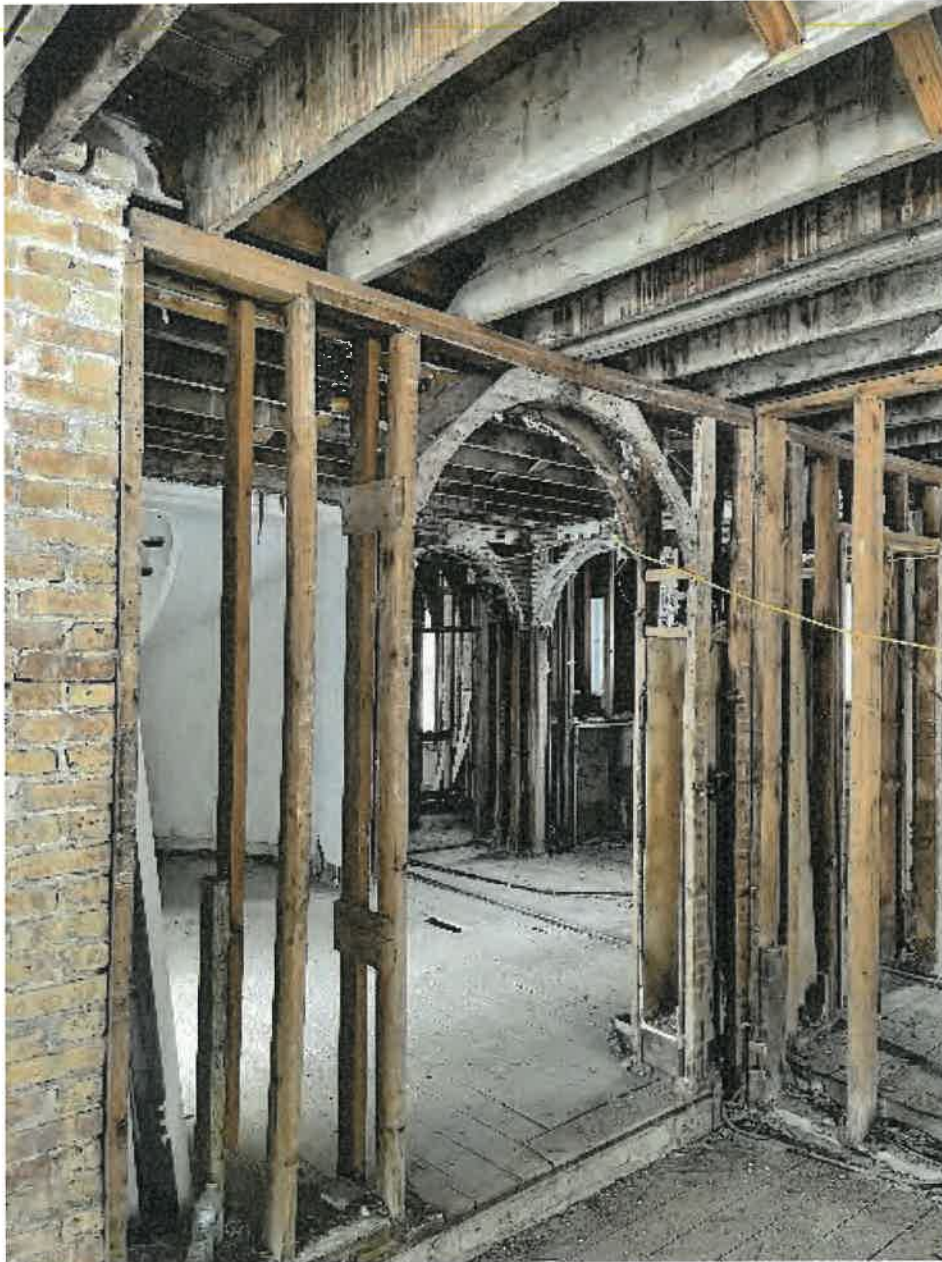
Photo 23: South Wing (First Floor) – Floor framing second floor bouncy with too much deflection. Wood framed bearing wall lacking header at door opening and joist ends. Structural reinforcement required. Efflorescence at brick wall and evidence of moisture damage at wood framing members bearing on masonry. In the upper left corner of the photo, the wood framing member that is typically pocketed into the masonry is exposed and illustrates the concern about susceptibility of wood decay where wood framing is pocketed into masonry.
