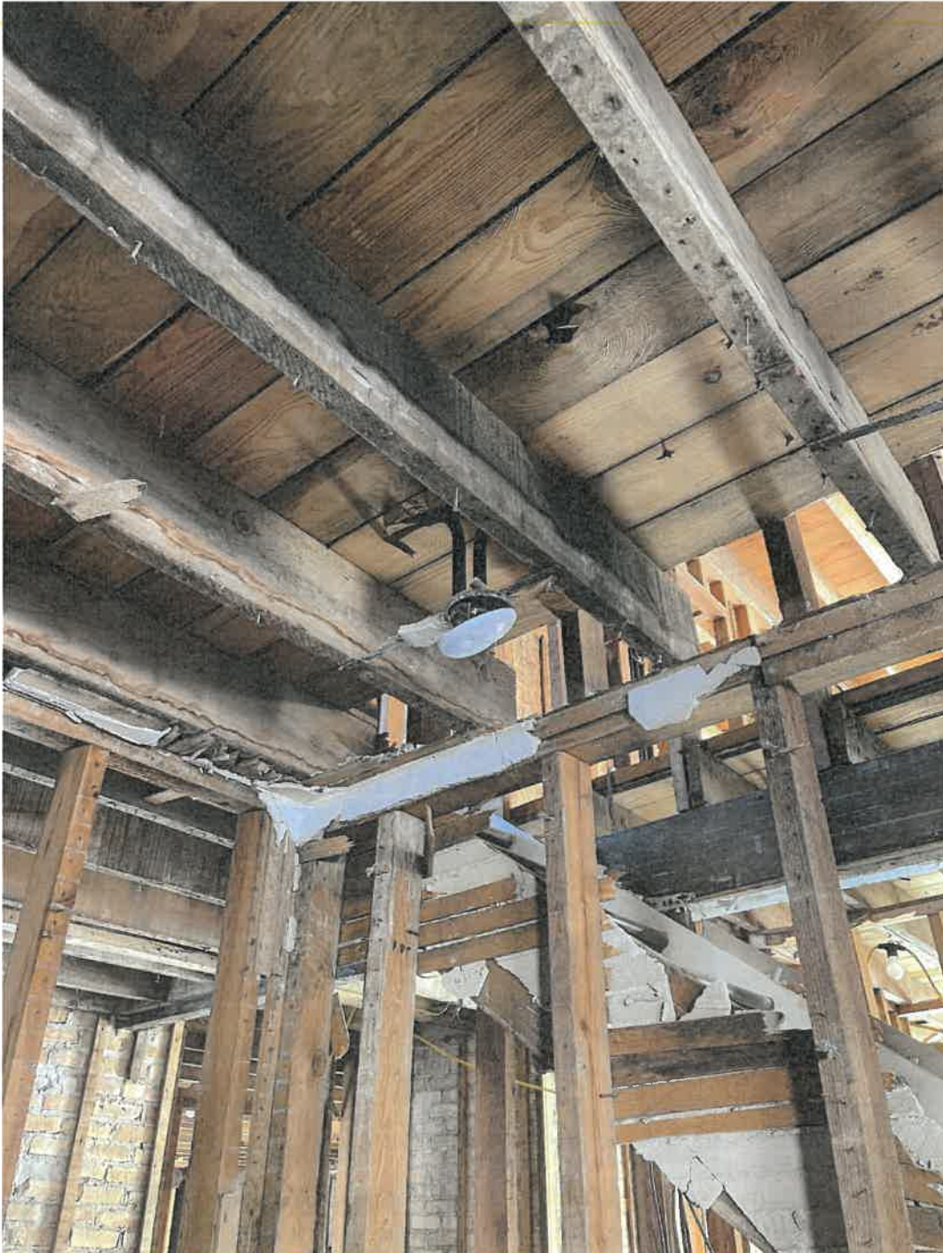
Photo 18: North & East Wing (First Floor) – Wood floor/ceiling joists bouncy & not level. Wood framing members stained indicating moisture damage and possible mold. Timber beam vertically unsupported.
