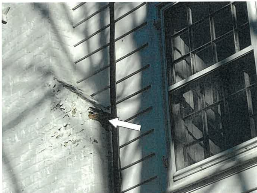
Photo Two – Deteriorated masonry on a chimney on the main house.
