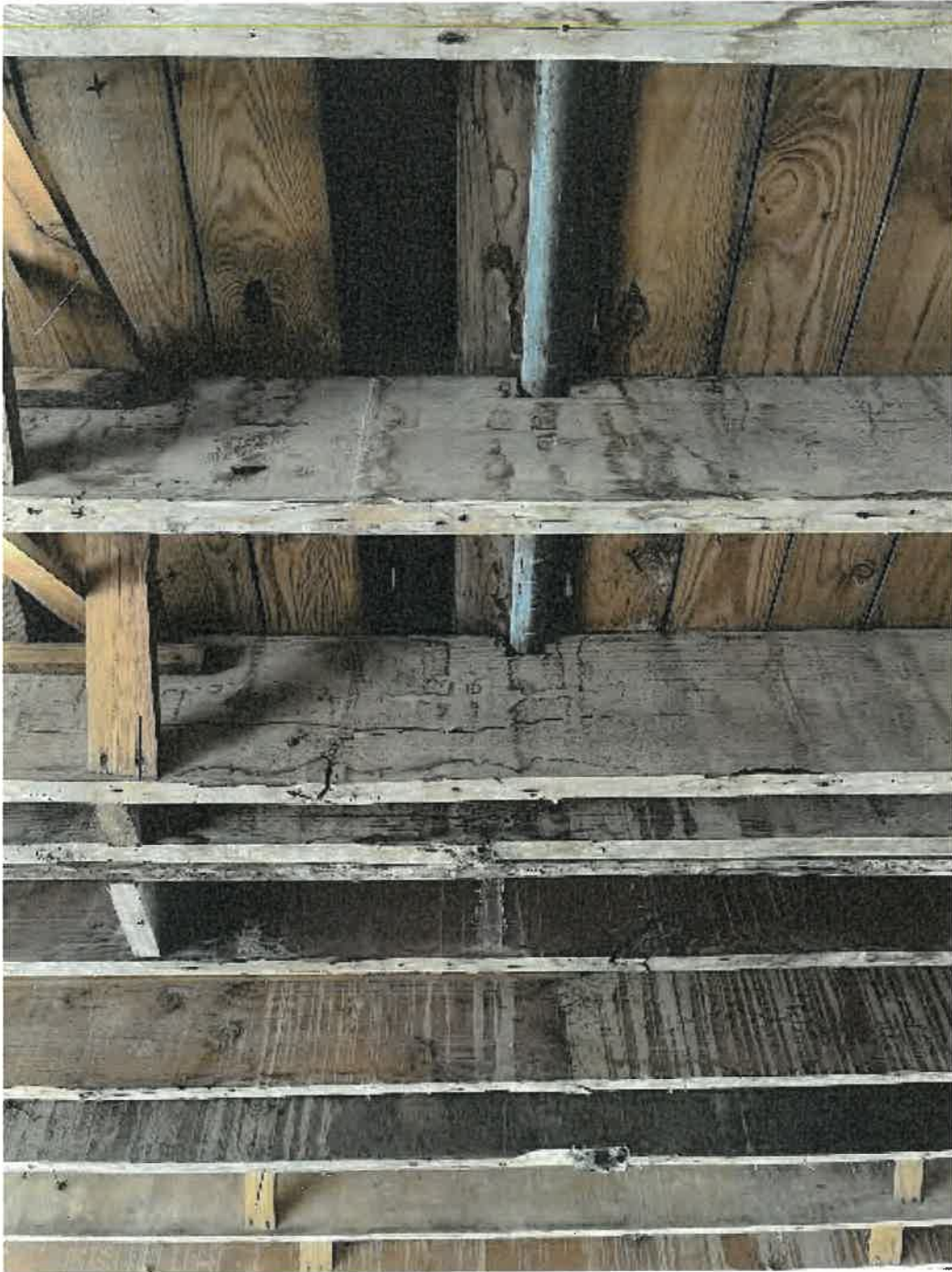
Photo 2: South Wing (First Floor) - Second floor joists discolored and stained showing possible evidence of moisture damage. Floor framing bouncy at both first and second floors. Note structural failures of some joists.
