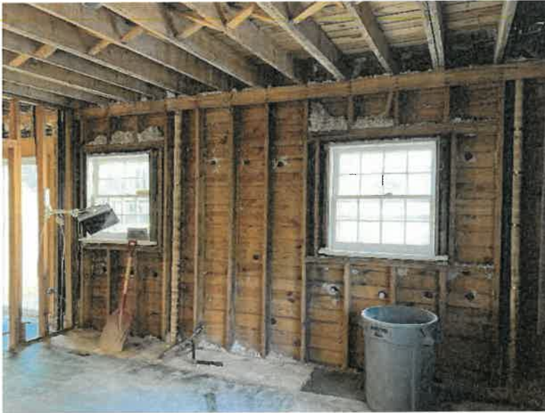
Photo 10: North Wing (First Floor) – Balloon framing at west wall.
