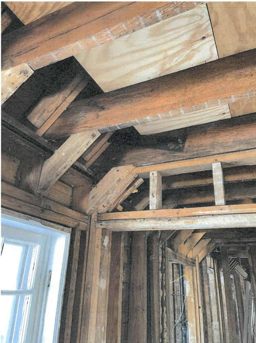
Photo 22B: South Wing (Second Floor) – Black strap end connection detail that appears part carpenter built timber truss/beam at wall and ceiling framing. Roof framing not totally connected to wall plates. Water damage evident and possible mold. Structural reinforcement of floor, ceiling and roof framing required.
