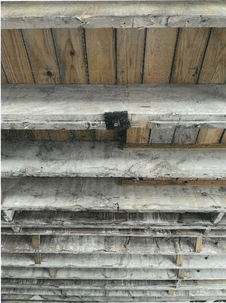
Photo 21: South Wing (First Floor) – 1of 2 tie rod connectors at ceiling framing connected through second floor to roof framing. Floor/ceiling joists bouncy. Evidence of structural failure in some of the framing members. Joists stained by possible moisture damage. Structural reinforcement of floor, ceiling and roof required.
