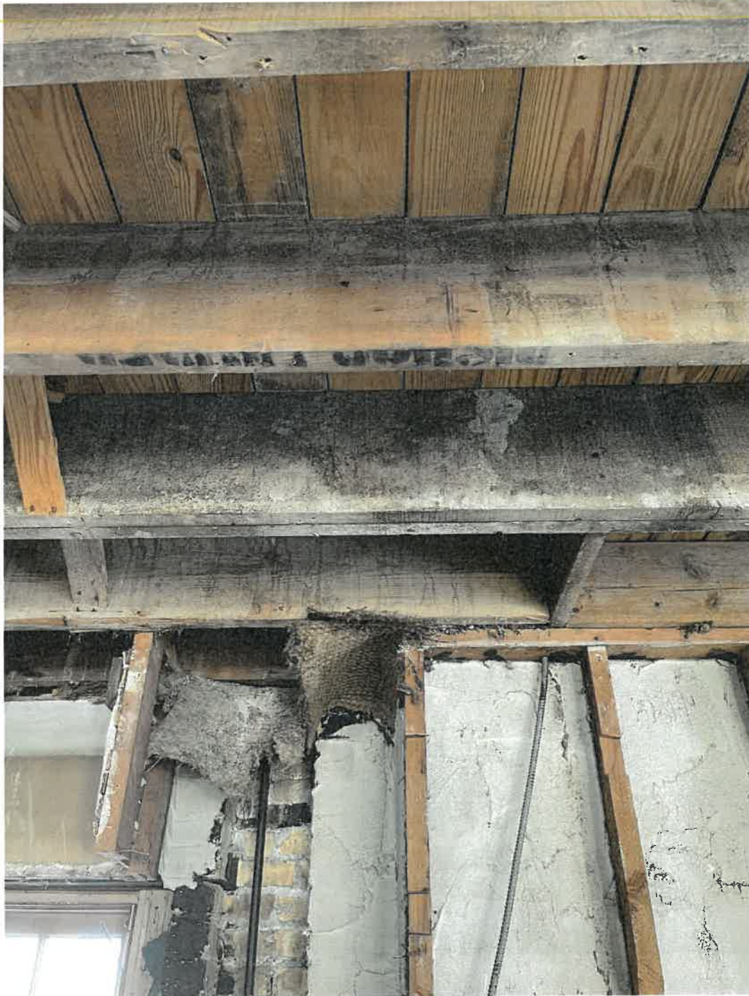
Photo 4: South Wing (First Floor) – Second floor wood joists and floor boards showing stain from moisture and possible mold
