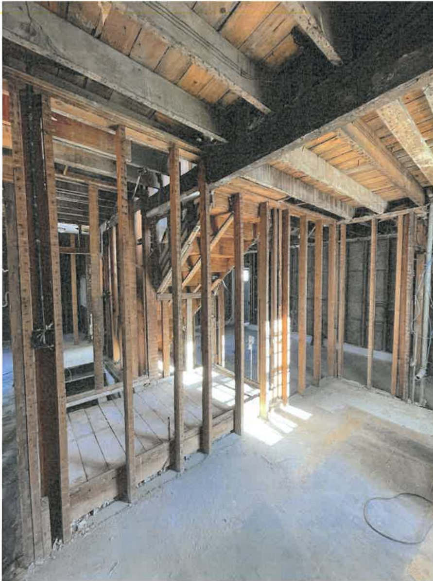
Photo 24: North/East Wing (First Floor) – Interior wood framing. Second floor framing bouncy and significantly not level with 3" +/- dip in floor. Vertical support of north beam end at stair indeterminate. Structural reinforcement of floor framing required.
