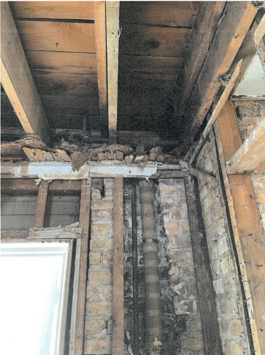
Photo 7A: Central Wing (First Floor) – Detail second floor wood joists & timber window header bearing on 3-wythe brick masonry wall. Efflorescence & water damage at brick wall and corner wood framing. Typical condition at masonry window openings, wood infill between top of window and underside of timber header, with 1-wythe brick masonry jack arch exterior side. Masonry cracking evident from exterior over windows. Masonry chopped out for piping
