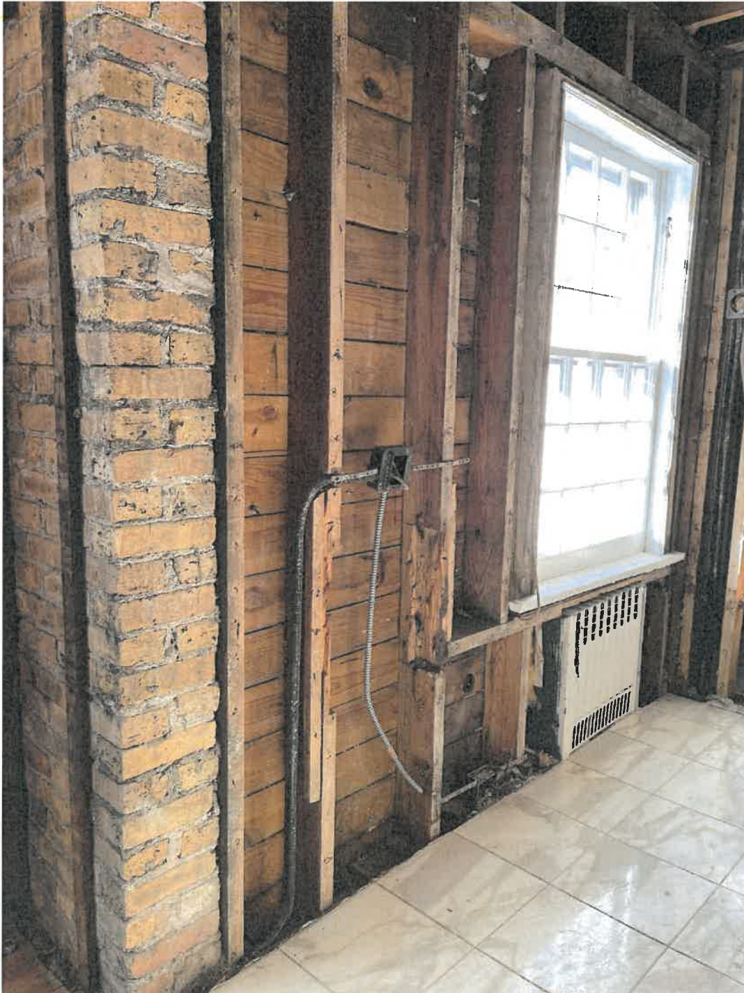
Photo 14: North Wing (Second Floor) – Balloon framing at west wall. Framing hacked out and spliced. No header at window opening. Indication of moisture penetration at masonry.
