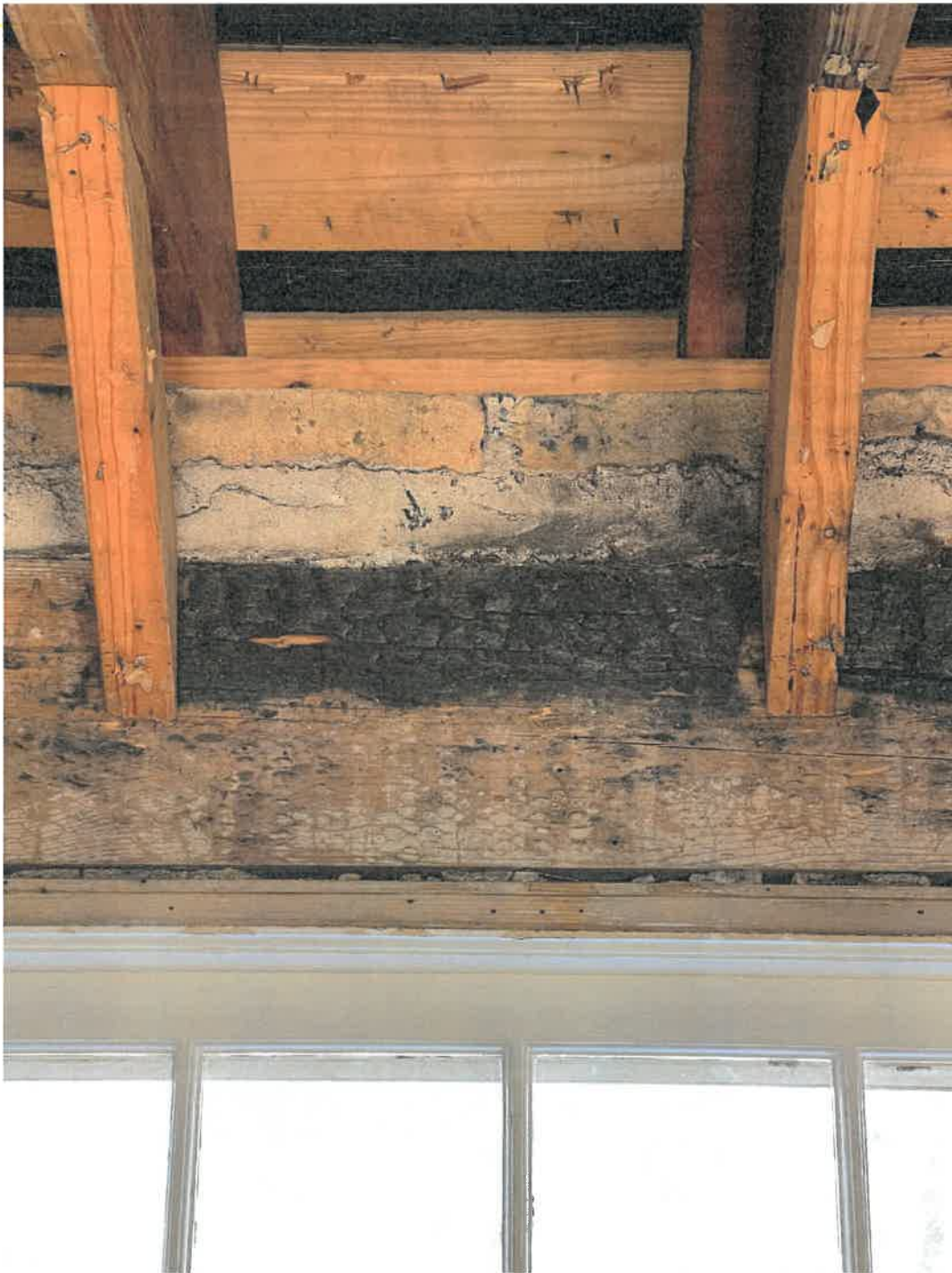
Photo 9: Central Wing (Second Floor) – Charred timber header
