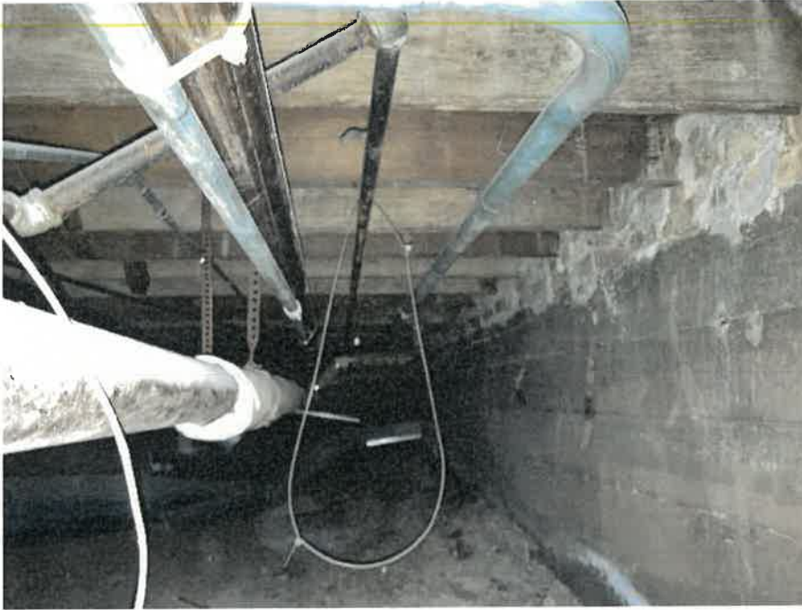
Photo 6: South Wing (Crawlspace) - First floor wood joists pocketed into 3-wythe brick masonry bearing wall at grade and top of foundation, Environmental Reports indicate high presence of mold
