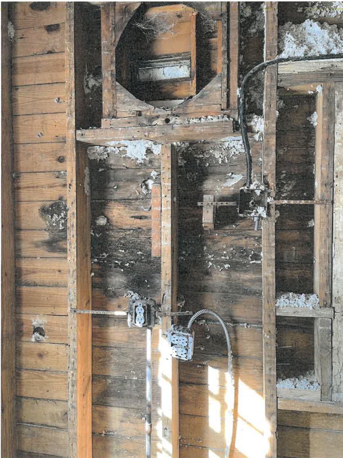
Photo 11: North Wing (First Floor) – Balloon framing at north wall, mold inside face of cladding
