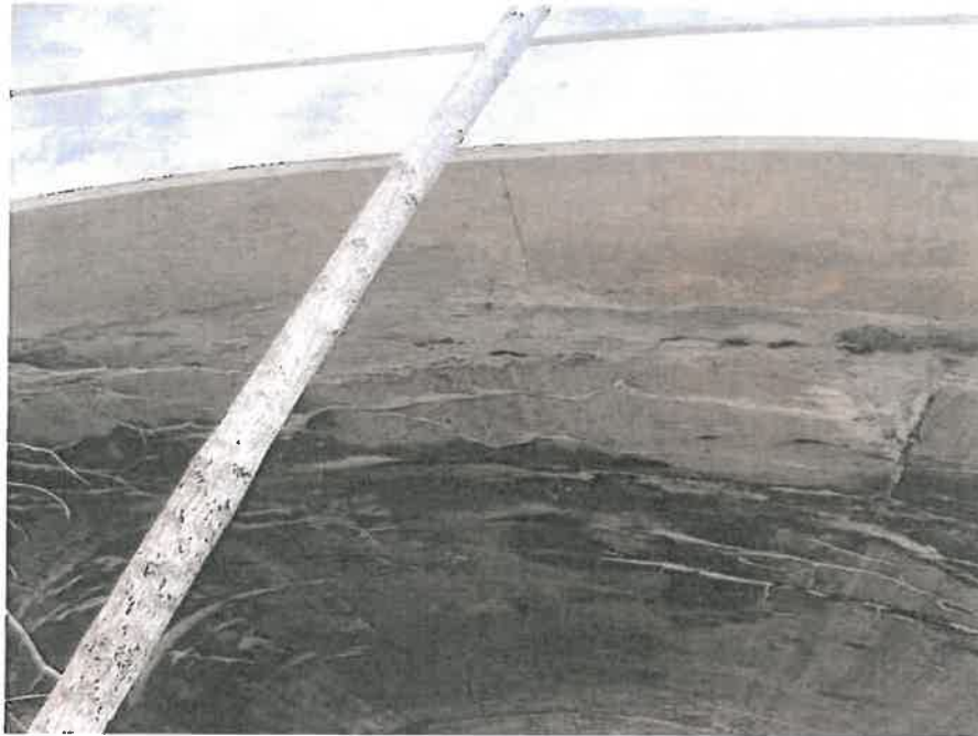
Exhibit 2.G.1 Soffit of north span, east side showing longitudinal cracking
