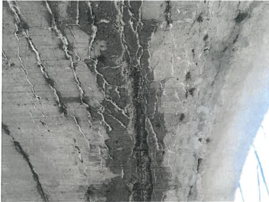
Exhibit 2.G.3 Soffit of north span, west side showing longitudinal cracking & spalls
