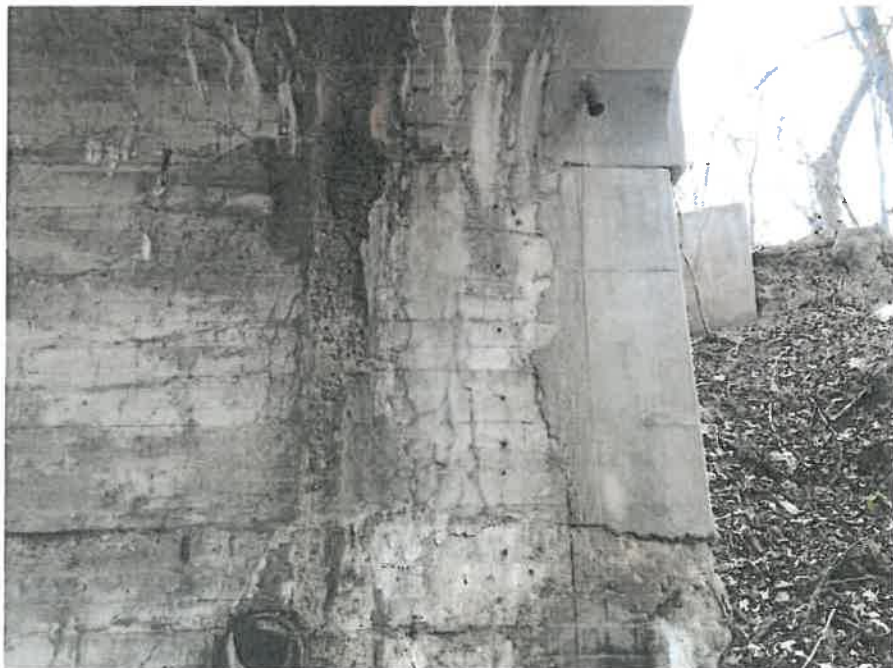
Exhibit 2.F.2 South pier, west side showing spandrel wall repair joint
