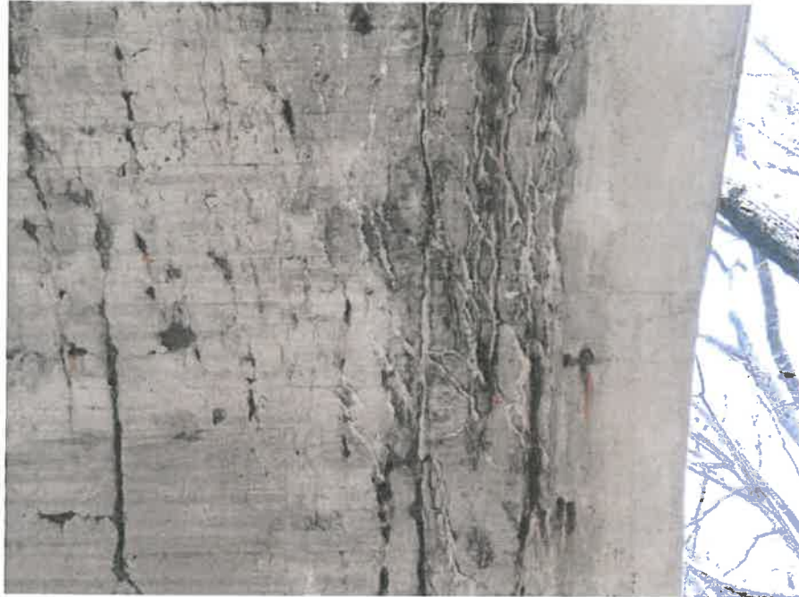
Exhibit 2.G.5 Soffit of center span, west side showing longitudinal cracking
