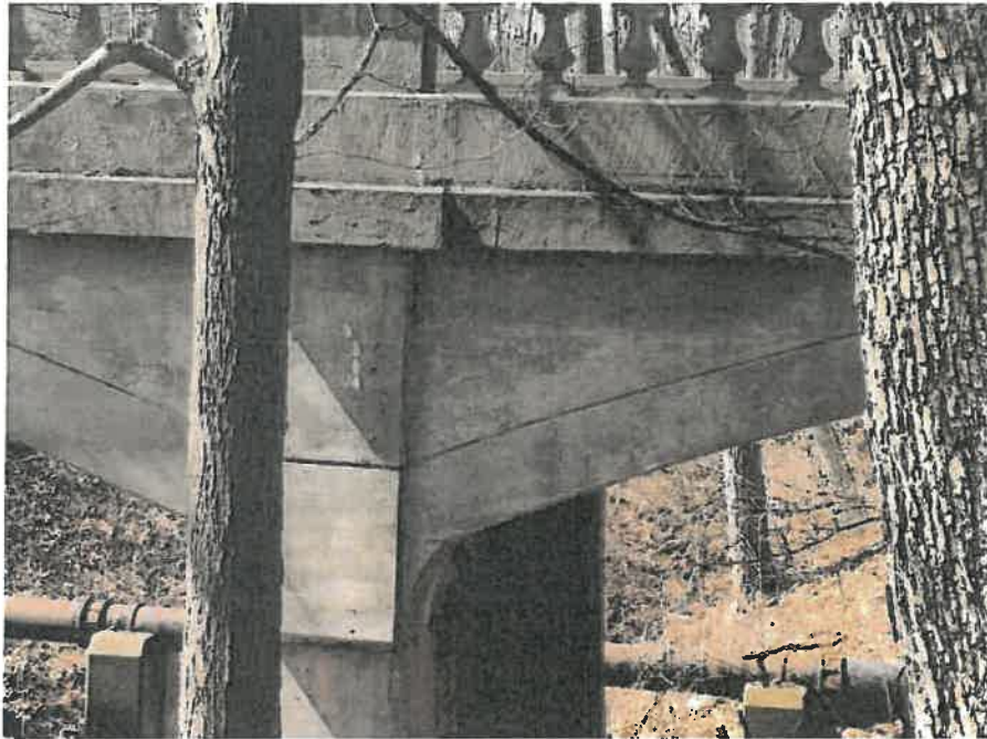
Exhibit 2.F.1 North pier elevation showing spandrel walls
