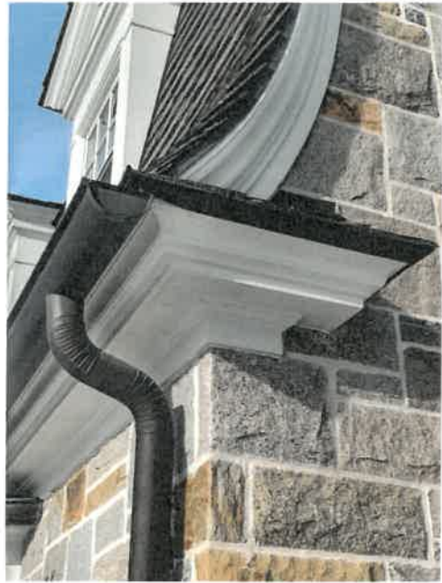
Typical eave and gutter detail
