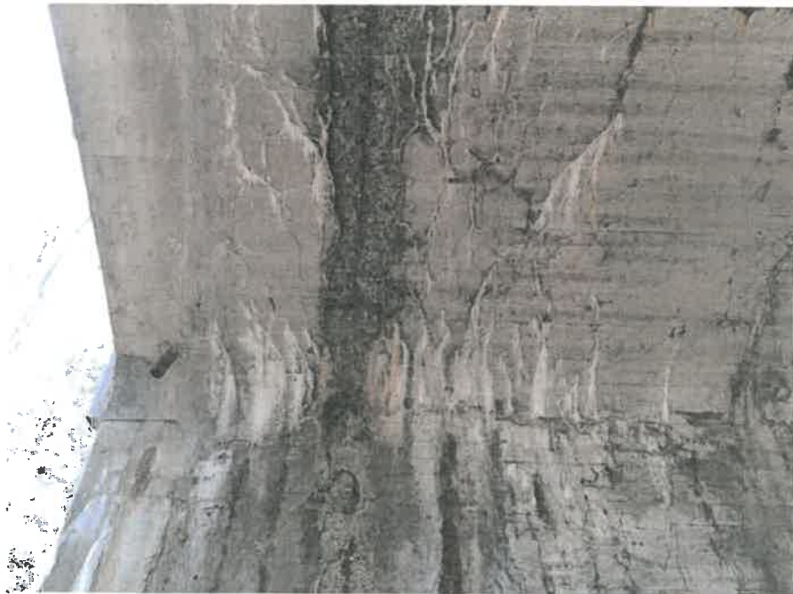
Exhibit 2.G.6 Soffit of center span showing longitudinal cracking & spalls
