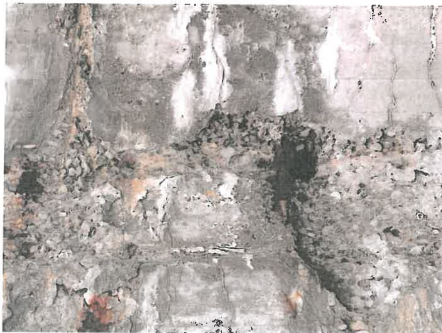
Exhibit 2.H.3 Barrel-to-pier joint at north face of north pier
