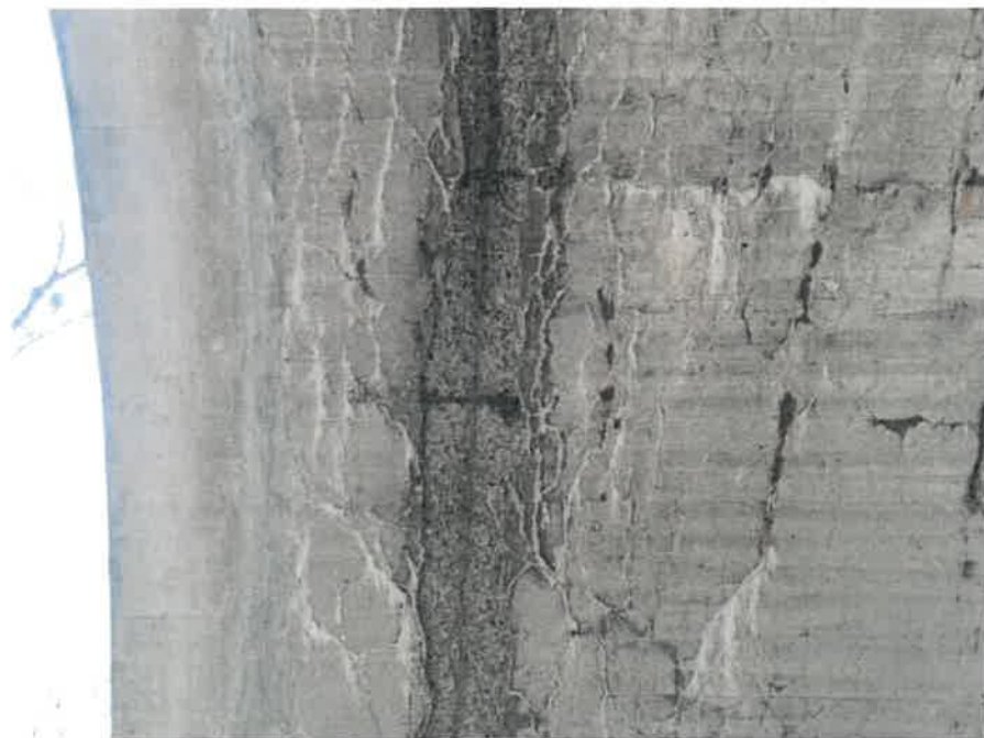
Exhibit 2.G.4 Soffit of center span, east side showing longitudinal cracking & spalls
