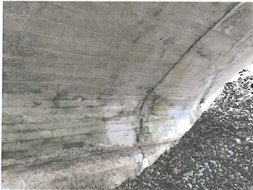
Exhibit 2.G.2 Soffit of north span showing transverse cracking
